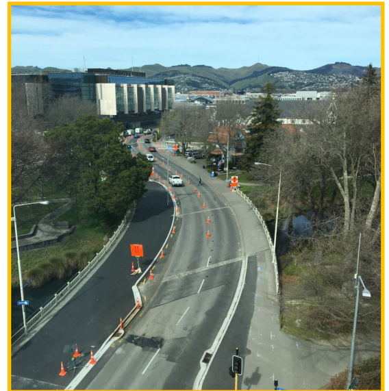
Cashel Street to Lichfield Street: where work is starting first.
