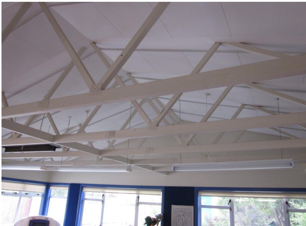
Photograph 4 Exposed timber roof trusses at eastern end of building.
