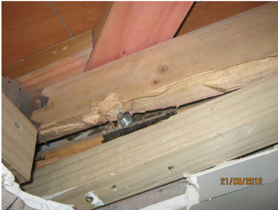
Photo 3: Longitudinally split timber rafter plate to wall on grid ae
