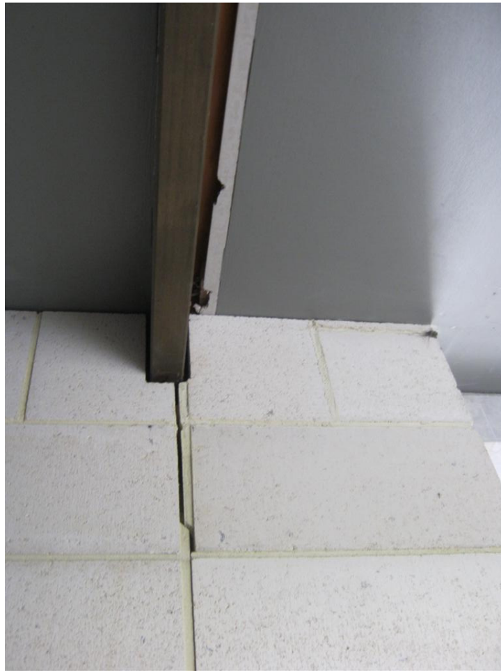
Photo 5: Cracking to the external masonry veneer in the central stair area
