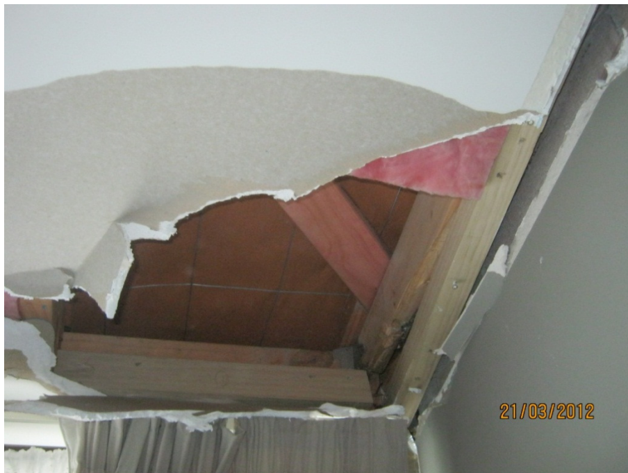
Photo 2: Longitudinally split timber rafter adjacent wall to grid ae
