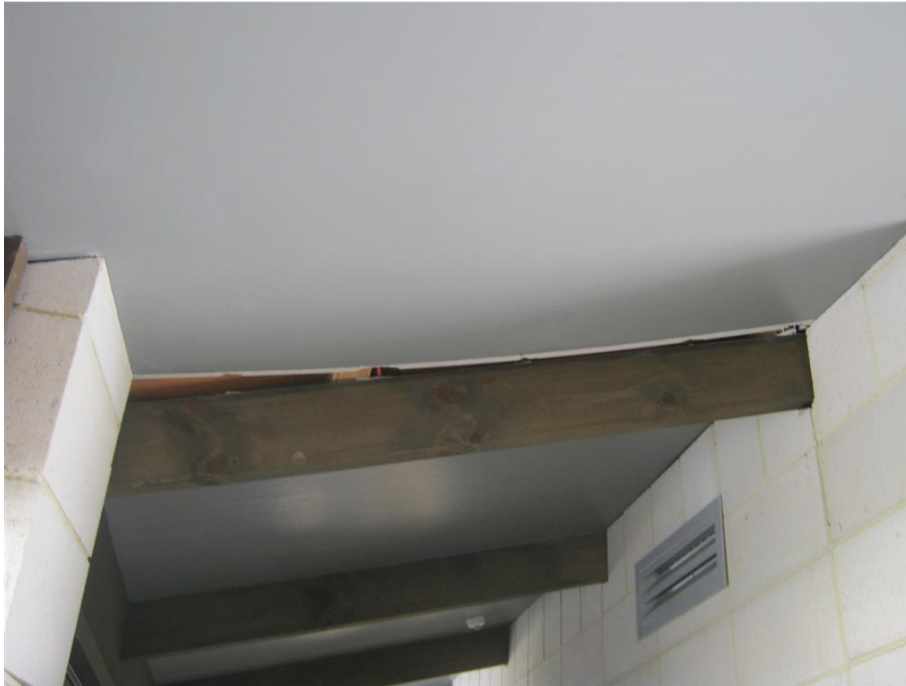
Photo 7: Separation between the timber roof members and the plaster ceiling
