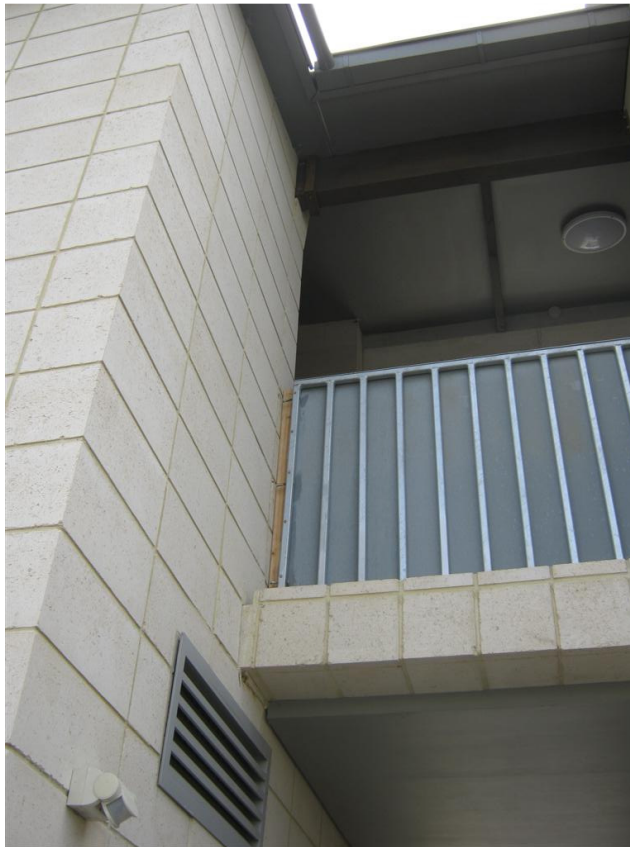
Photo 1: Deformation to masonry veneer in central stair area
