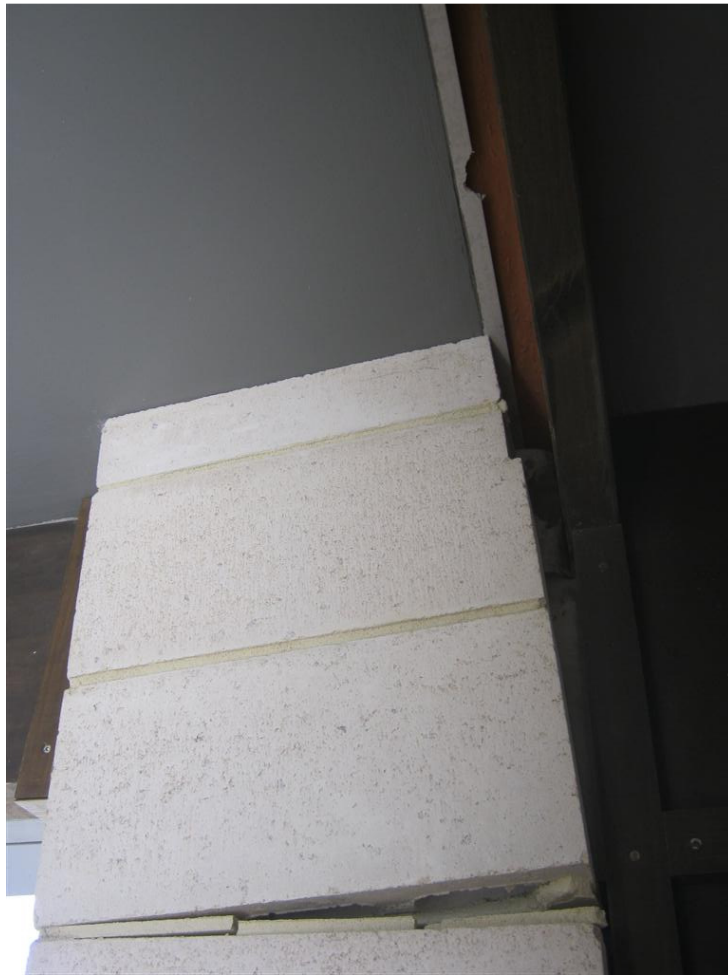
Photo 6: Displaced masonry veneer in the central stair area
