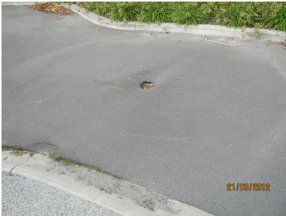
Photo 4: Evidence of liquefaction to external areas
