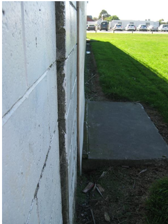
Photo 13: Close-up of gap in construction joint.
