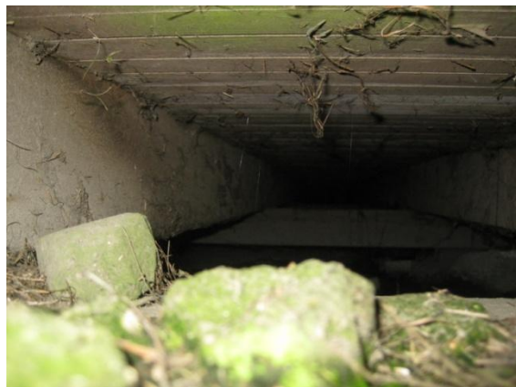
Photo 15: Suspended timber floor seen through vent hole in concrete plinth foundation.
