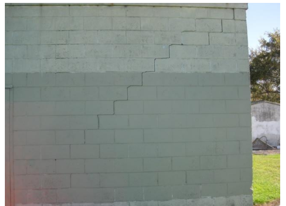
Photo 16: Step cracking along mortar joints.
