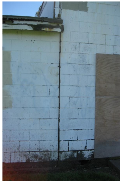
Photo 12: Gap opening up at construction joint between the two sections of the building. View of East wall.
