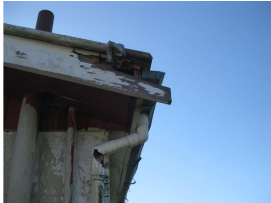
Photo 9: Suspected water damage to roof purlin on South wall.
