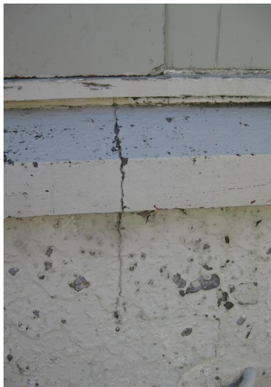
Photo 7: Crack in concrete lintel under window on South wall.
