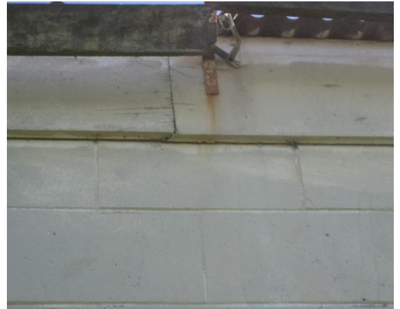
Photo 10: Gap between fascia board at the top of the wall and masonry opening up.
