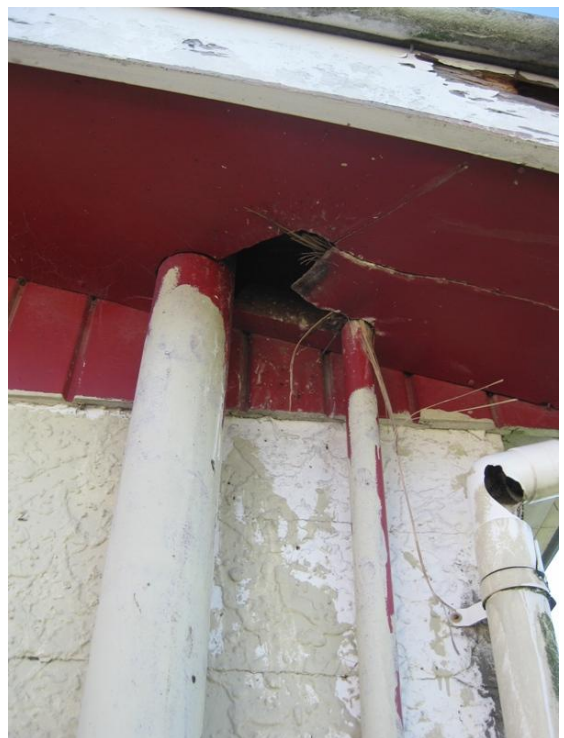
Photo 8: Existing damage to soffit lining and pipes on South side of building.
