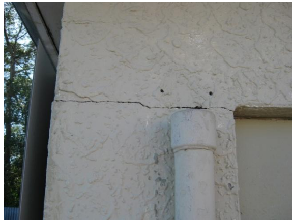
Photo 5: Hairline cracks in stucco cladding around openings on South wall.
