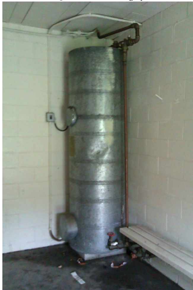
Photo 4: Hot Water Cylinder
