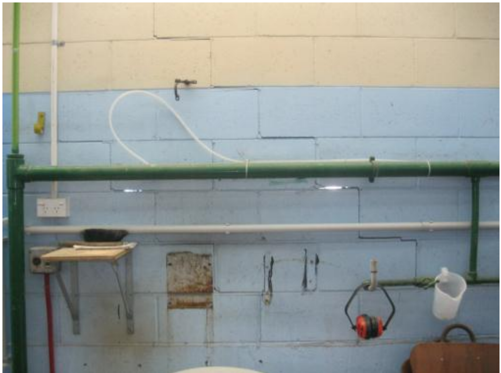
Photograph 10: Shear damage to southeastern external wall.
