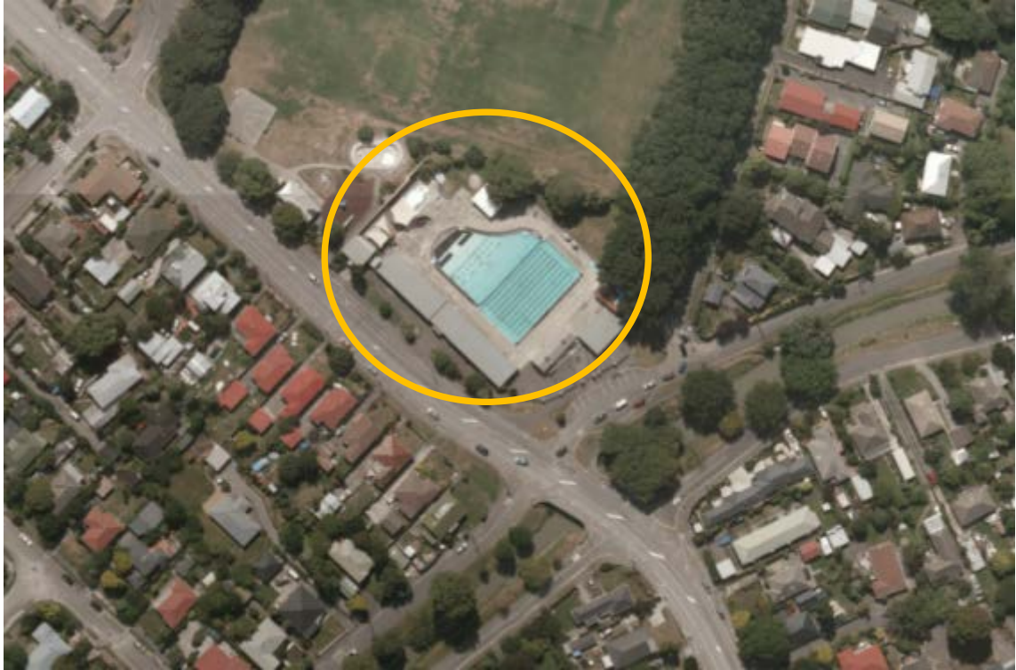
Figure 3 Post February 2011 Earthquake Aerial Photography 3
