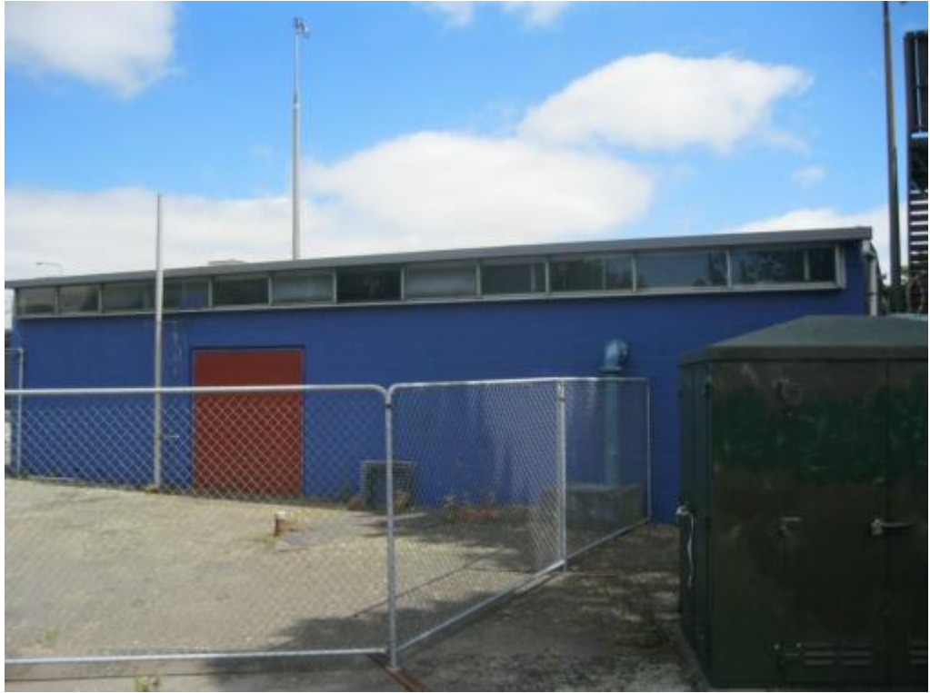
Photograph 9: Southeastern external wall elevation.
