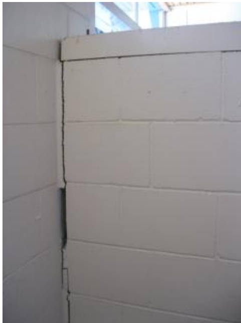
Photograph 2 Typical masonry wall separation.
