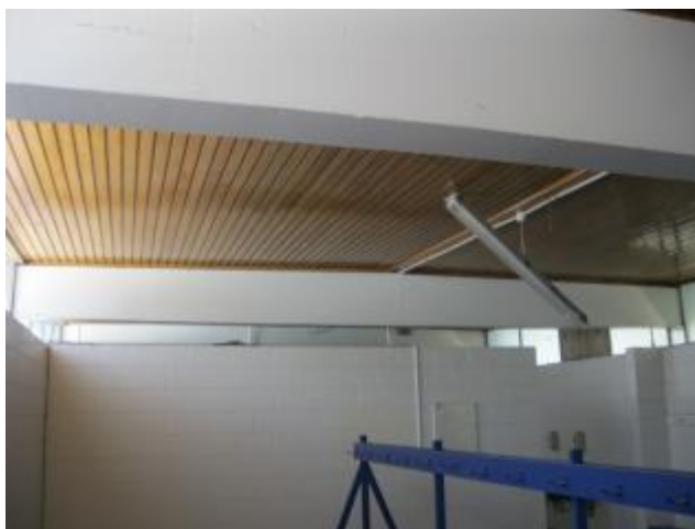
Photograph 2 Typical masonry wall separation.
