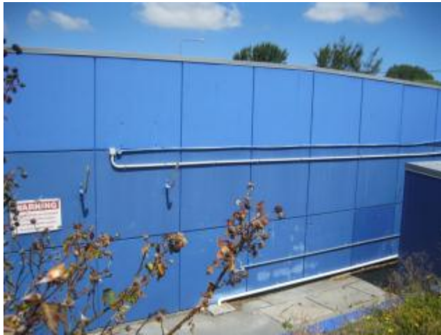
Photograph 8 North-west end precast concrete panel.
