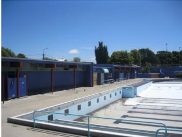
Photograph 1 Pool side elevation of the main complex.
