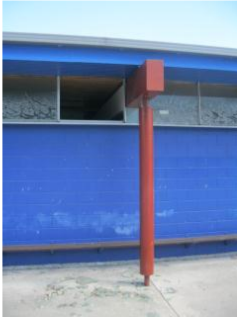
Photograph 4 Typical concrete portal – note the solid steel connectors.
