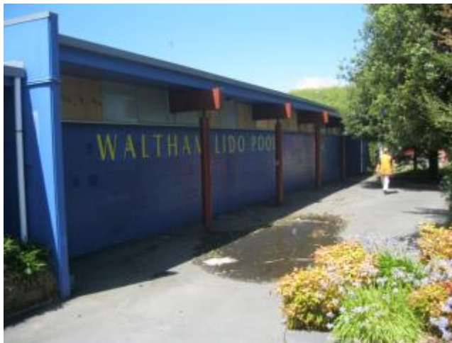
Photograph 5 Roadside south-east side.
