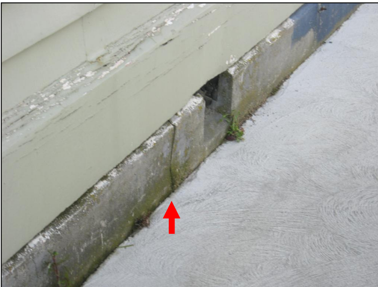
Photo 8: Crack in foundation, north-west side.
