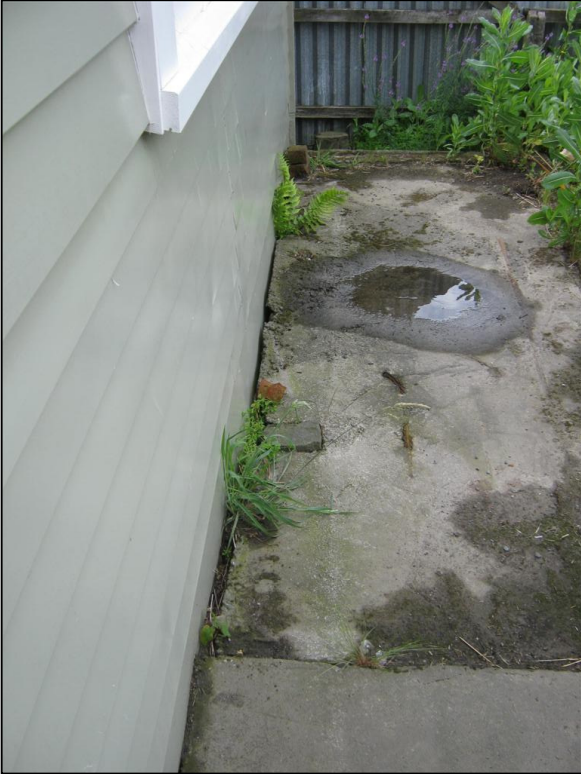
Photo 5: Crack between south-west wall and concrete path (prior earthquake?).
