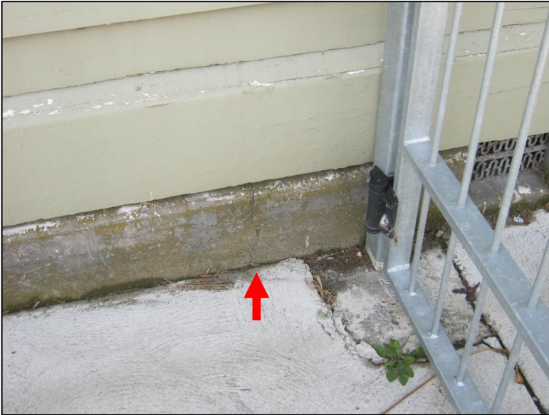
Photo 7: Crack in foundation, north-west side.
