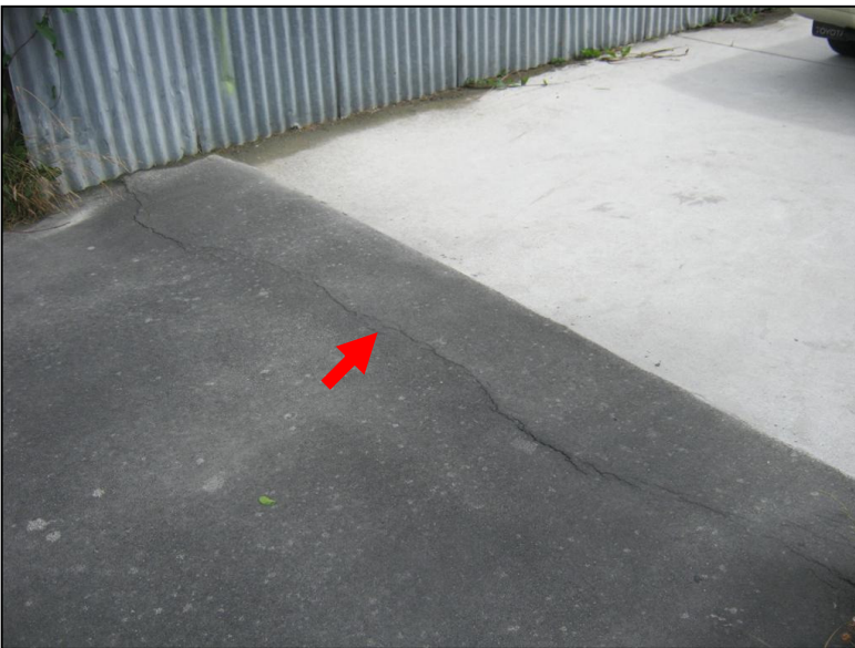
Photo 4: Crack (2mm) in asphalt in driveway resulting in minor heave (10mm).
