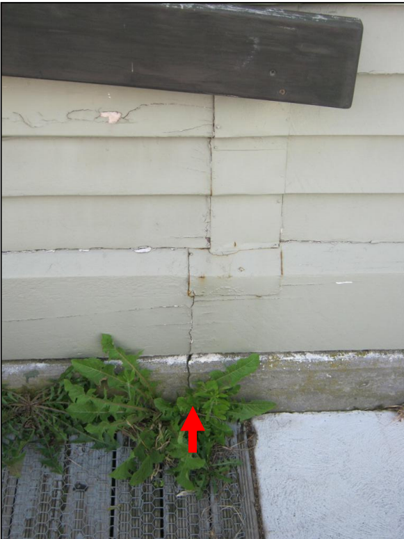
Photo 6: Crack in foundation, north-west side.
