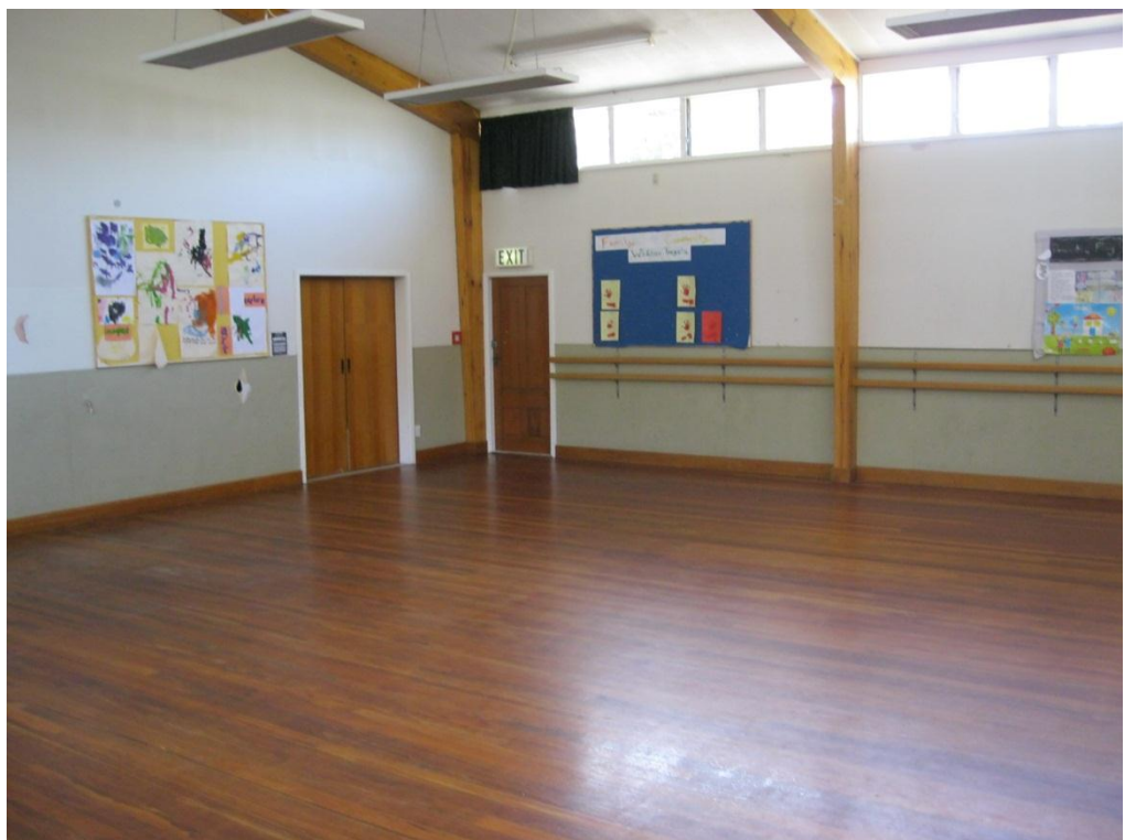
Photograph 6: Suspended timber flooring with internal plasterboard wall linings.
