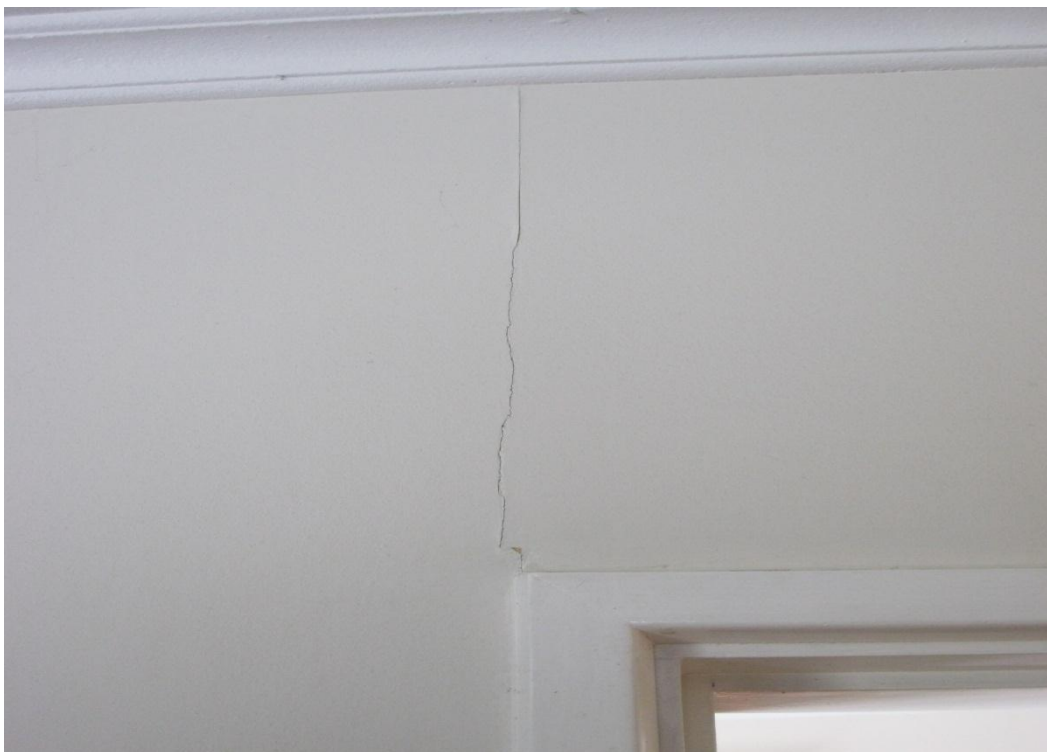
Photograph 7: Minor cracks on timber framed walls at toilet.
