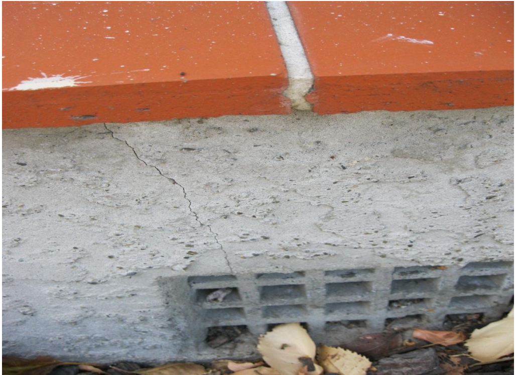
Photograph 9: Slight cracking to the perimeter strip footing.
