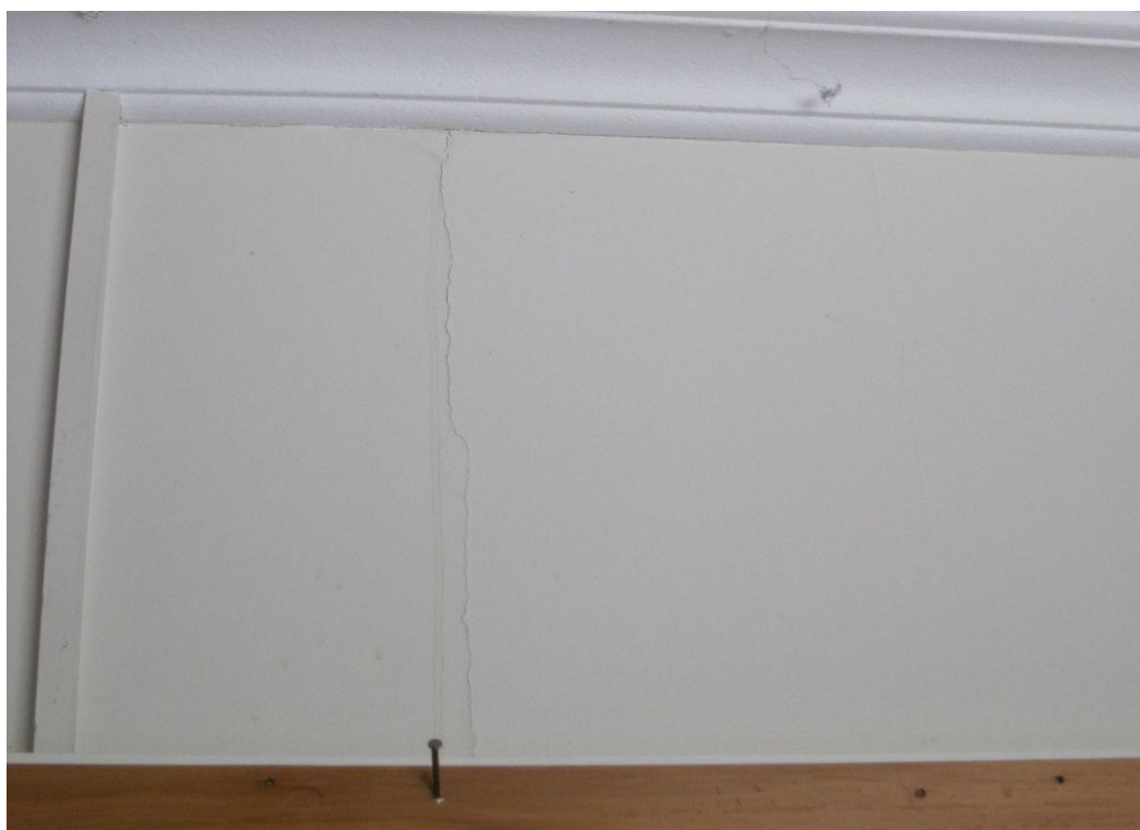
Photograph 8: Minor cracks on timber framed walls at chapel.
