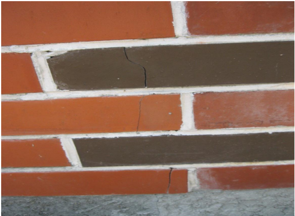
Photograph 10: Minor cracking of the external brick veneer.
