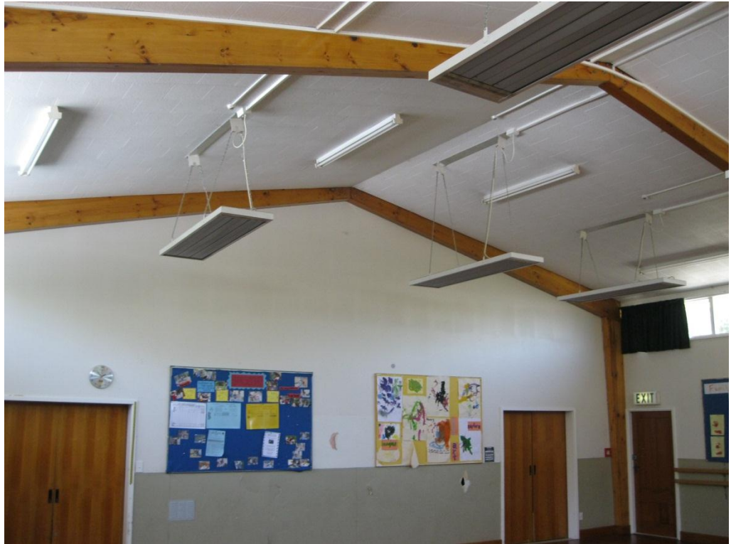
Photograph 5: Glulam timber portal frame.
