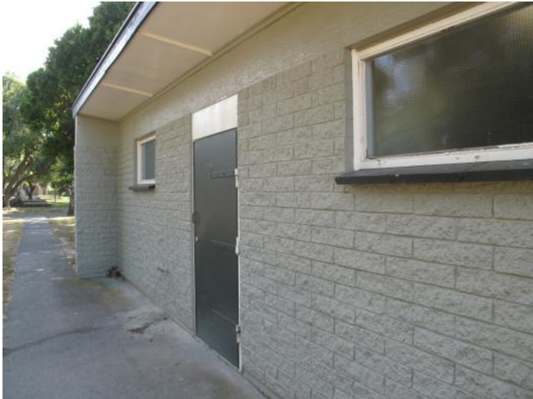
Photograph 3 Brick veneer on the exterior concrete masonry walls
