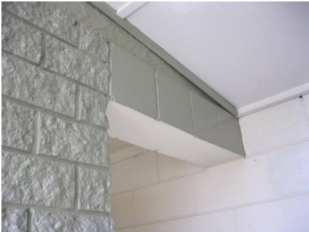
Photograph 6 Concrete masonry lintel beam
