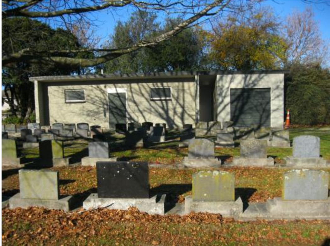
Photograph 1 North-western elevation of the building
