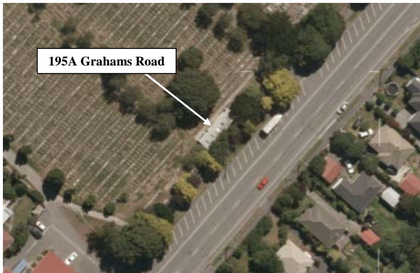
Figure 4 Post February 2011 Earthquake Aerial Photography 2
