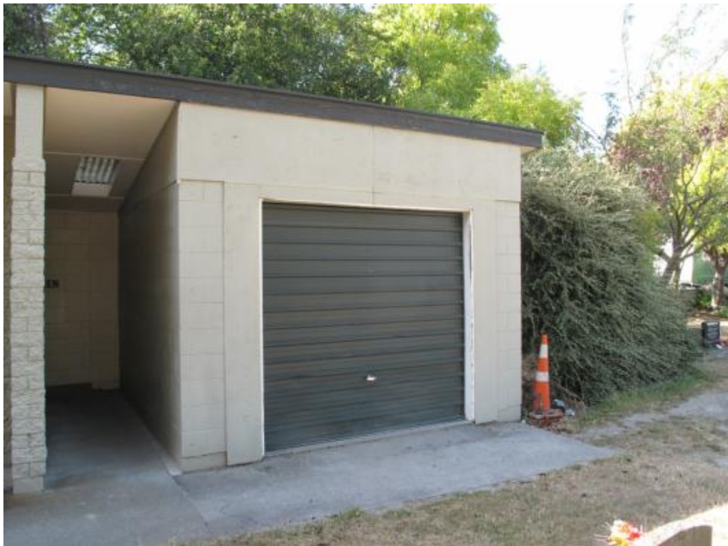
Photograph 4 Extension to the south-west of the original building
