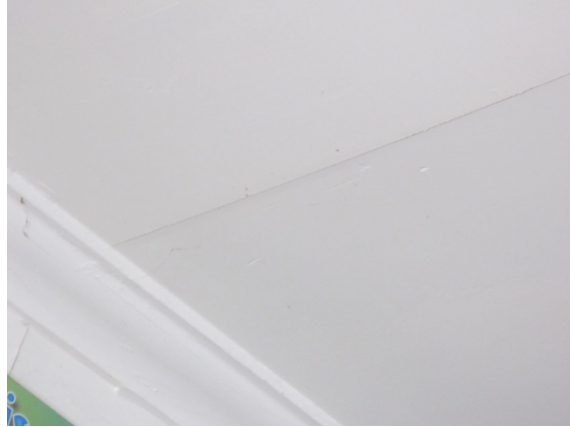
Photo 9: Gaps opening up between plasterboard ceiling cladding panels
