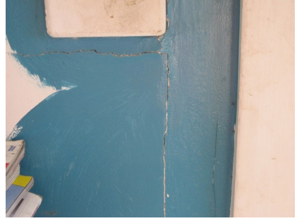
Photo 10: Gaps opening up between plasterboard wall cladding panels
