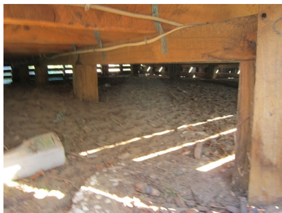
Photo 7: Timber framing and piles
