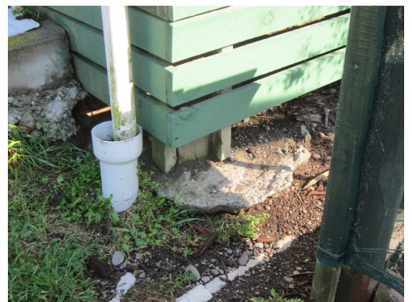
Photo 8: Timber piles in concrete footing
