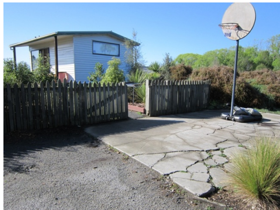
Photo 11: Heavily cracked concrete slab west of the building
