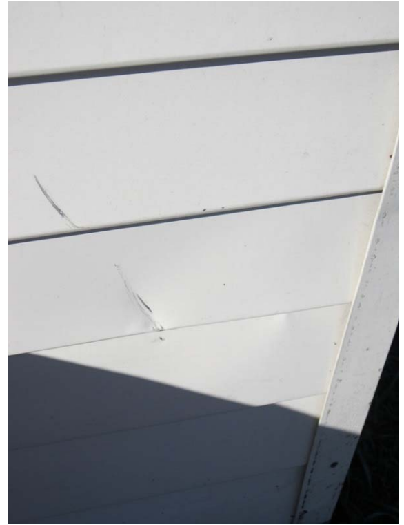
Photo 6: Impact damage to external profiled metal wall cladding
