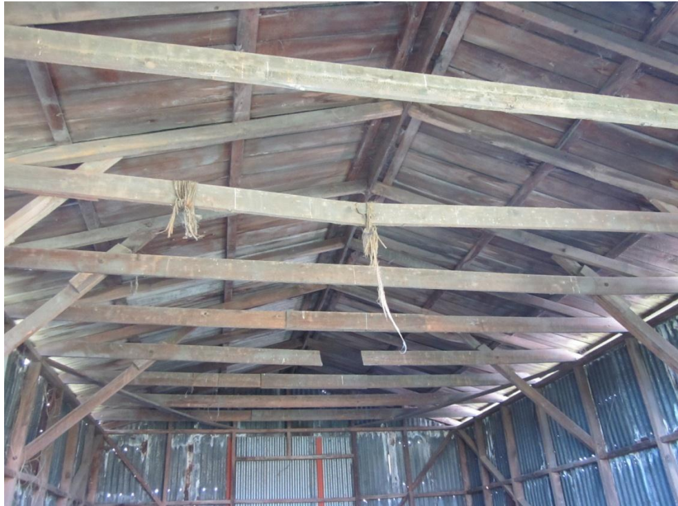
Photograph 5: Interior view of cross-braced and knee braced timber roof and cross-braced timber wall structures.
