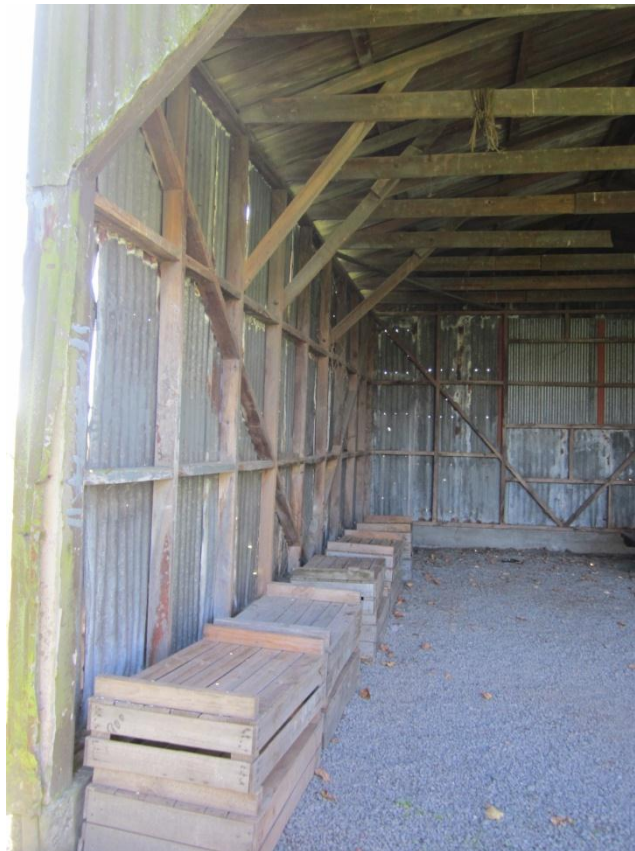
Photograph 6: Interior view of cross-braced external walls.
