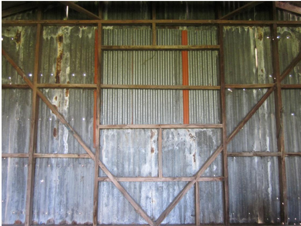
Photograph 11: Timber cross-bracing of north external wall.
