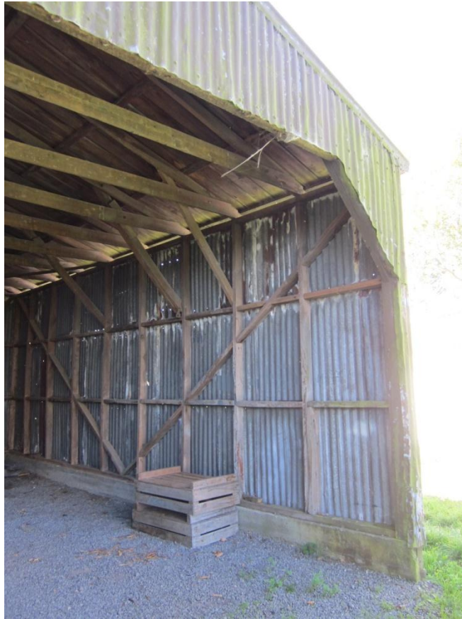
Photograph 7: Interior view of wall and roof structures and short concrete foundation wall.
