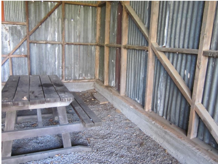
Photograph 8: Interior view of cross-braced timber walls and short concrete foundation walls.
