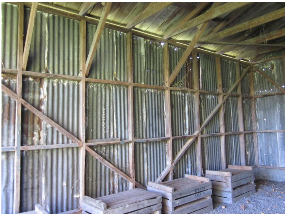
Photograph 10: Interior view of cross-braced timber walls and roof structure and short concrete foundation walls.
