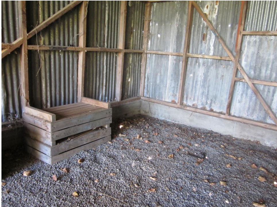
Photograph 9: Interior view of cross-braced timber walls and short concrete foundation walls.
