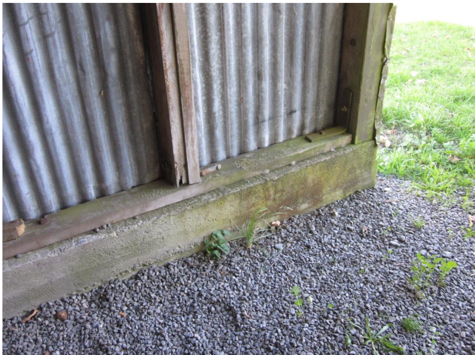
Photograph 12: Typical wall-to-foundation attachment.
