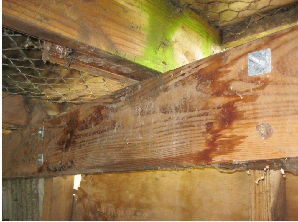
Photograph 15 Provision of bolts to the joint between rafters and timber post.
