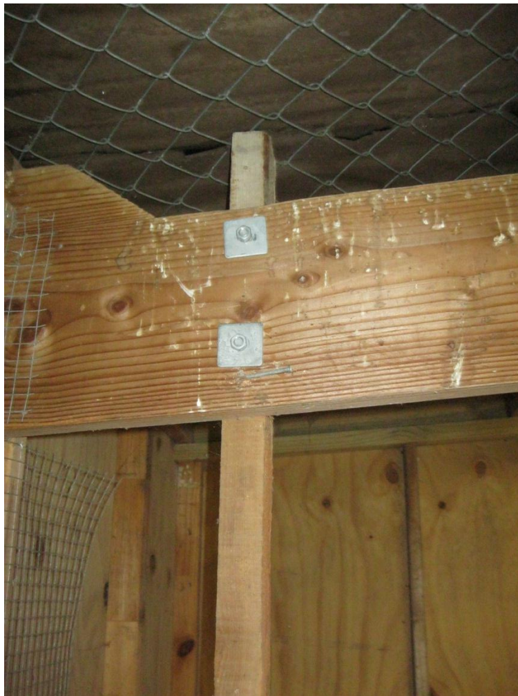
Photograph 14 Provision of bolts to the joint between rafters and timber post.
