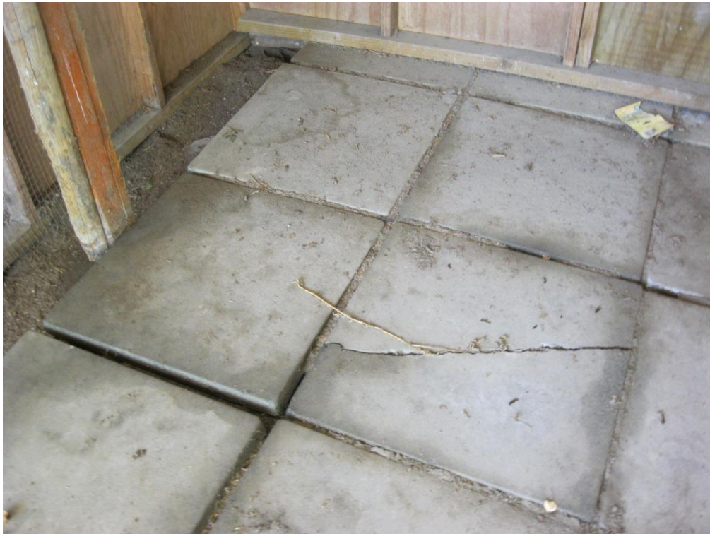
Photograph 11 Differential concrete tiles settlements.
