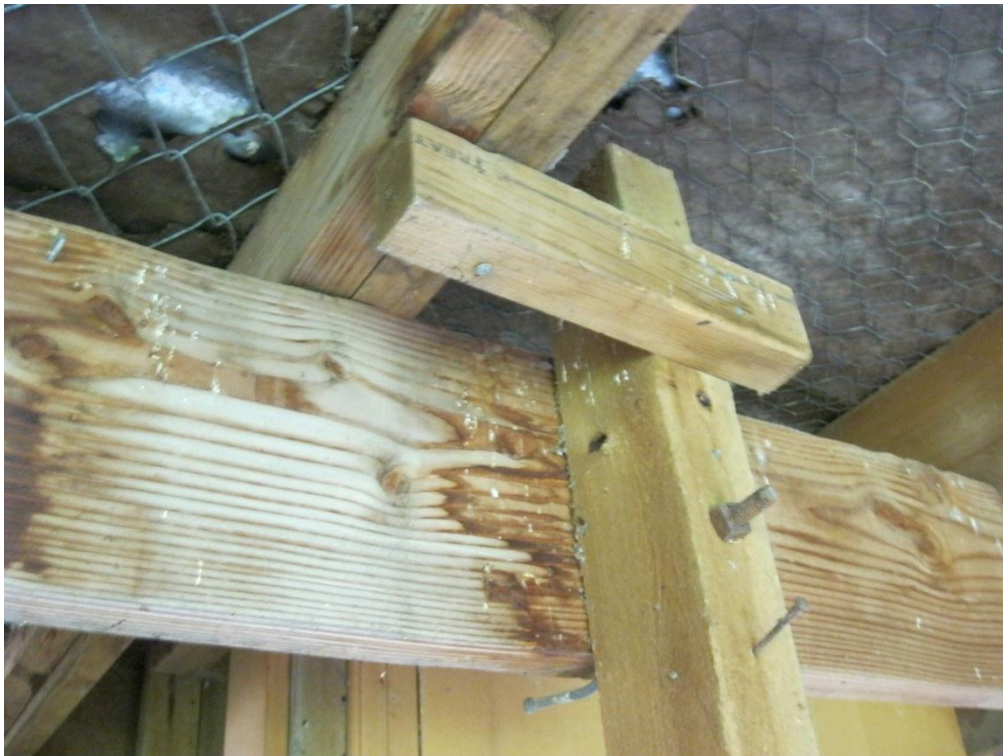
Photograph 10 Missing bolts of the joint between rafters and timber post.
