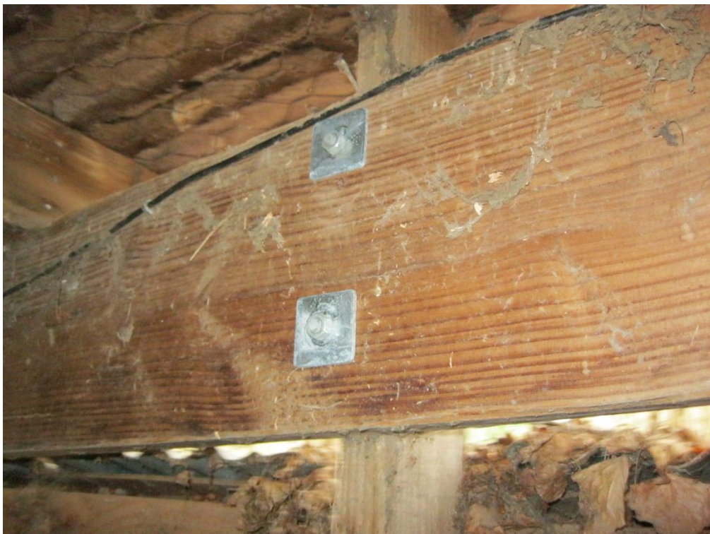
Photograph 12 A number of bolts provided to a connection.
