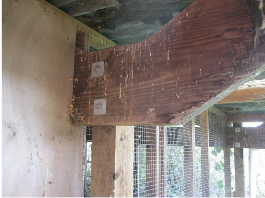
Photograph 13 Provision of bolts to the joint between rafters and timber post.
