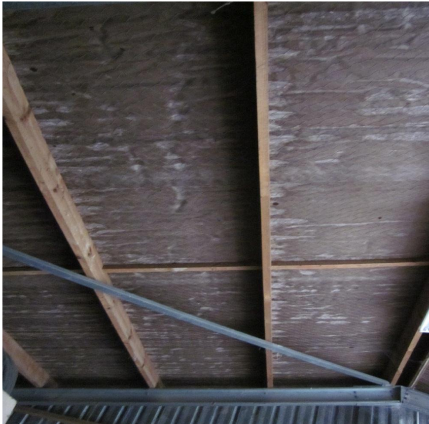
Photo 8 View of the diagonal roof bracing.
