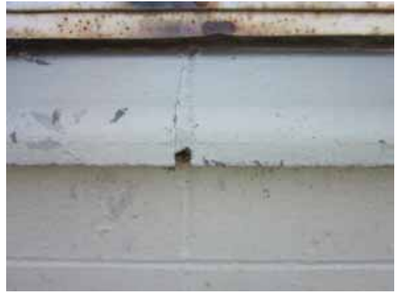
Photo 6: Cracking in the window sill and wall beneath the central window
