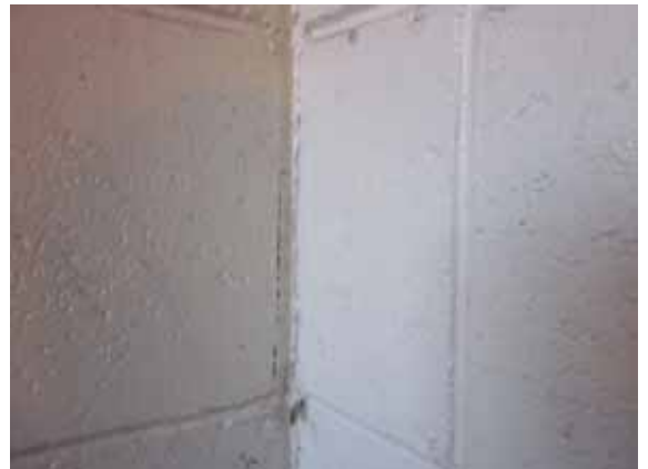
Photo 4: Typical separation between internal and perimeter masonry walls
