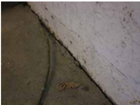
Photo 11: Separation between the internal floor slab in the shower room and the footing the masonry wall to the east
