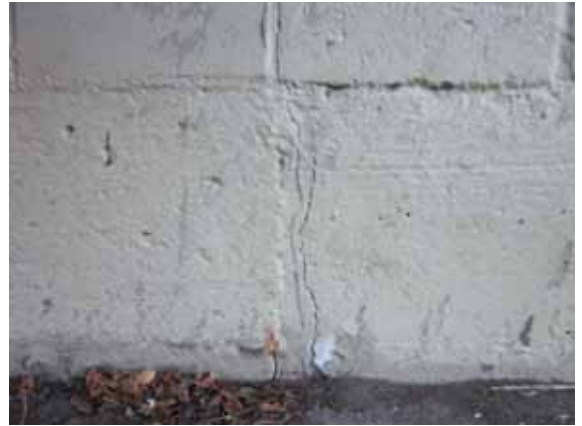
Photo 10: Detail of the footing at the junction showing separation
