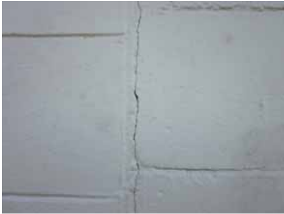
Photo 9: Detail of the junction showing separation between structures
