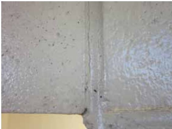
Photo 3: Typical vertical cracking in the mortar at each end of the lintels of door and window openings
