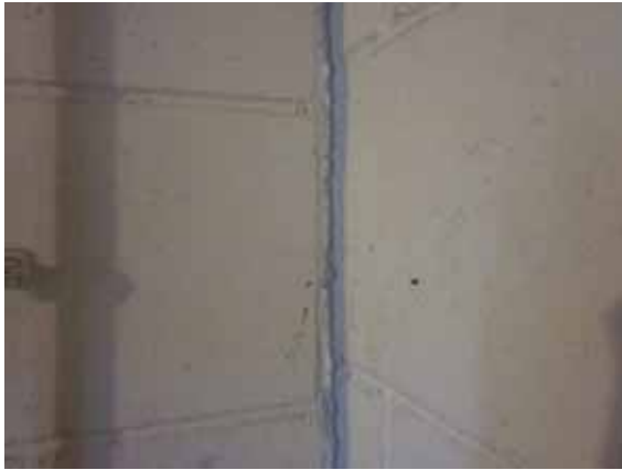
Photo 13: Typical detail of sealant used on the interior of the building at the central junction between structures
