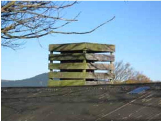
Photo 17: Timber framing for the water tank fixed to the roof of the building. Note damage to lower plank and lean in the structure
