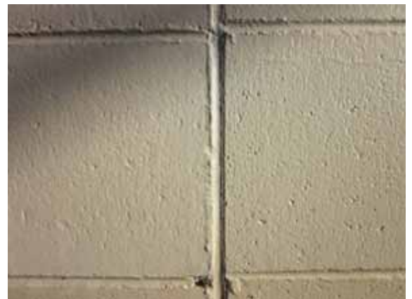
Photo 16: Detail of the separation between the westernmost extension and the adjacent structure
