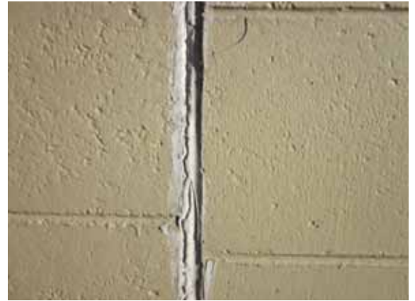
Photo 14: Detail of the sealant on the exterior of the north wall at the central junction between structures
