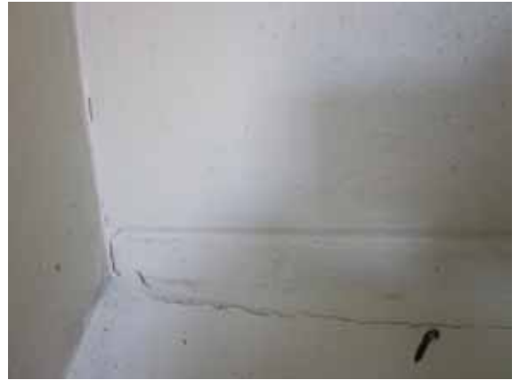
Photo 18: Typical damage to the paint at the junction between internal timber framing and the perimeter masonry walls
