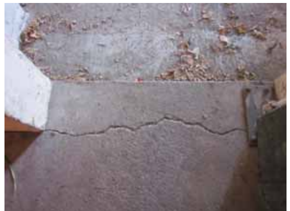
Photo 12: Cracking in the internal floor slab over the footing to the east of the shower room
