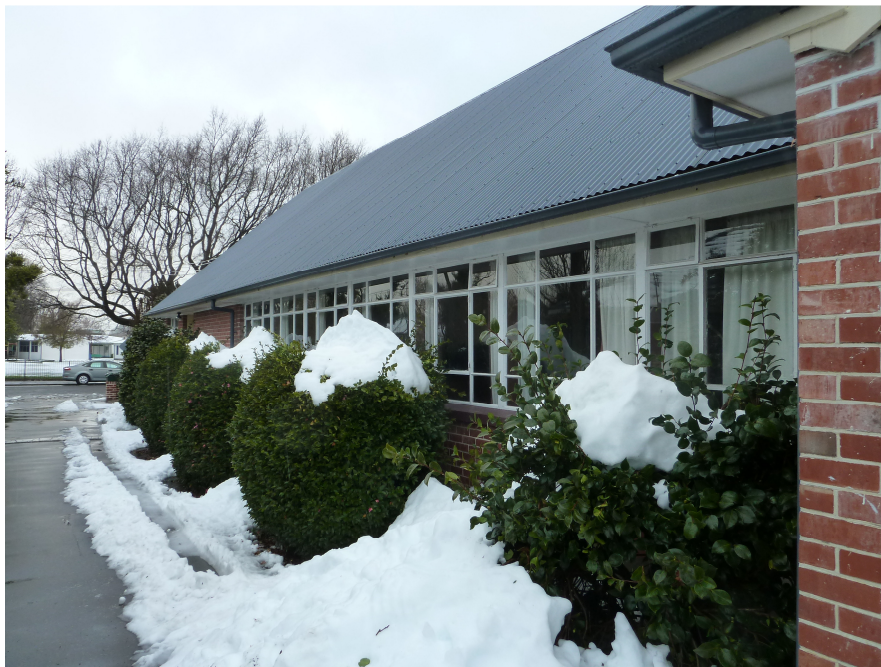
Photo 2 – General view of the building
