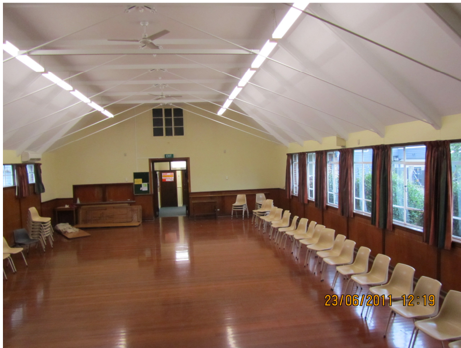
Photo 3 – Interior of Hall showing ceiling line and steel rafter ties
