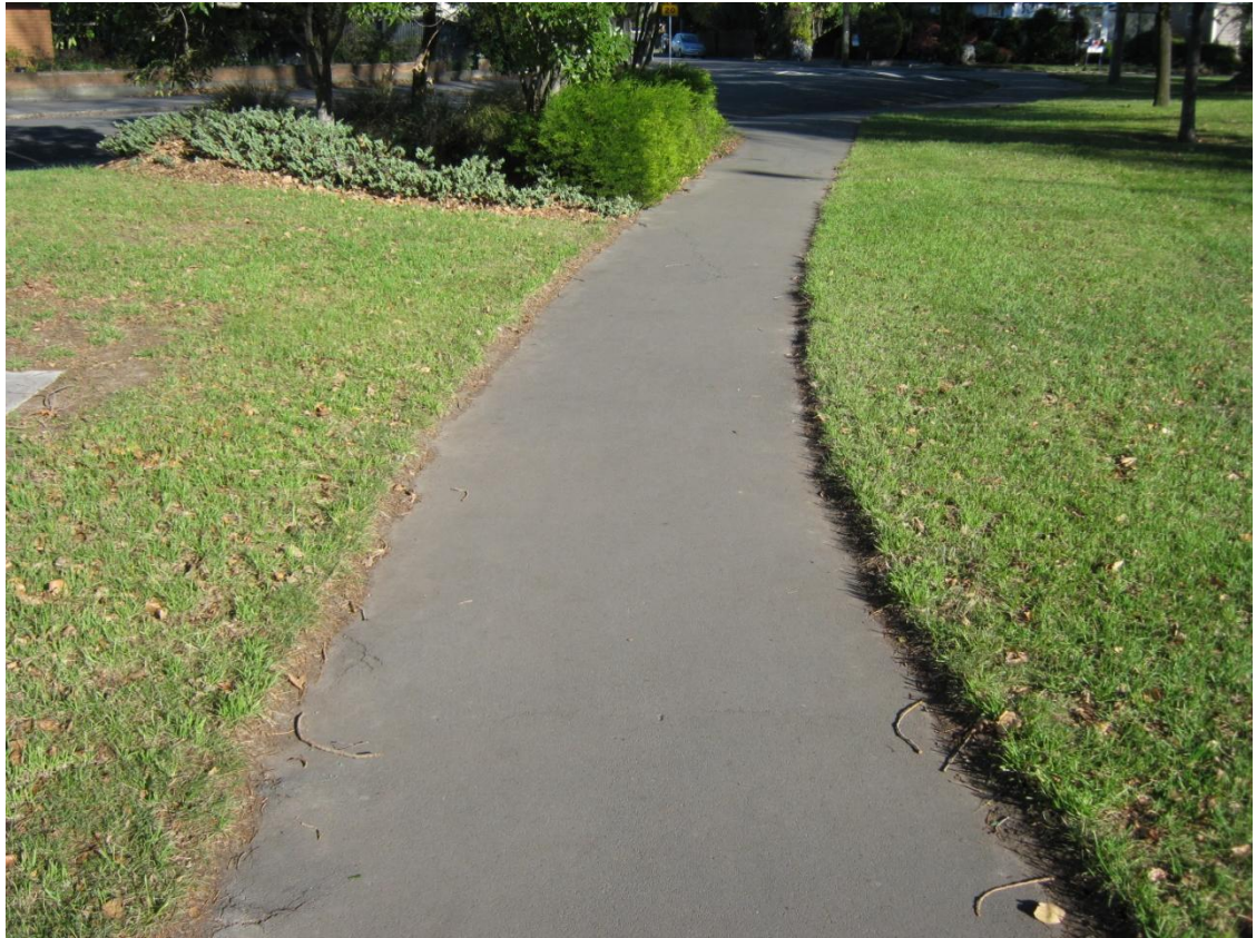
■ Figure 8 - Minor cracking of the path asphalt surface
