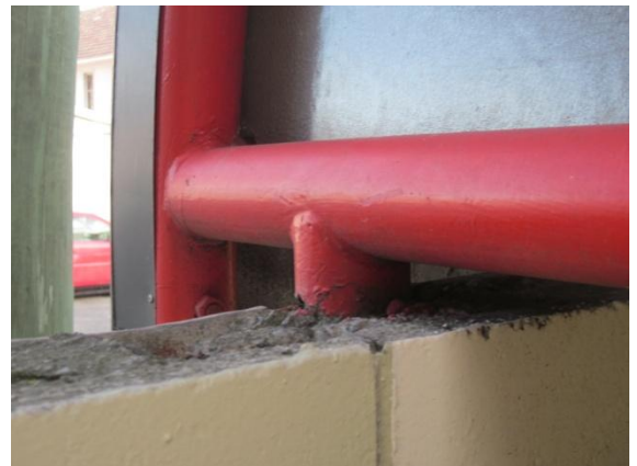
Photo 4: Detail of the steel posts cast in to the walls of the building
