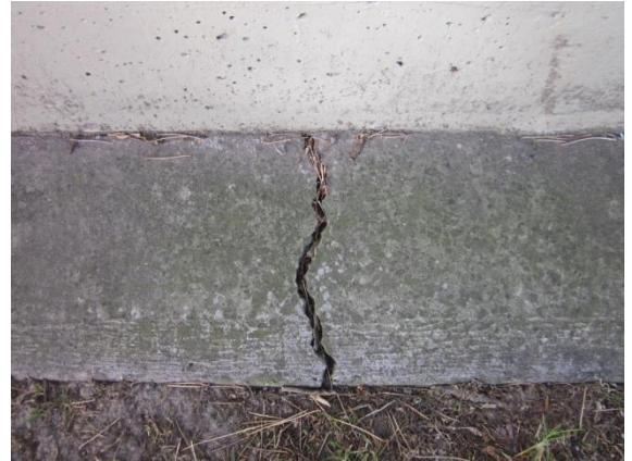
Photo 6: Existing cracking in the narrow slab that have been exacerbated by the recent seismic activity
