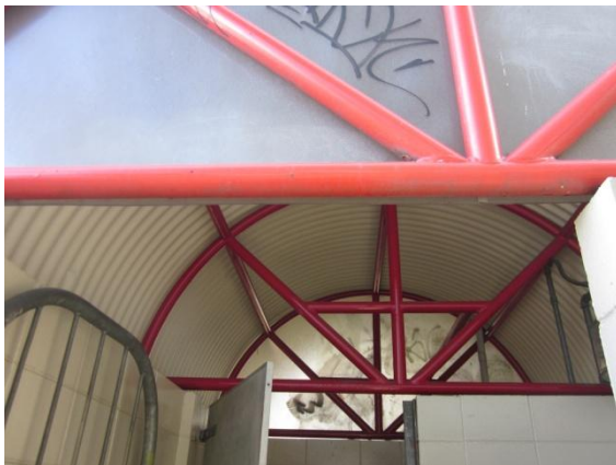
Photo 3: The steel canopy framing
