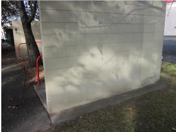
Photo 5: The narrow external concrete slab on the west, south and east sides of the building
