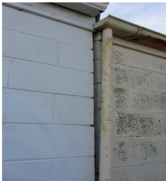
Photo 7: 25mm separation between the south elevation of the garage and the storage shed (1)
