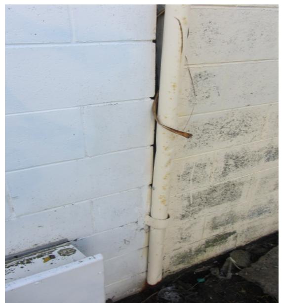
Photo 8: 25mm separation between the south elevation of the garage and the storage shed (2)
