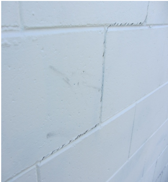
Photo 5: Close up view of steps cracks through mortar joints in photo 4
