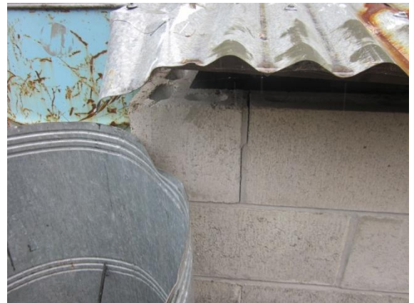
Photo 4: Cracking to Mortar in the NE Corner
