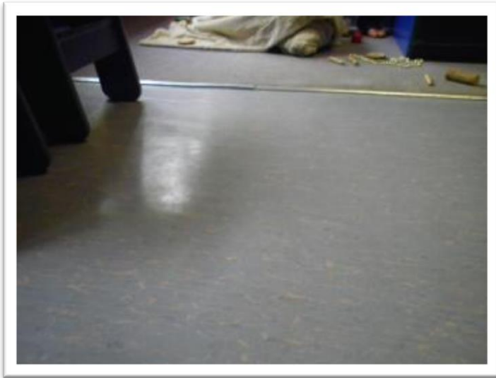
Nursery floor where distortion in lino is observed (appeared after earthquake)
