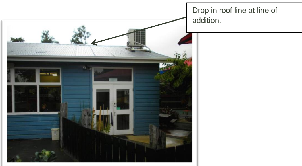
Play Centre North elevation – Note drop in roof line where new section added (this is in line with the distortion in the floor of the play centre)
