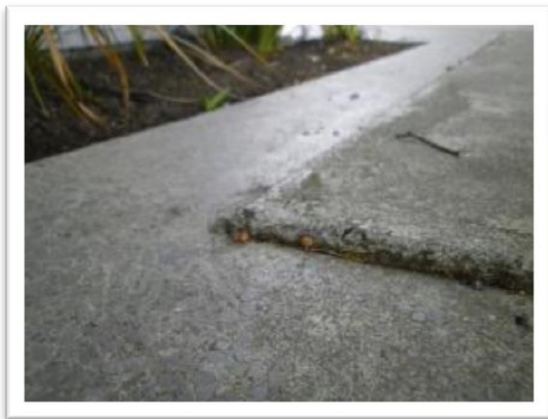
Uneven Concrete slab outside entrance to library
