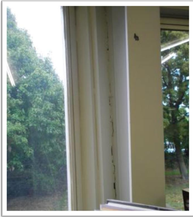
Cracking between window frame and steel column
