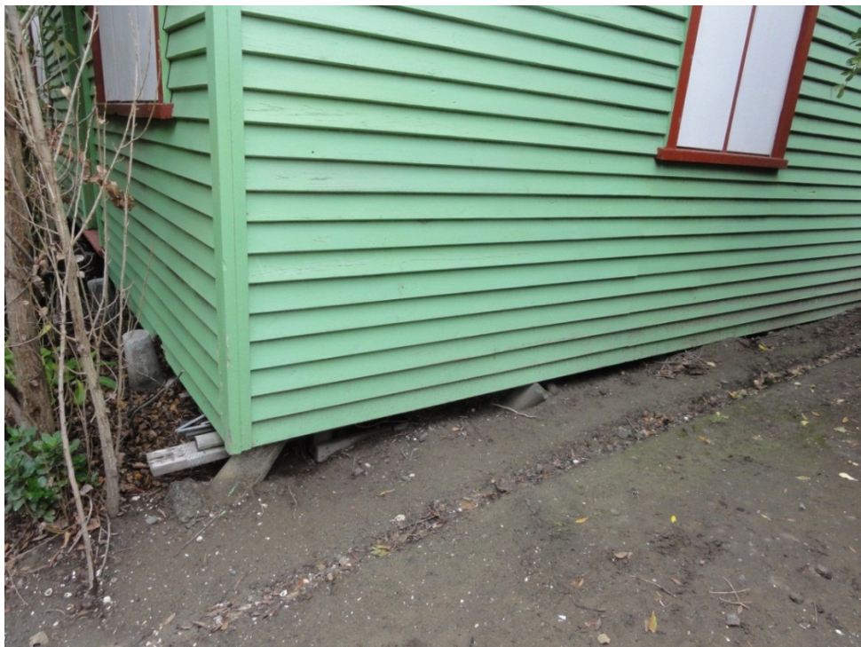
Figure 6: Foundation damage to the neighbouring building towards the north.
