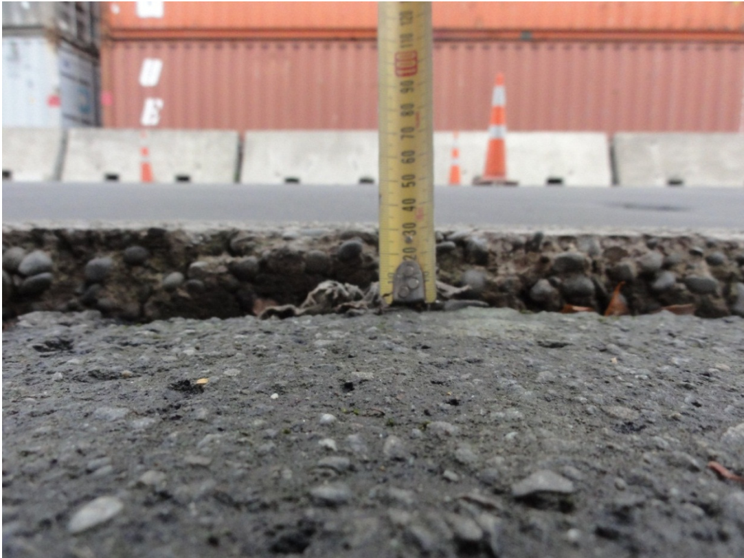
Figure 3: Main Road footpath has settled 30mm relative to the kerb.
