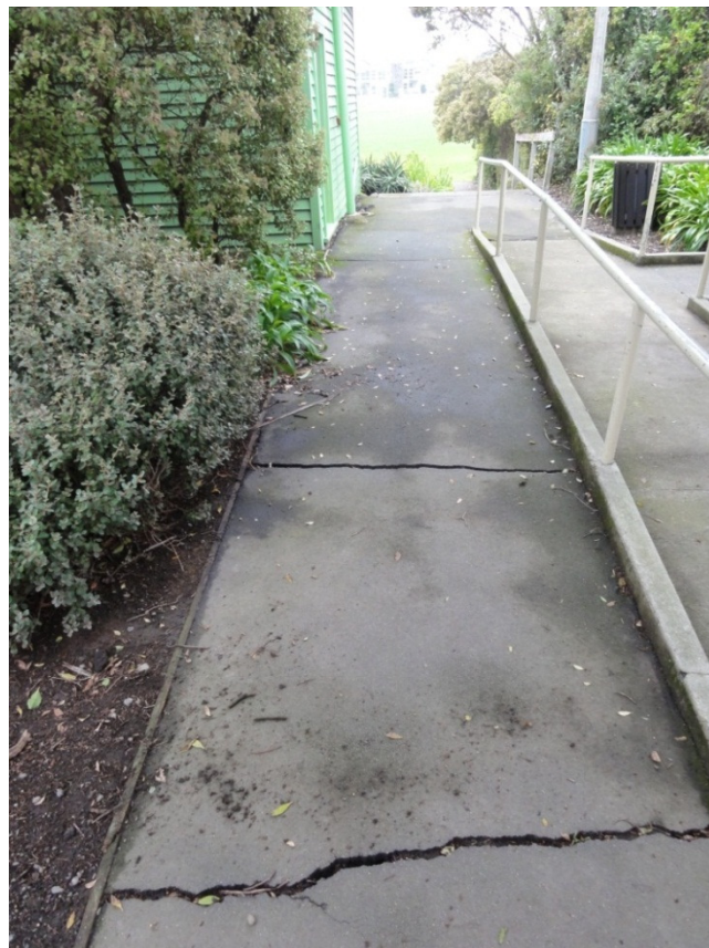
Figure 2: 20mm to 30mm wide cracking of the paved footpath north of the building
