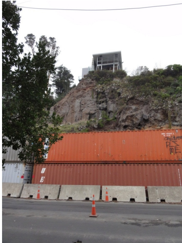
Figure 5: Shipping containers are being used as a rockfall protection scheme along the western side of the Main Road.
