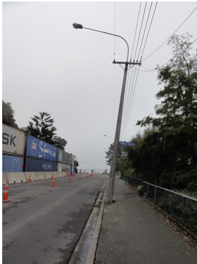
Figure 4: Street Lights along Main Road lean towards the east.
