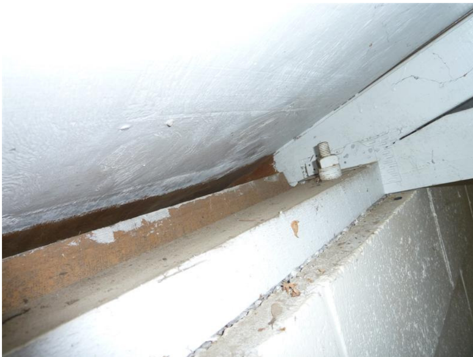
Truss, top plate connection to masonry bond beam
