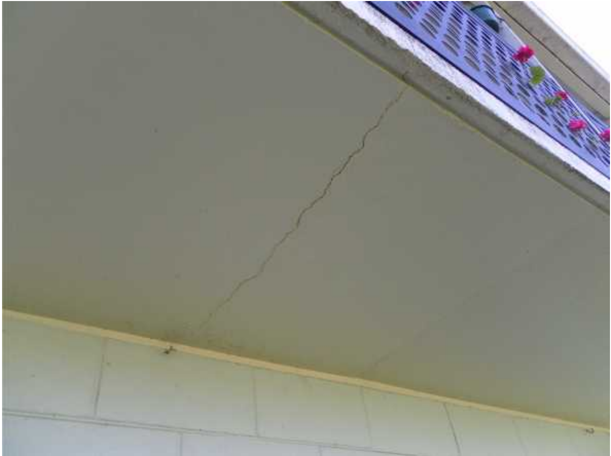
Photo 16: Underside of typical first floor balcony.
