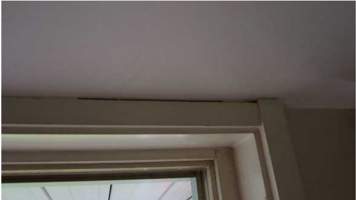
Photo 10: Door architrave and ceiling.
