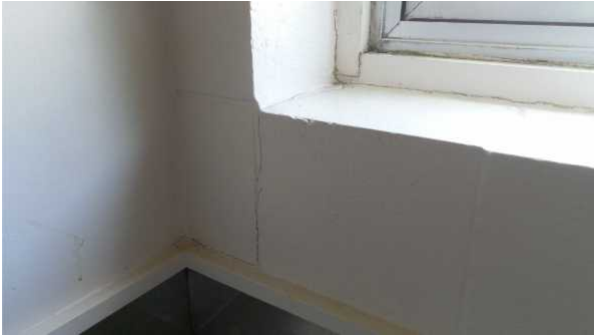
Photo 22: Inner skin (15series) of concrete masonry block wall – ground floor in Block C.
