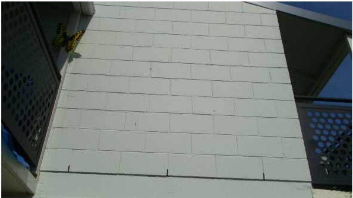
Photo 19: Concrete masonry block wall – Block C.
