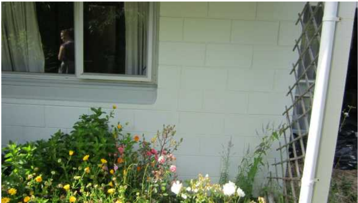
Photo 7: Concrete block masonry veneer – Block A.
