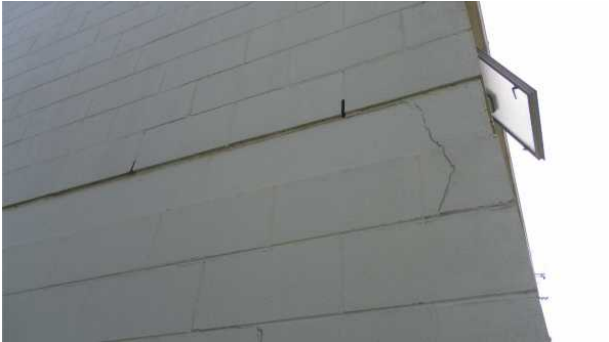
Photo 18: First floor slab – Western end wall in Block C.
