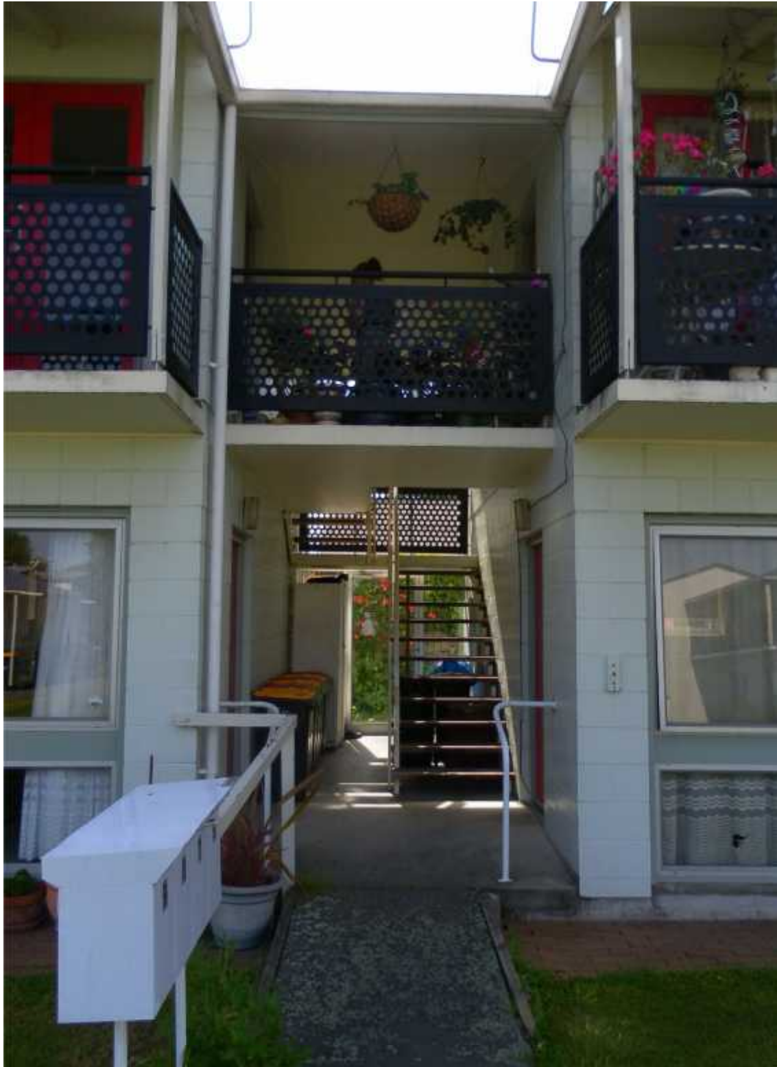
Photo 5: Intra-block stairs. Detail is typical for the three sets of stairs in Block C, as well as the set of stairs in Block B. The stair landings are the dividing feature/seismic separation between each block (refer to Section 11.1).
