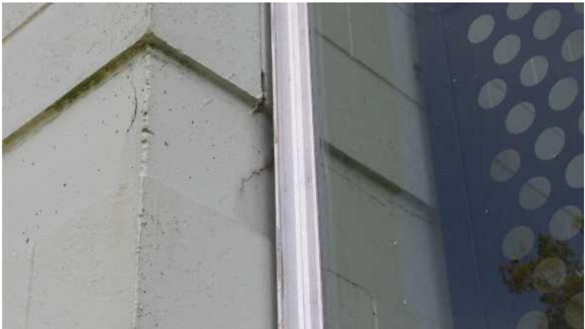
Photo 17: First floor slab – Block C.
