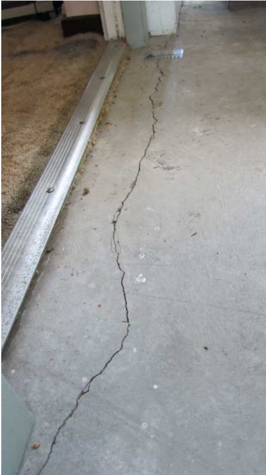
Photo 13: Stair landing in Block C.
