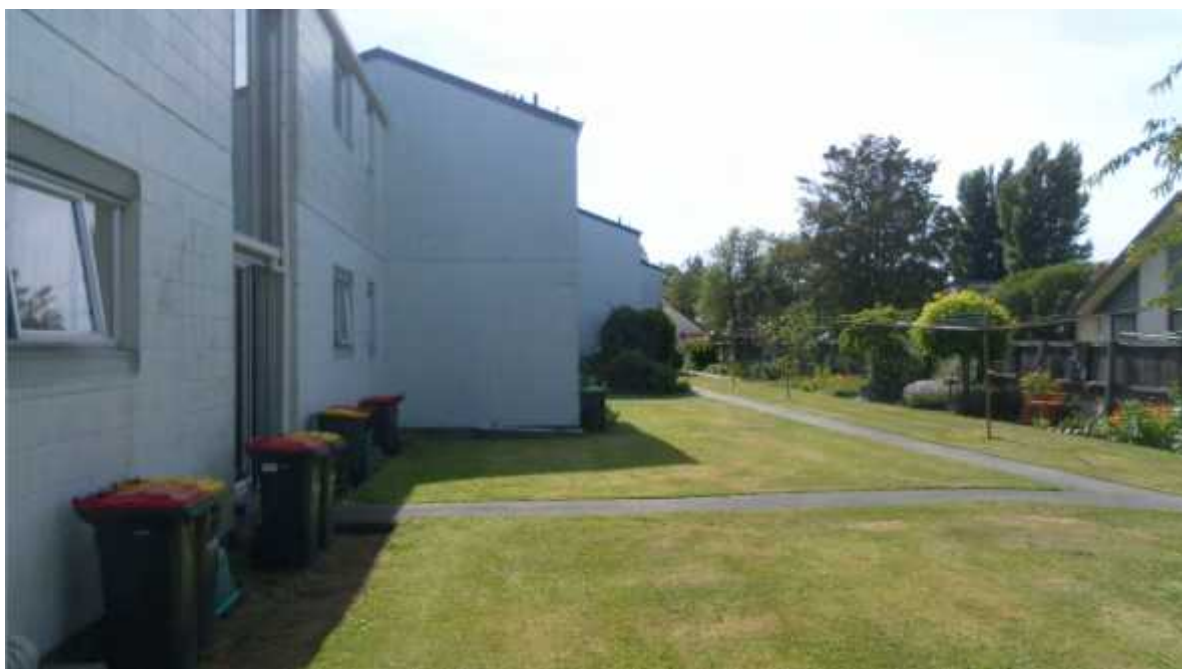
Photo 4: Rear of Block C - view from west.
