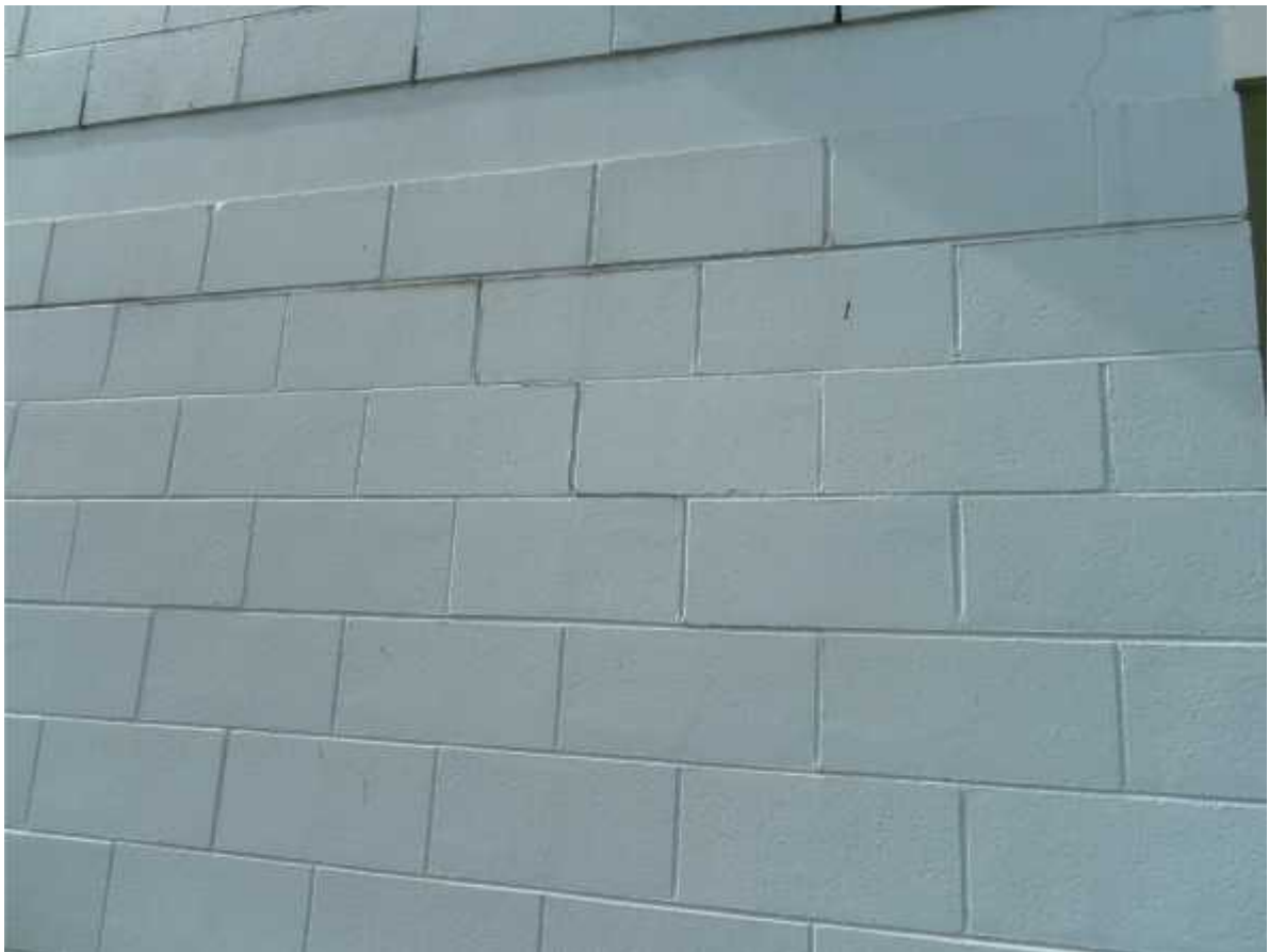
Photo 15: Reinforced concrete masonry block wall – northern end wall of Block B.
