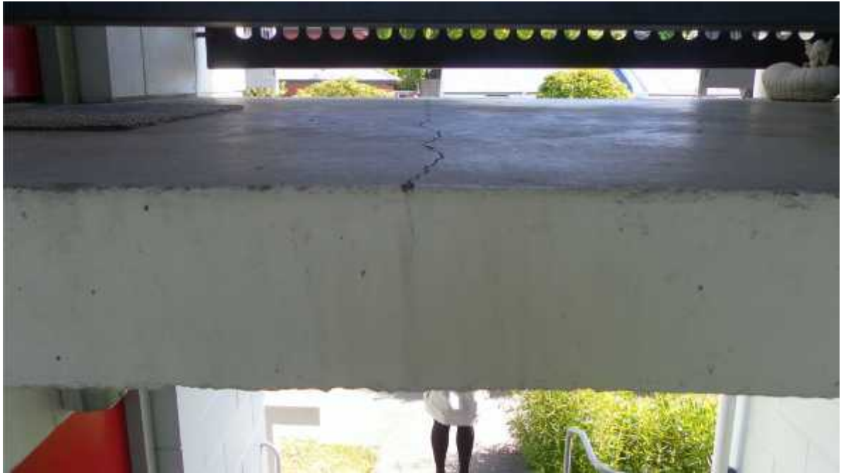
Photo 14: Stair landing in Block C.
