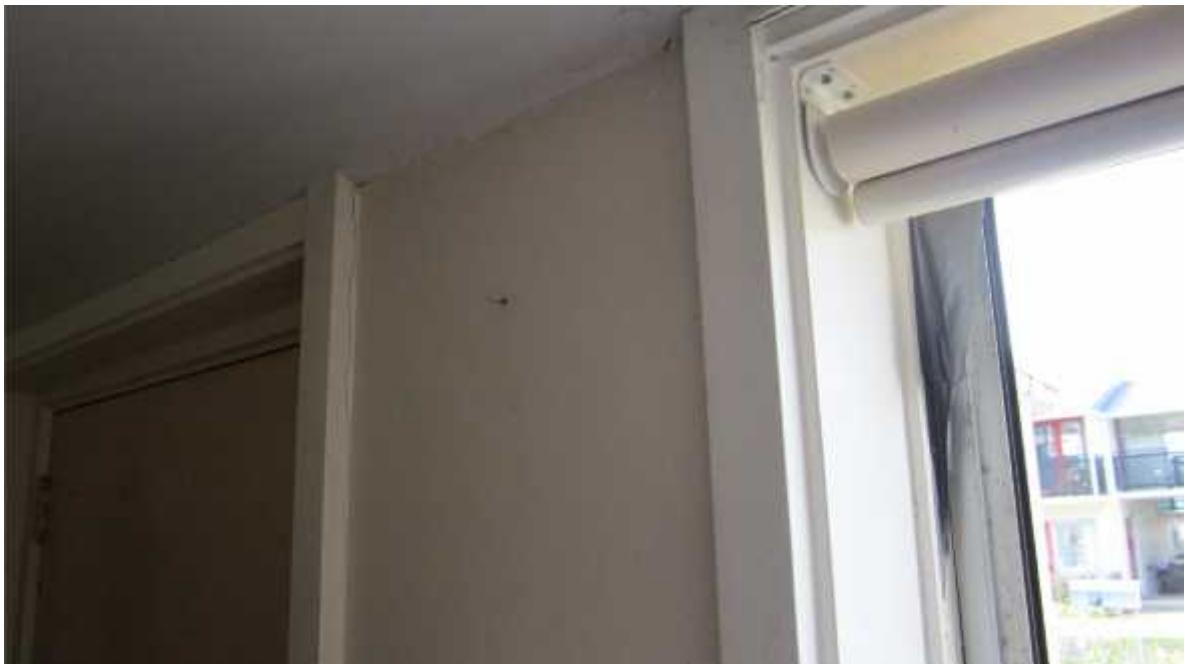
Photo 11: Window and door architrave and ceiling.
