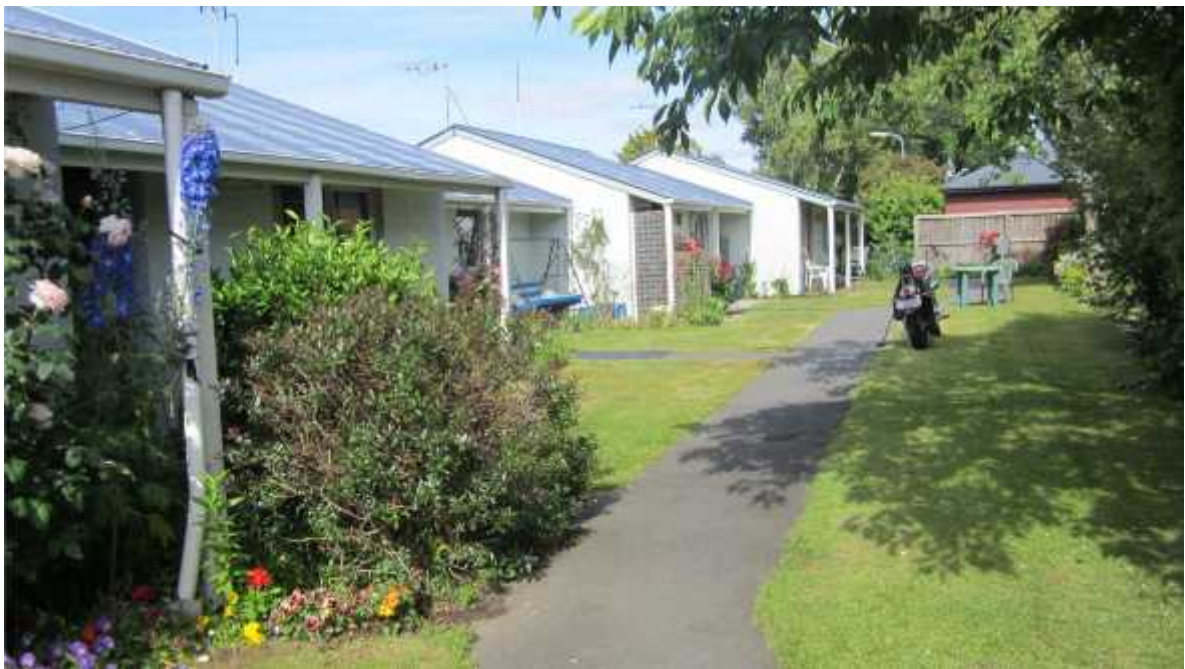
Photo 2: Block A - view from north east showing surrounding asphalt pavement.
