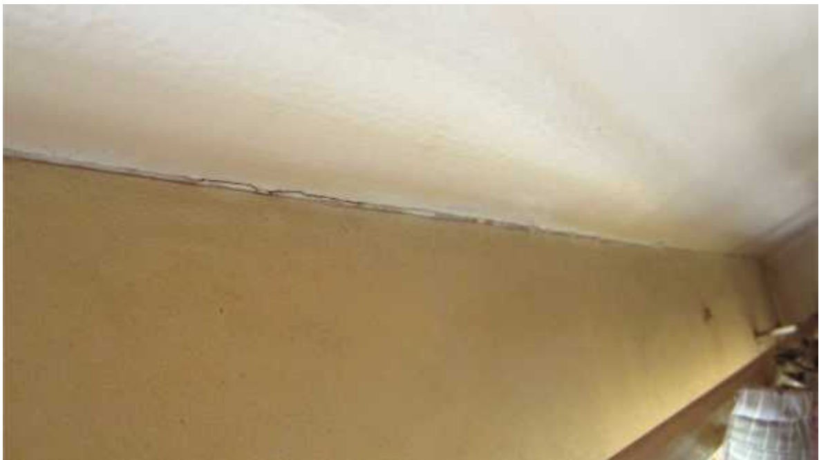
Photo 9: Internal wall and ceiling.
