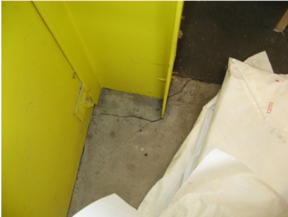
Photo 16: Typical cracking to concrete slab.
