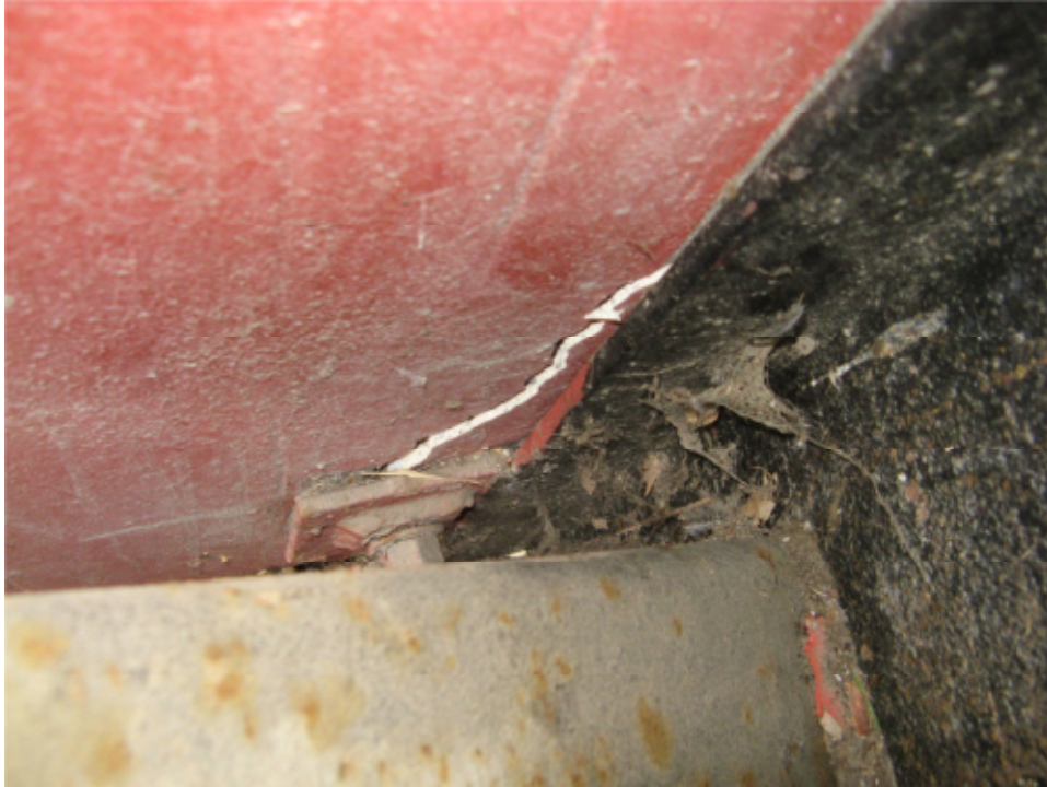
Photo 13: Panel connection with concrete cracking at southern corner of building
