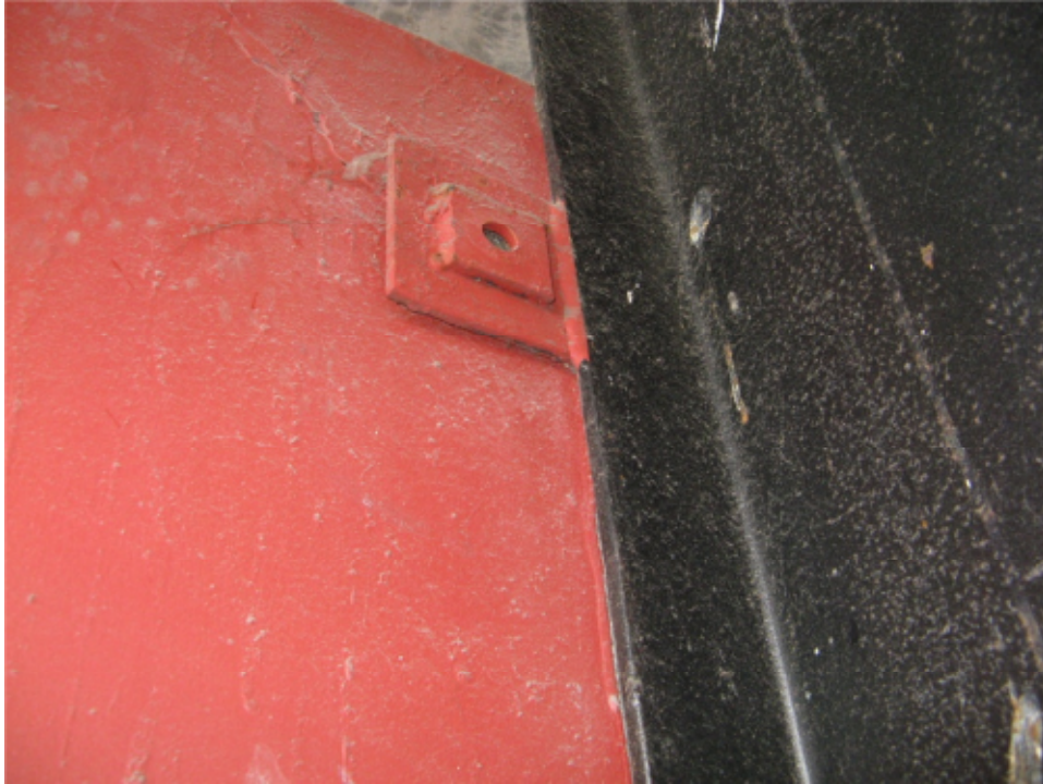
Photo 11: Panel connection with missing bolt at southern corner of building
