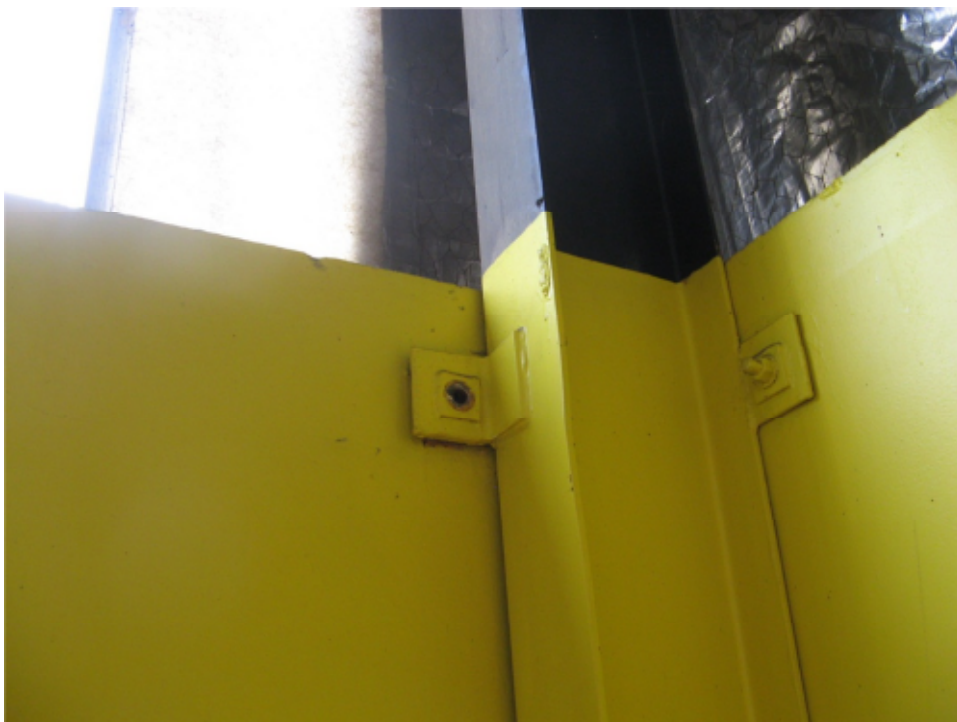
Photo 9: Panel connection with missing bolt at north corner of building
