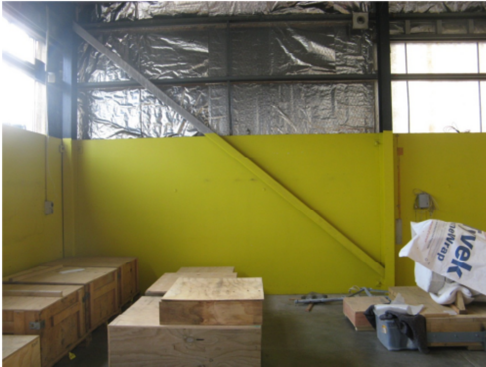
Photo 9: Tension/Compression brace with large connection eccentricities at each end.
