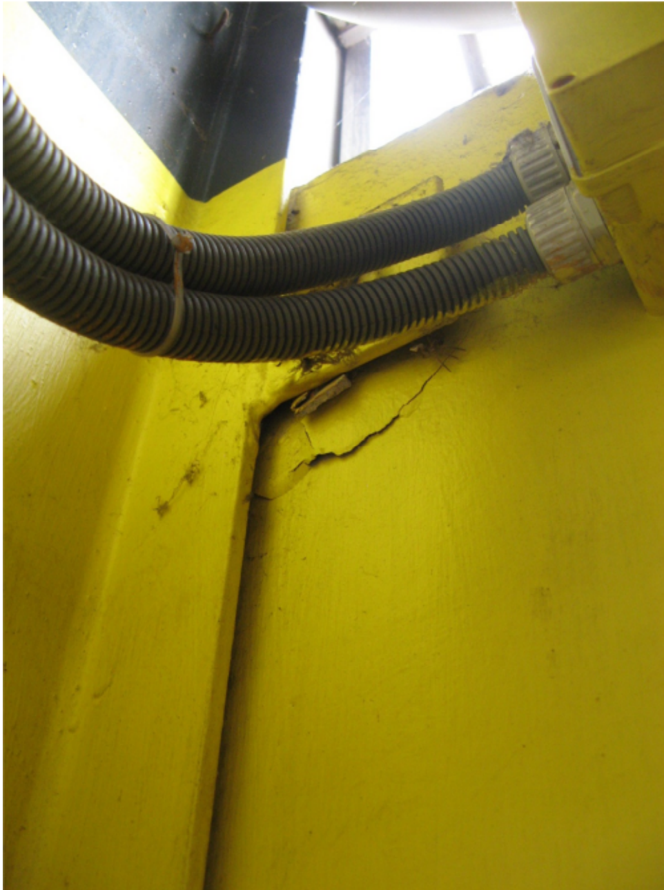
Photo 11: Panel connection with concrete spalling.
