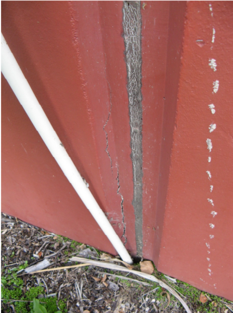
Photo 8: Typical cracking to concrete wall panel
