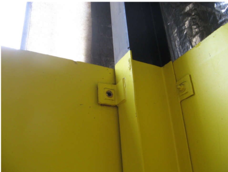
Photo 10: Panel connection with missing bolt at north corner of building.
