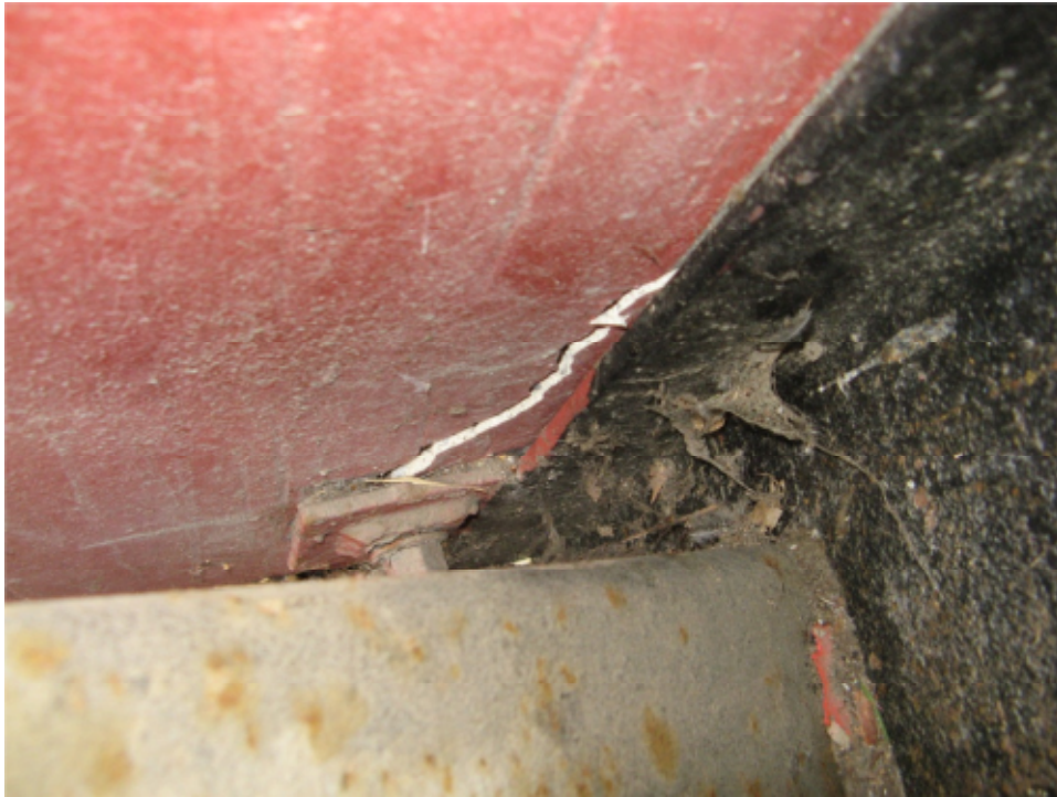
Photo 14: Panel connection with concrete cracking at southern corner of building.
