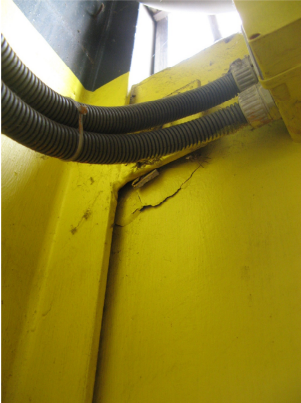
Photo 10: Panel connection with concrete spalling
