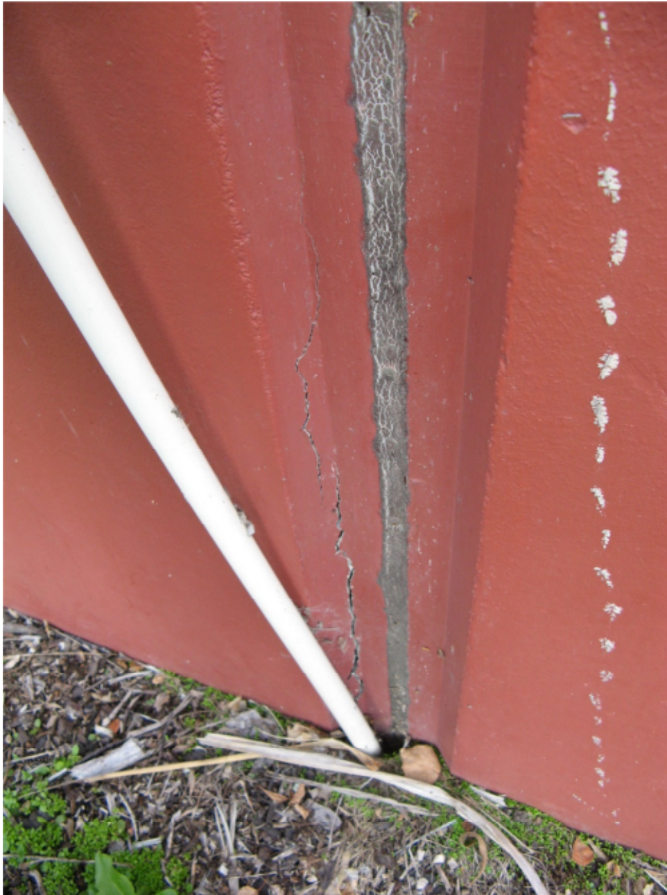
Photo 8: Typical cracking to concrete wall panel.
