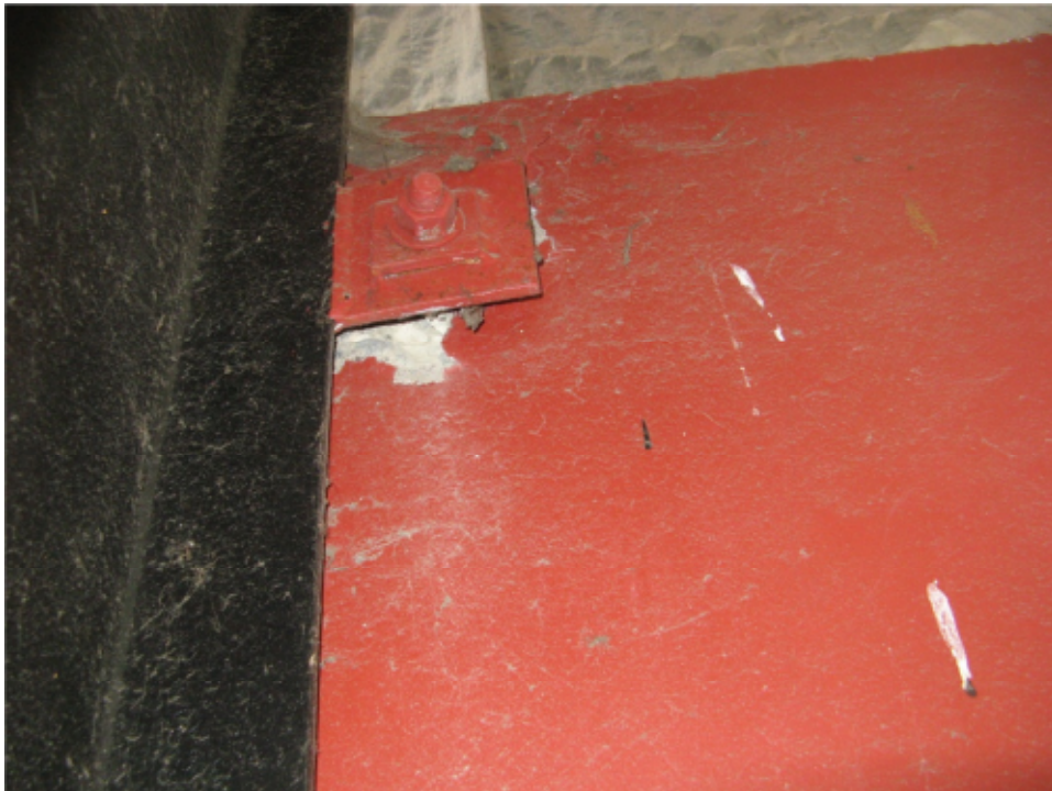
Photo 12: Panel connection with concrete spalling at southern corner of building
