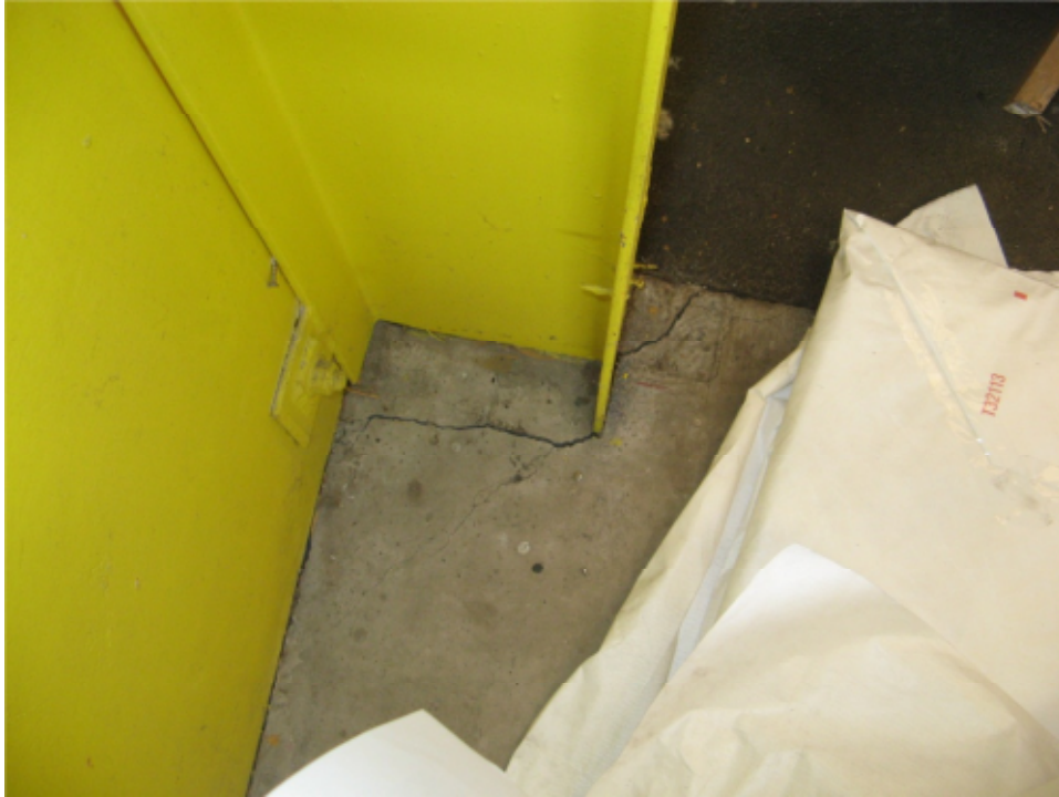
Photo 15: Typical cracking to concrete slab
