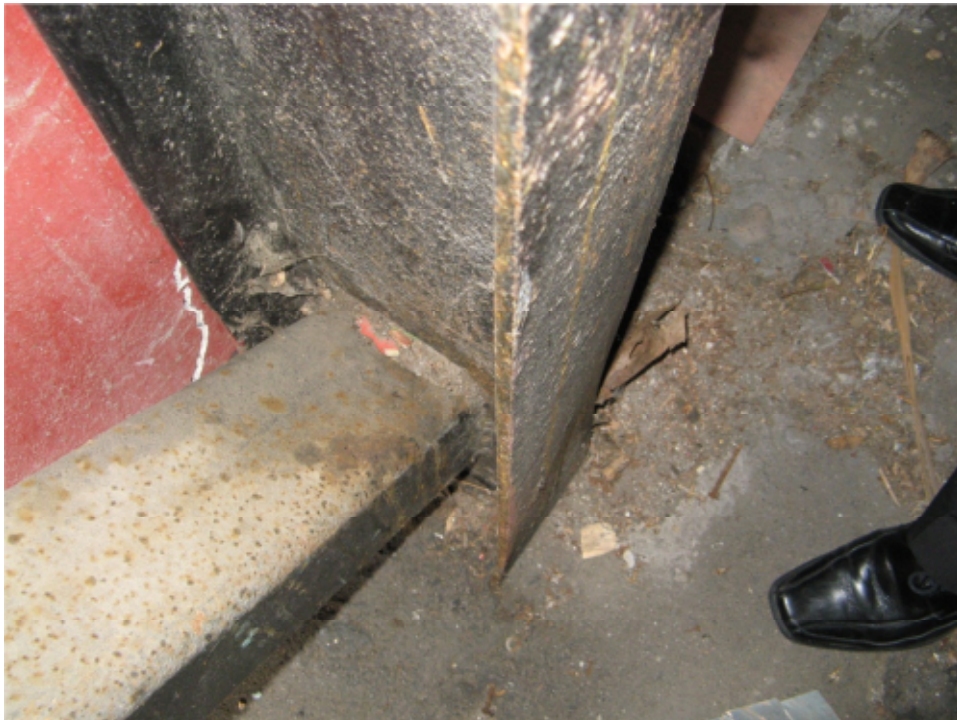
Photo 14: Tension/compression brace connection at southern corner of building
