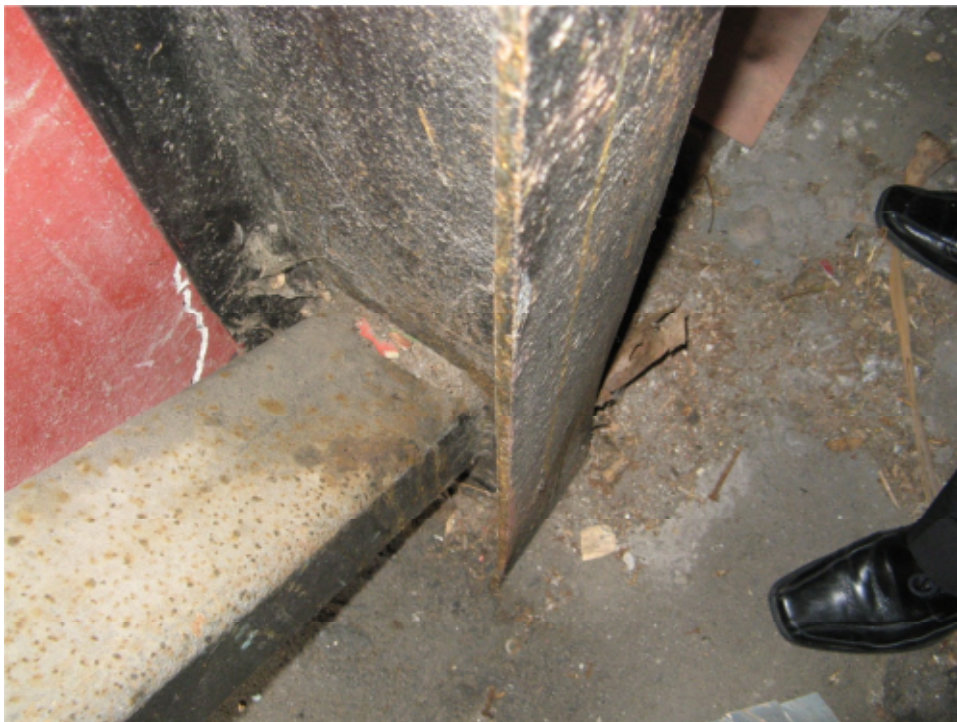
Photo 15: Tension/compression brace connection at southern corner of building.
