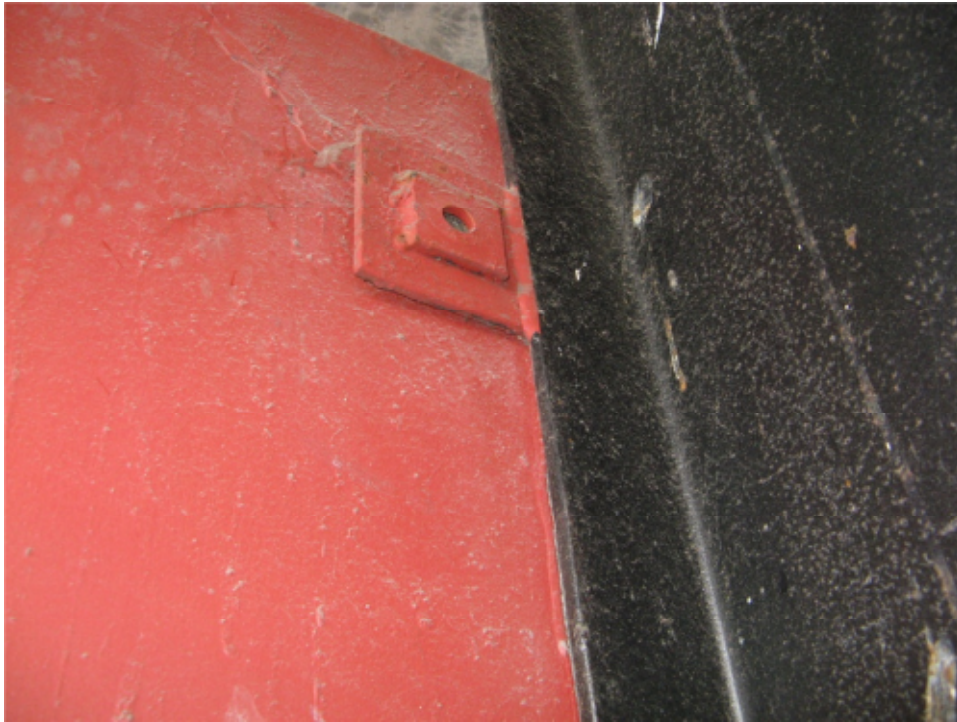
Photo 12: Panel connection with missing bolt at southern corner of building.
