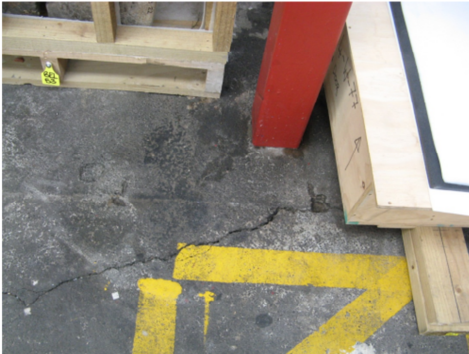
Photo 15: Cracking to asphalt pavement
