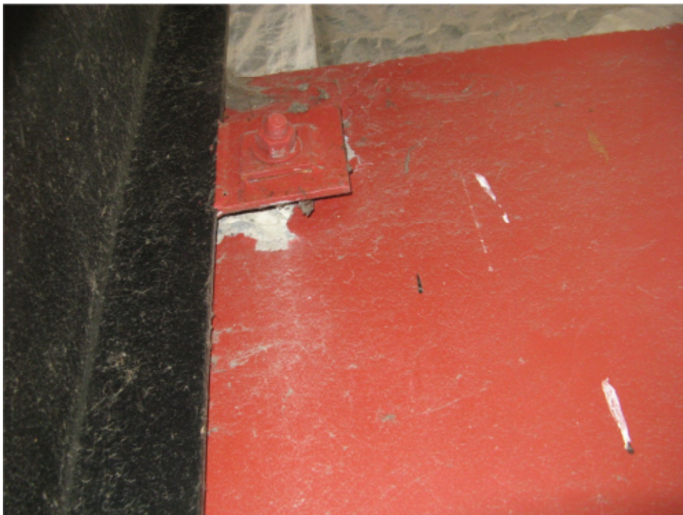
Photo 13: Panel connection with concrete spalling at southern corner of building.
