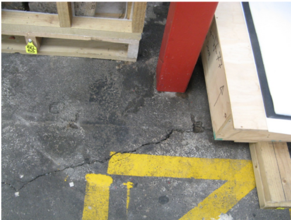
Photo 17: Cracking to asphalt pavement.
