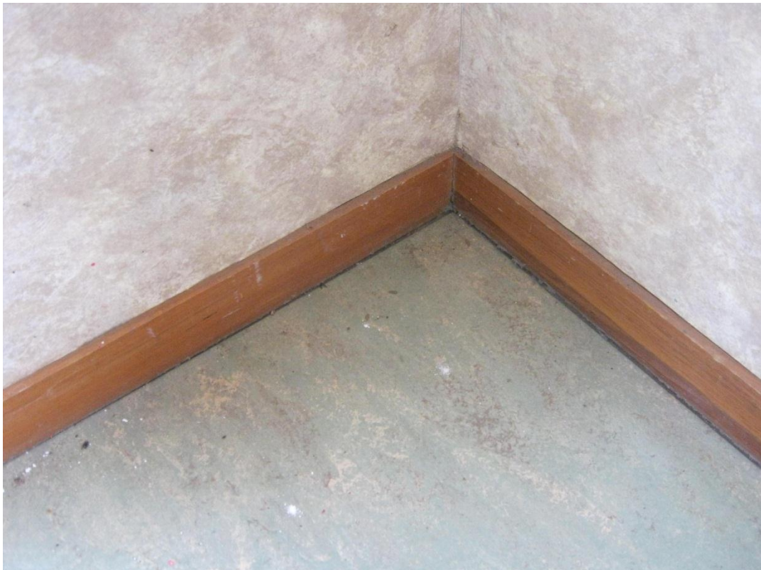
Photo 6: Settlement of the floor in the north west corner of the main room in the eastern wing.
