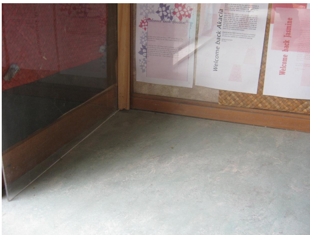
Photo 4: Approximately 10mm settlement of the floor in the large room in west wing.
