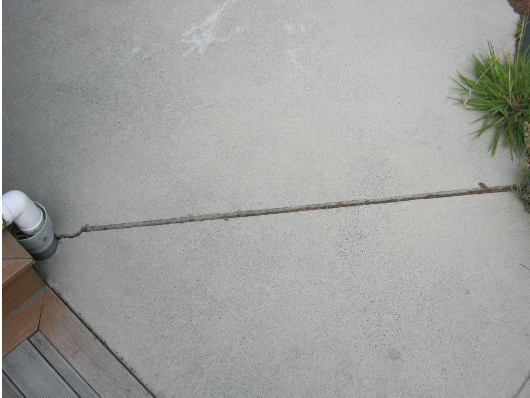
Photo 5: Separation and cracking of concrete shrinkage cut.
