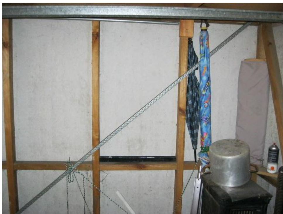
Photograph 6: Interior view of wall bracing at longitudinal wall.
