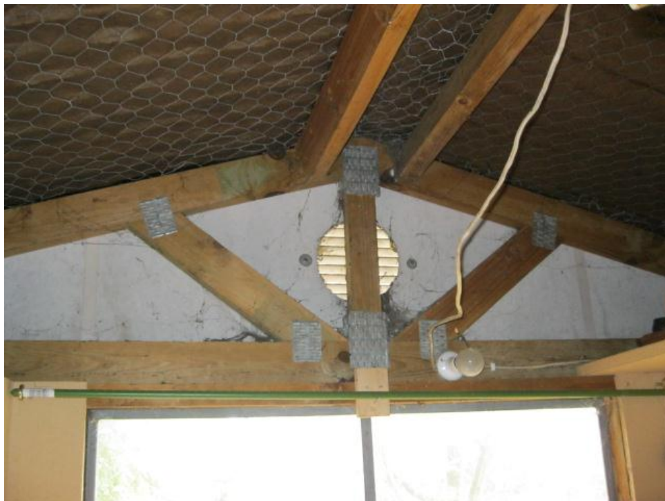
Photograph 7: Interior view of roof structure, which has no cross-bracing.
