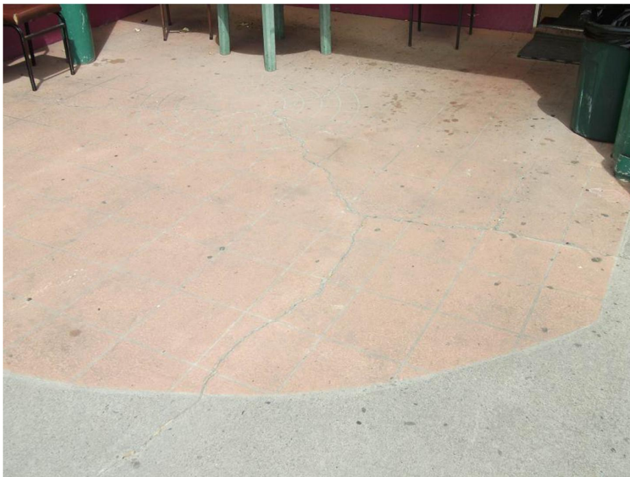
Photo 6: Typical slab cracking
