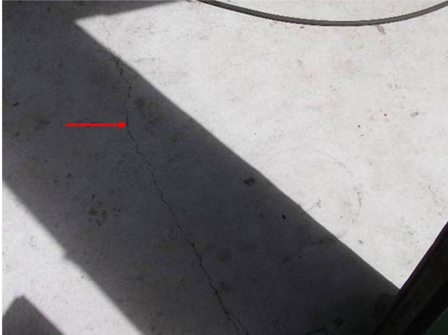
Photo 12: Typical slab cracking
