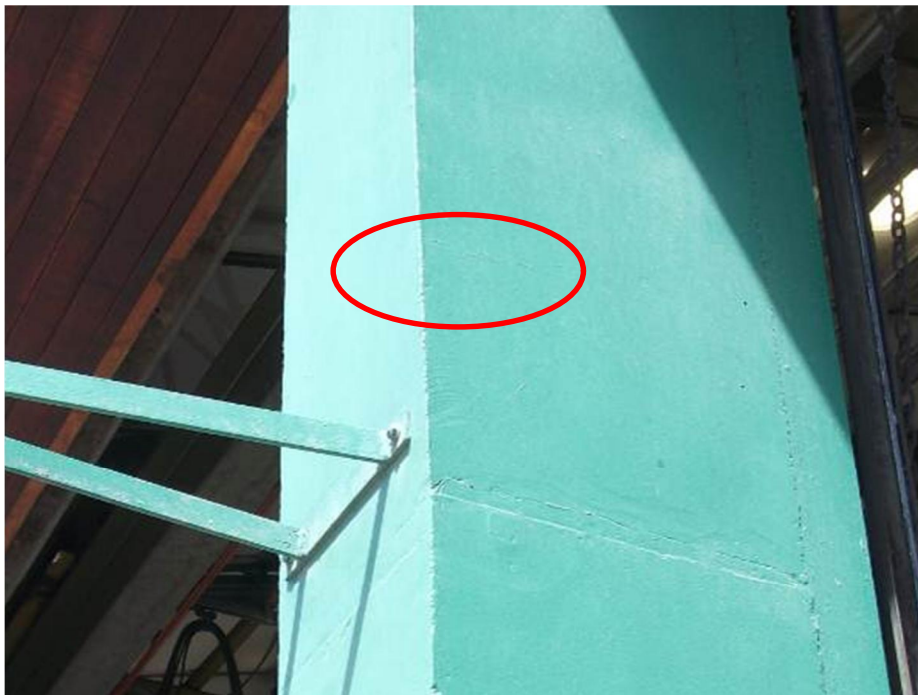
Photo 8: Typical cracking to concrete encasement of column.
