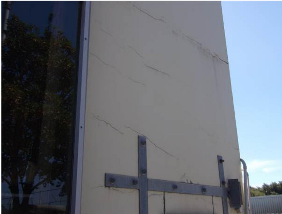
Photo 9: Typical cracking to concrete shear walls at corners of building.
