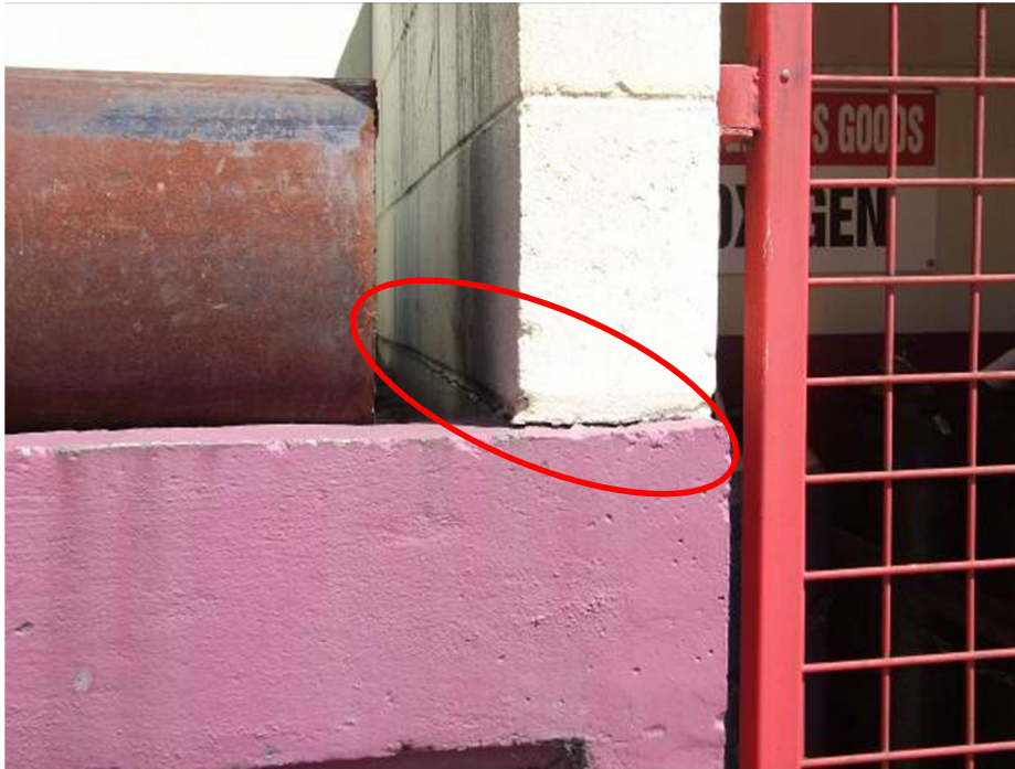
Photo 13: Cracking to oxygen tank storage blockwork
