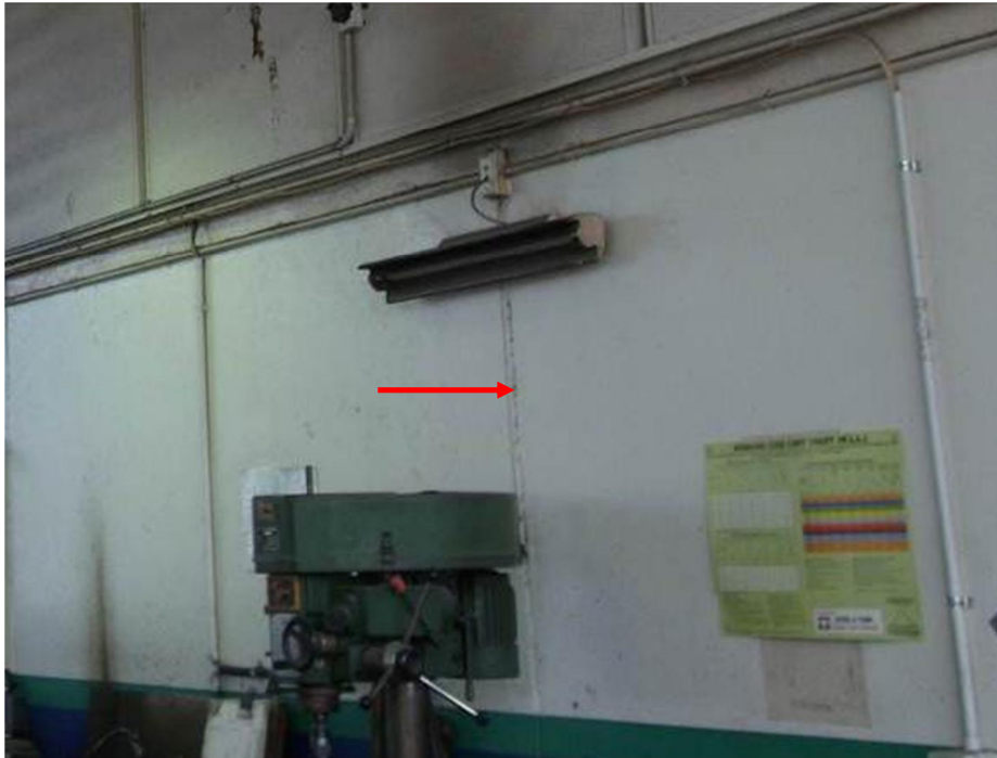
Photo 11: Typical cracking along movement joints
