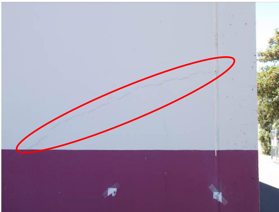
Photo 10: Typical cracking to concrete shear walls at corners of building
