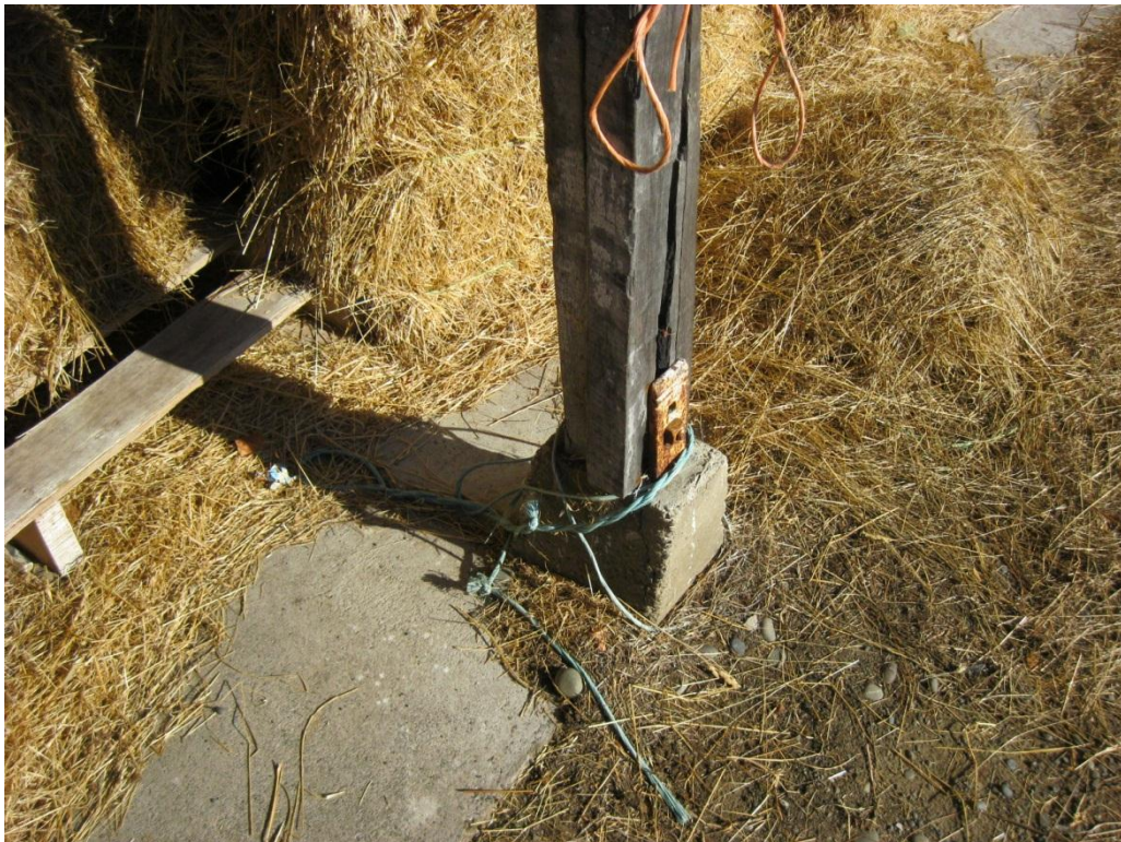
Photograph 6 Cracking to the timber post at the north-west wall. It is not believed to be earthquake related.
