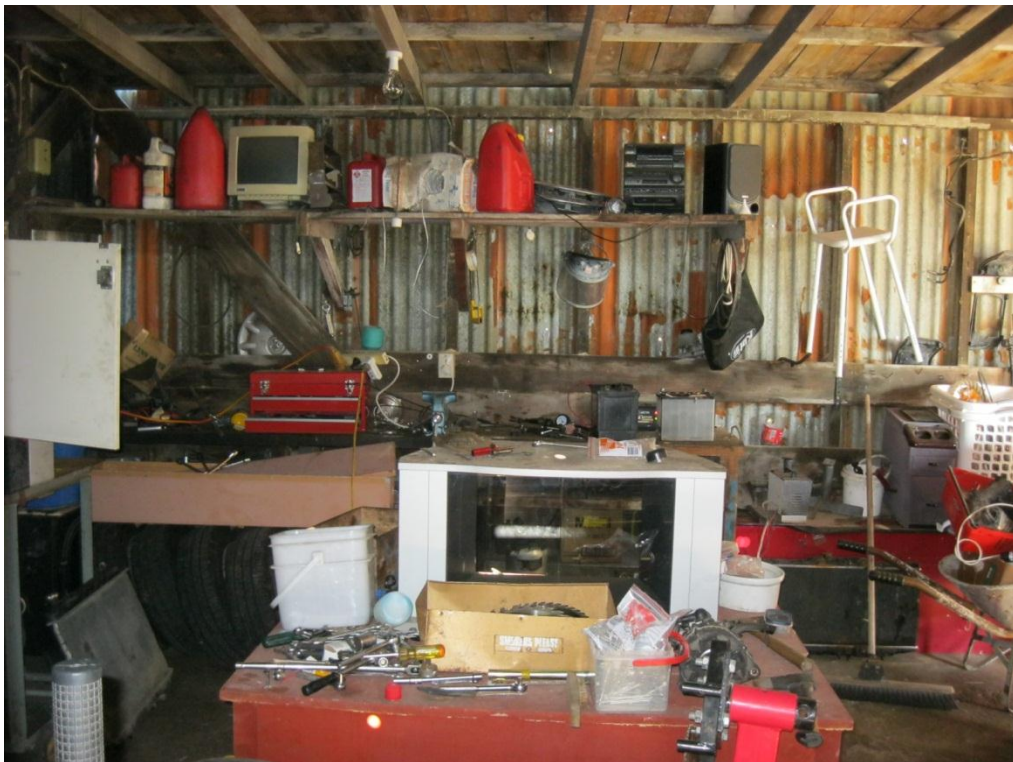
Photograph 8 Interior of the original portion of the building showing unbraced timber frame walls and roof.
