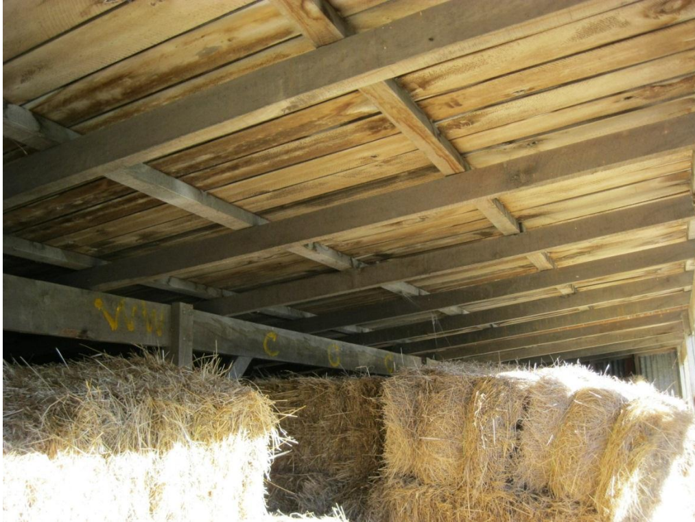
Photograph 7 Timber roof sarking on timber roof purlins on timber joists supported by the timber beam and post frame system.
