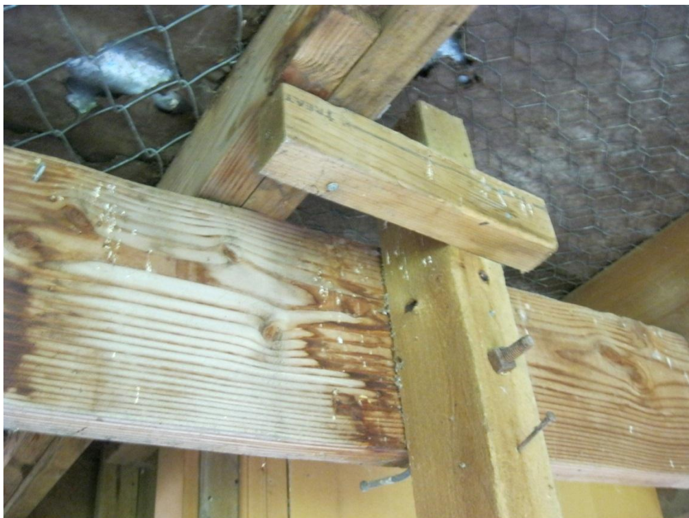
Photograph 5 Internal view of the split primary construction. View of the north wall.
