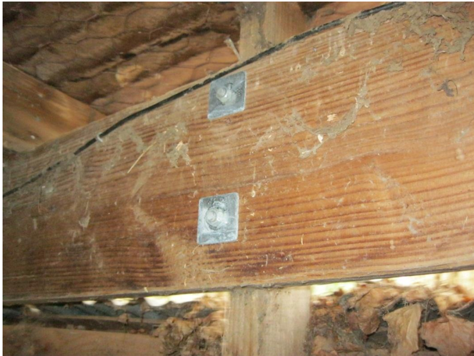
Photograph 7 A number of bolts provided to a connection.
