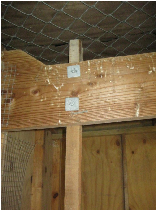
Photograph 9 Provision of bolts to the joint between rafters and timber post.
