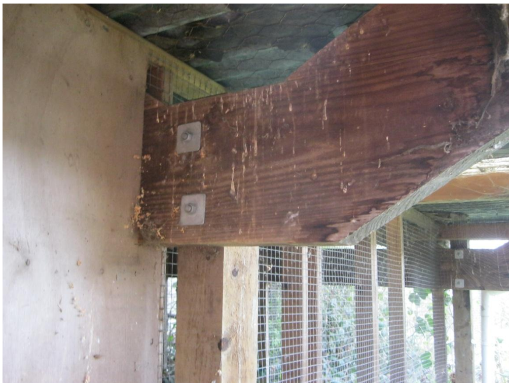
Photograph 8 Provision of bolts to the joint between rafters and timber post.
