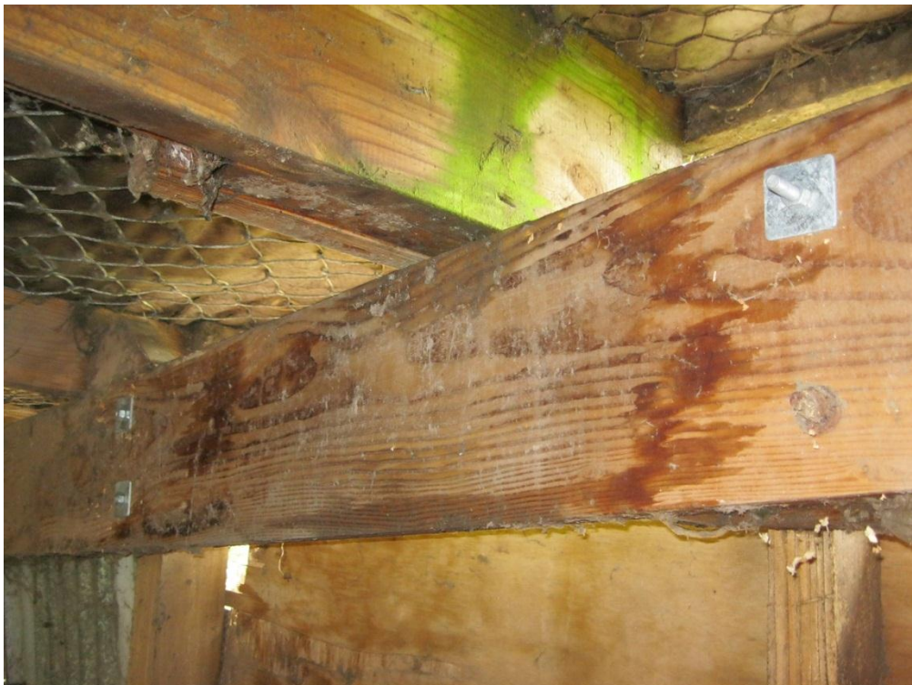
Photograph 10 Provision of bolts to the joint between rafters and timber post.
