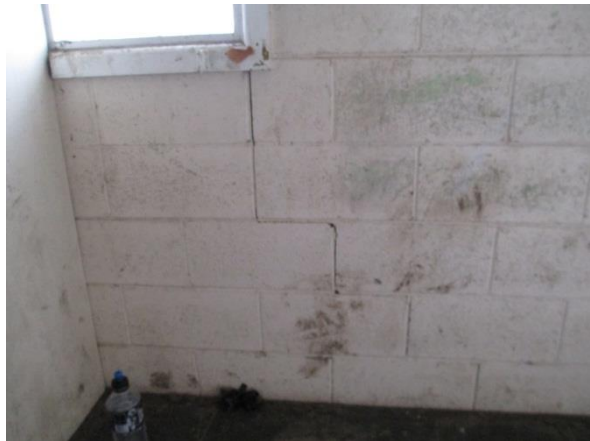
Minor step cracking in the blockwork under one of the windows
