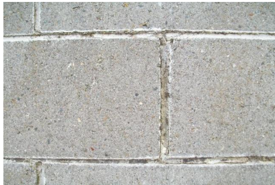
Photo 3: Typical stepped cracking in the block walls
