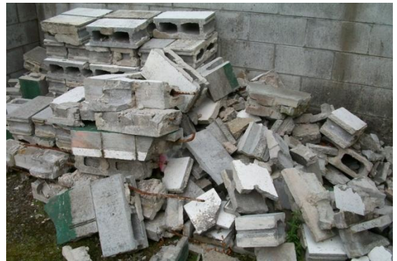
Photo 4: Rubble from the demolished wall showing partially filled and reinforced walls with poor compaction
