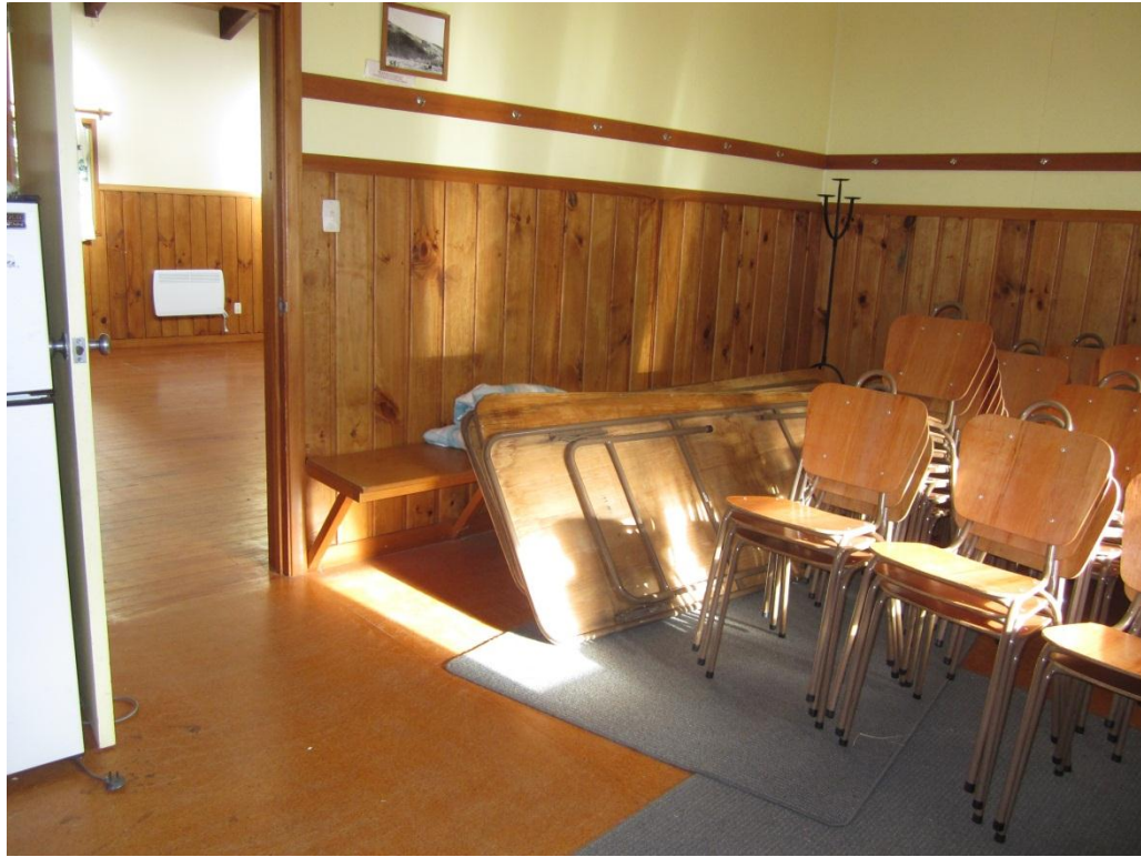
Photo 7. Timber board lining with plasterboard above.
