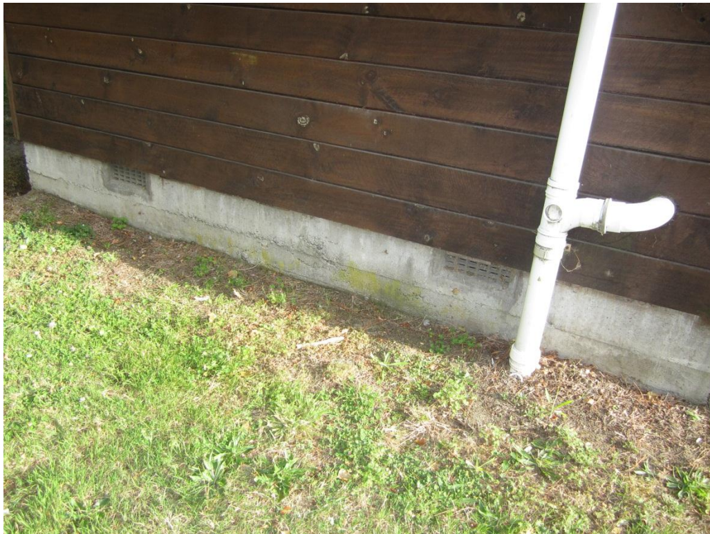
Photo 4. Concrete perimeter strip footing with weather boards above.
