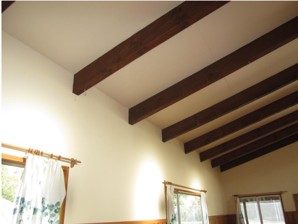
Photo 6. Timber rafters supporting roof structure.
