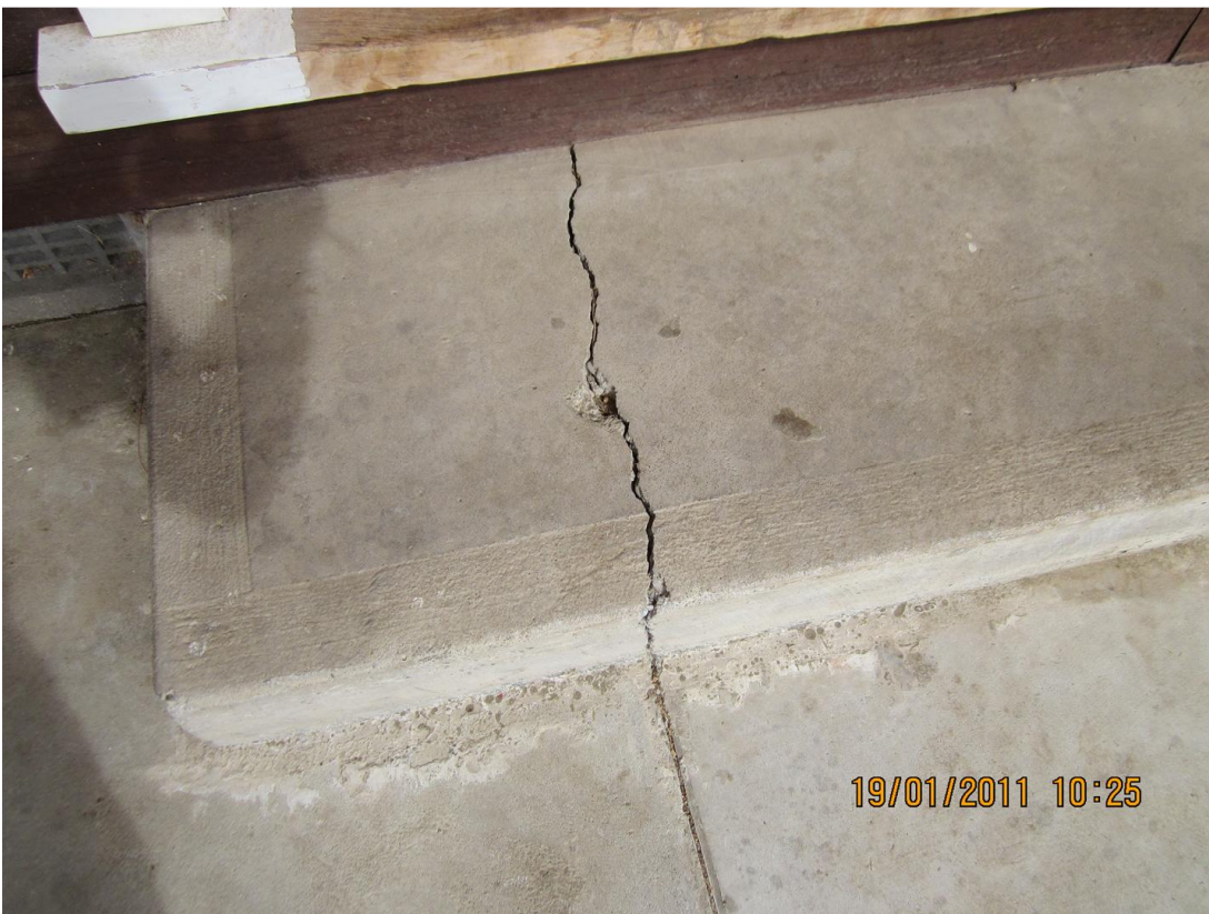
Photo 8: 5mm crack on step
