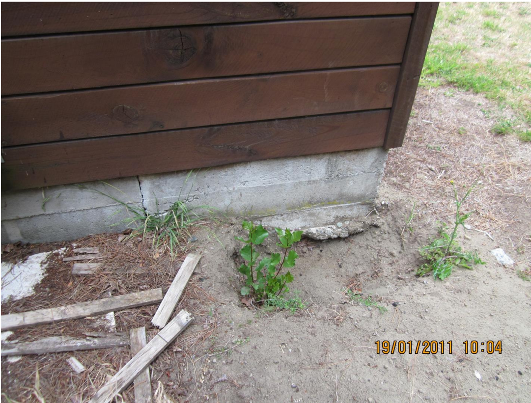
Photo 7: Undermined footing and cracks
