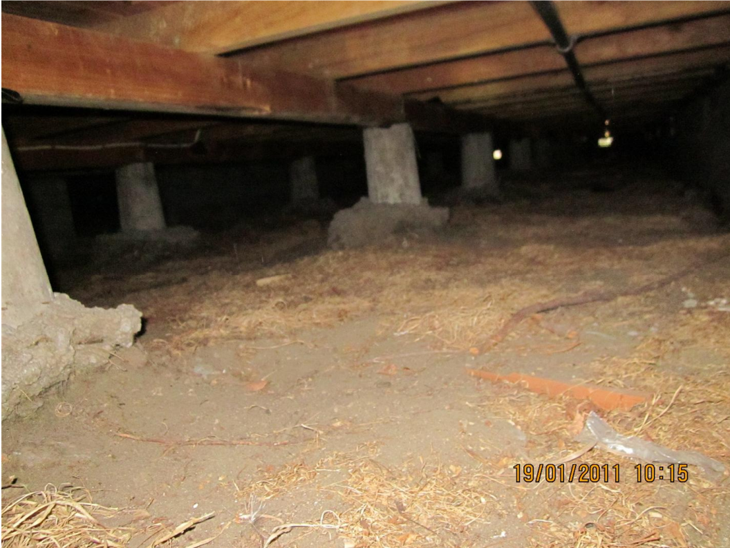
Photo 6 – View of the pile foundations and subfloor framing
