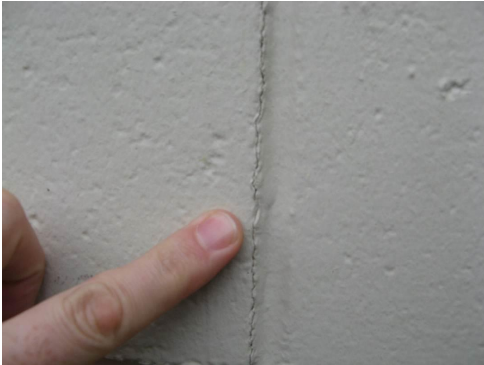
Photo 7: Cracking to concrete masonry wall (close up)
