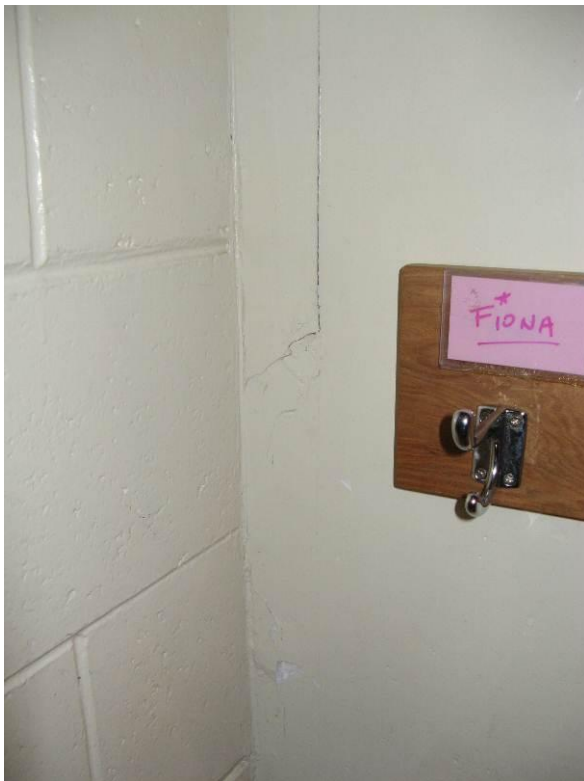
Photo 8: Joint between walls
