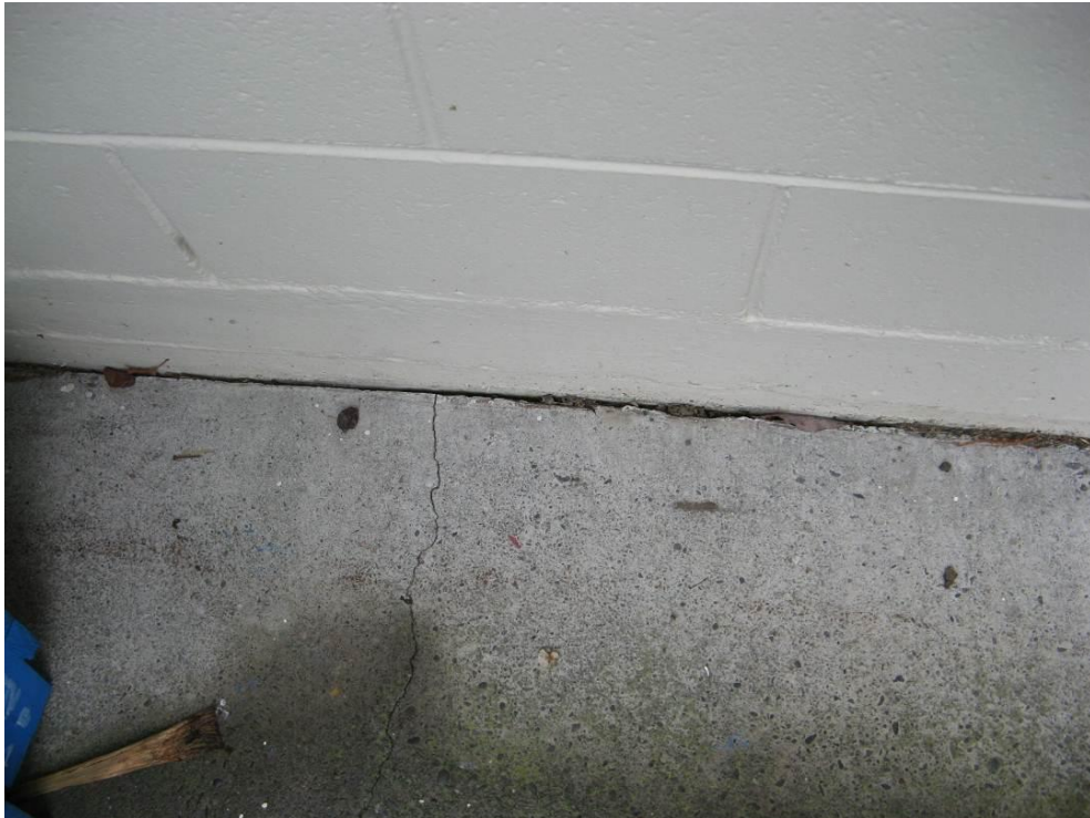
Photo 5: Cracking to concrete ground slab (west of building).
