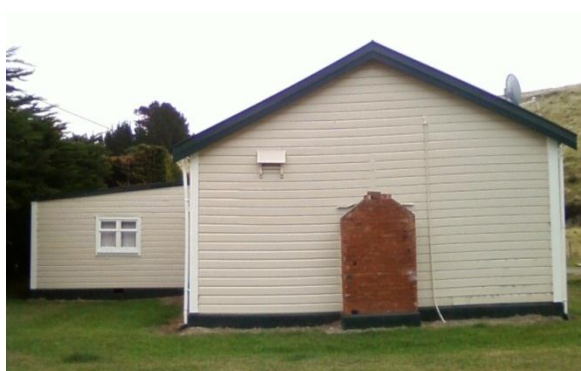
Southern elevation of Kaituna Hall. Note partial deconstruction of chimney.
