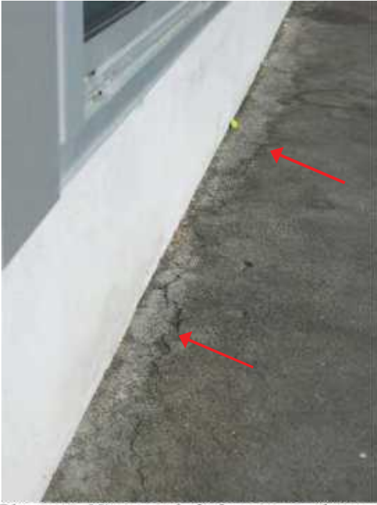
Photo 17: Minor asphalt damage on the north-west side of the Gym.
