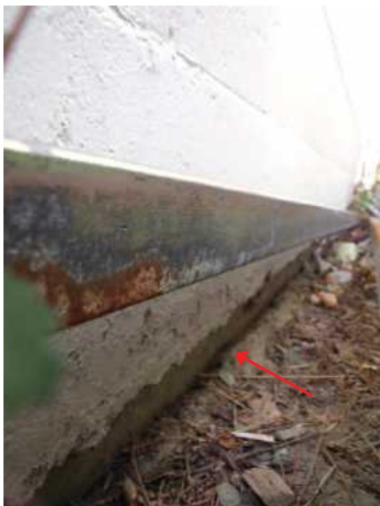
Photo 31: Possible settlement (20-30mm) of the asphalt on the north-western side of the Plant Room.
