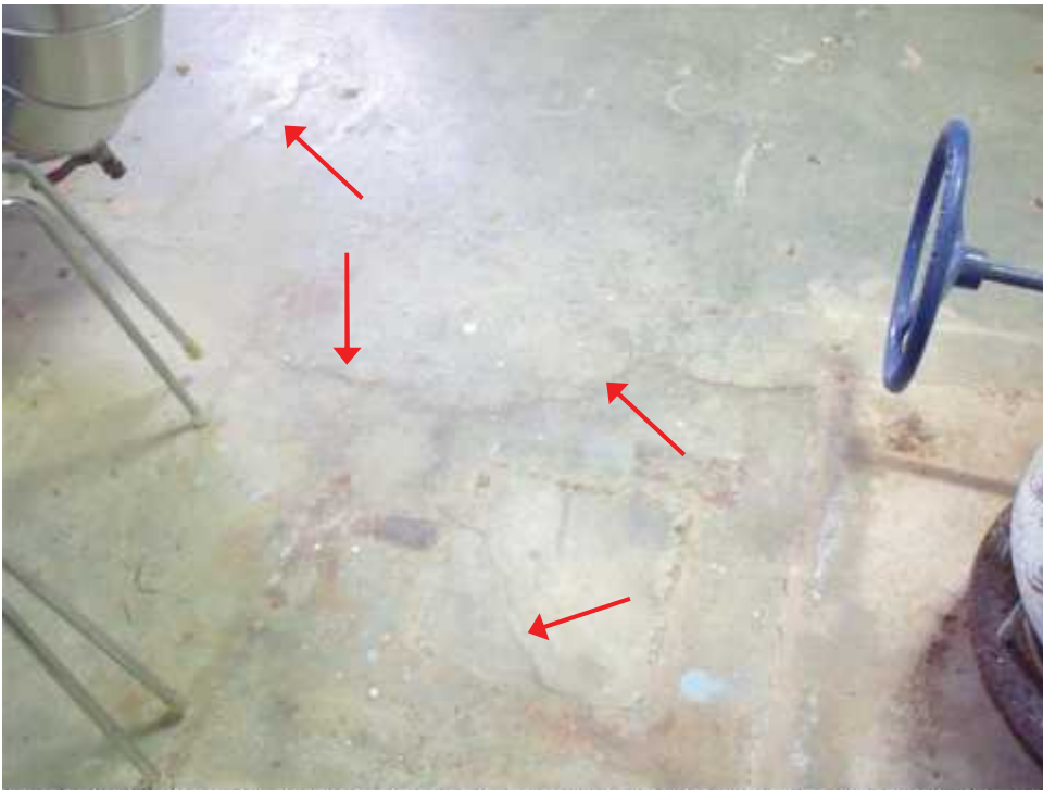
Photo 27: Minor crack (running north-west to south-east) in the floor slab of the Plant Room.
