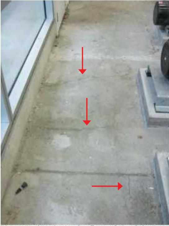
Photo 7: Cracks in the floor slab of the internal Plant Room 3.
