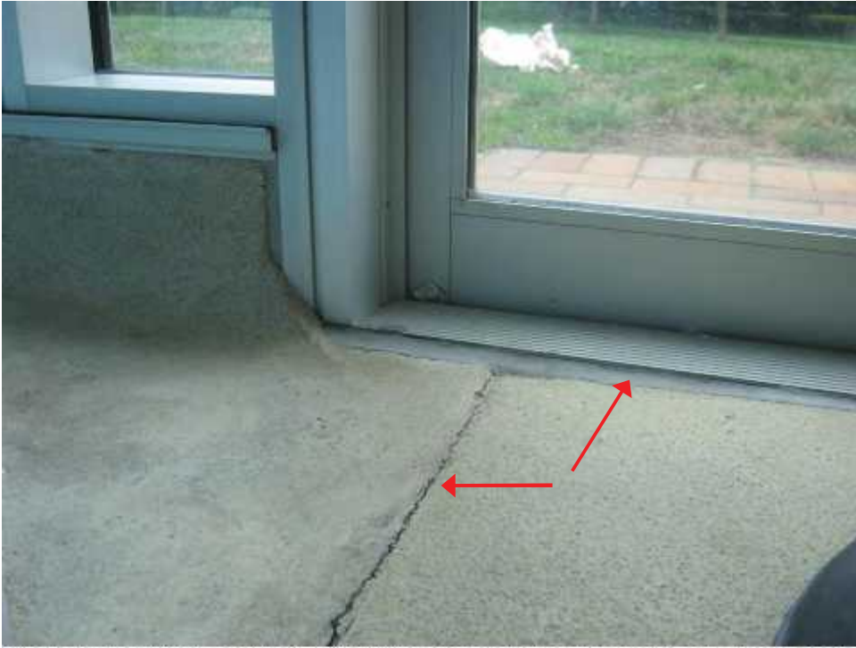
Photo 9: Possible settlement at the entrance to the Toddlers Pool. Note new seal at the base of external door frame.
