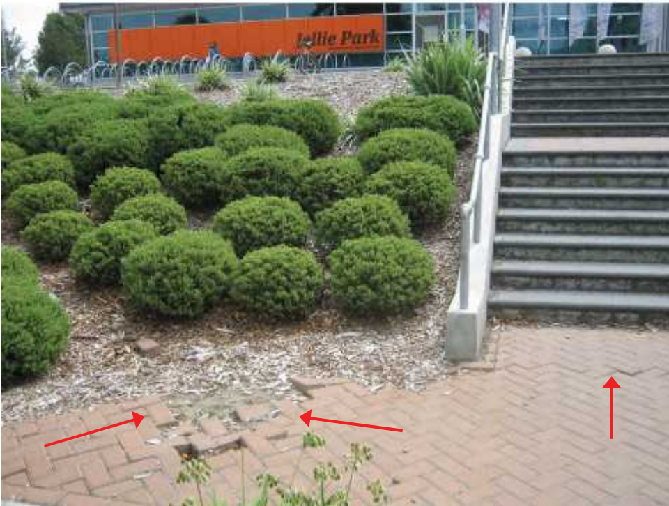
Photo 18: Sole location of liquefaction on site, 18m south-east of the main entrance to Jellie Park, less than 100mm of heave. Note the displacement of the bricks.
