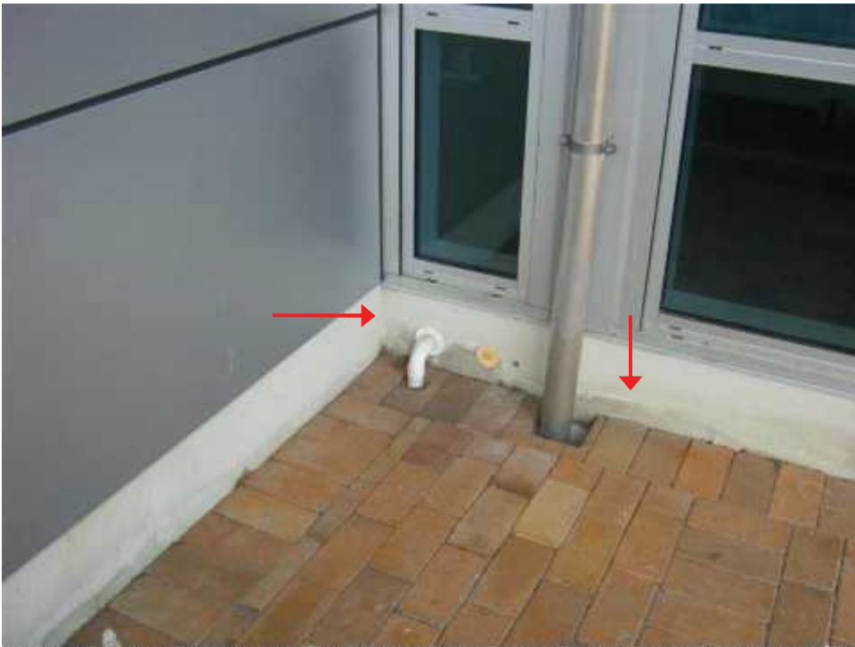
Photo 15: Minor vertical and horizontal cracking adjacent to the Gym and the Foyer, possible water damage.
