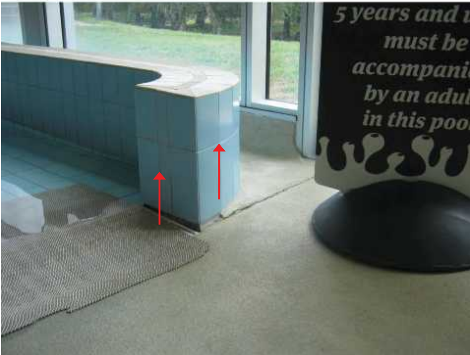
Photo 8: Possible settlement at the entrance to the Toddlers Pool, approximately 10mm to 15mm.
