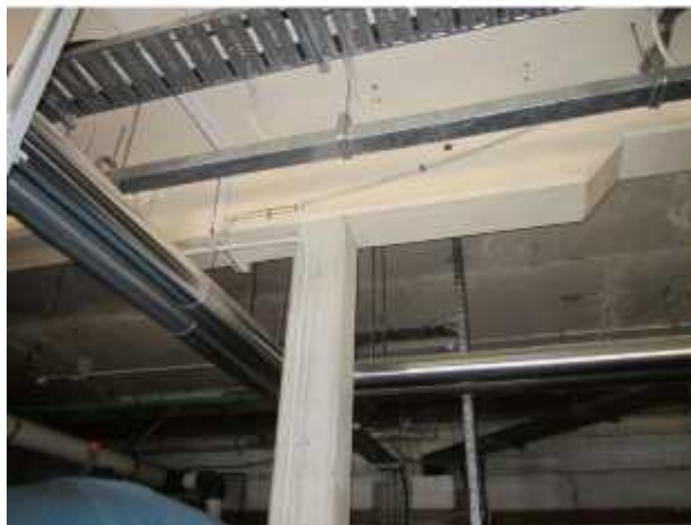
Photo 21 – Typical Interior Beam-Column Connection – plant room
