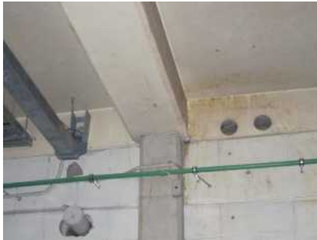
Photo 22 – Typical End Beam-Column Connection at Exterior Wall – plant room
