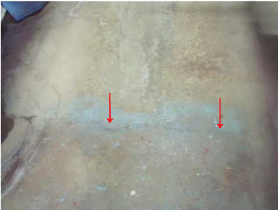
Photo 26: Minor crack (running north-west to south-east) in floor slab of Plant Room.
