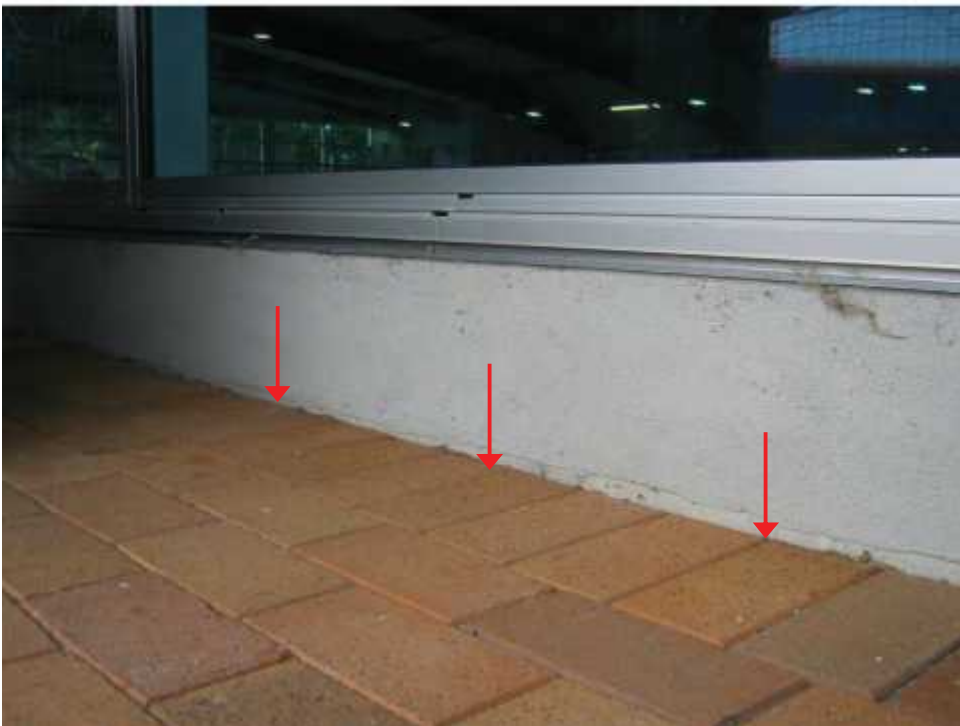
Photo 14: Horizontal crack in perimeter strip footing, north-west wall of the New Pool Hall.
