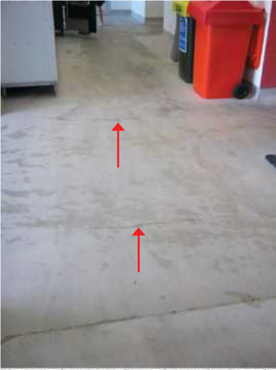
Photo 3: Cracks in floor slab in the foyer leading into the pool complex.
