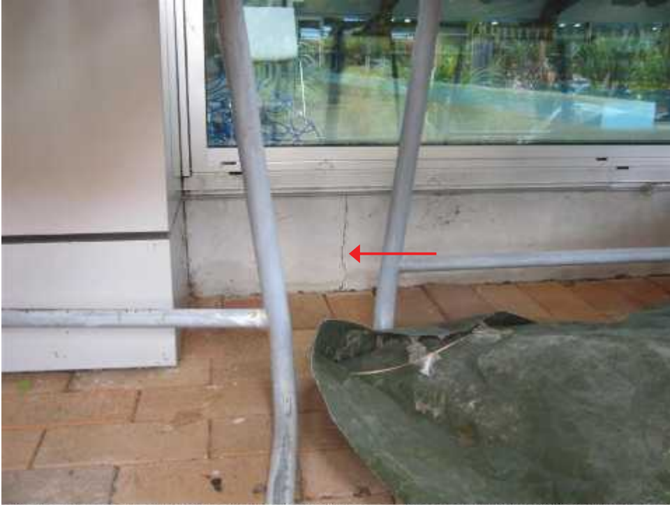
Photo 11: Crack in perimeter strip footing, north-west wall of the New Pool Hall.
