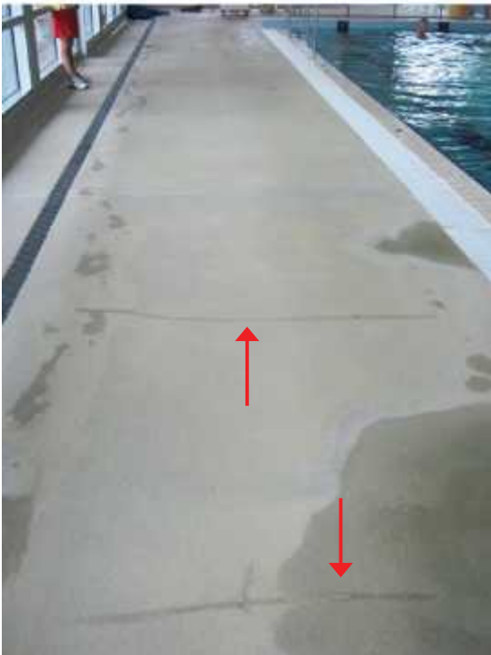
Photo 6: Cracks in floor slab in the New Pool Hall, looking north-east.
