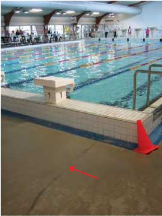
Photo 5: Crack in floor slab in the Old Pool Hall, looking north.
