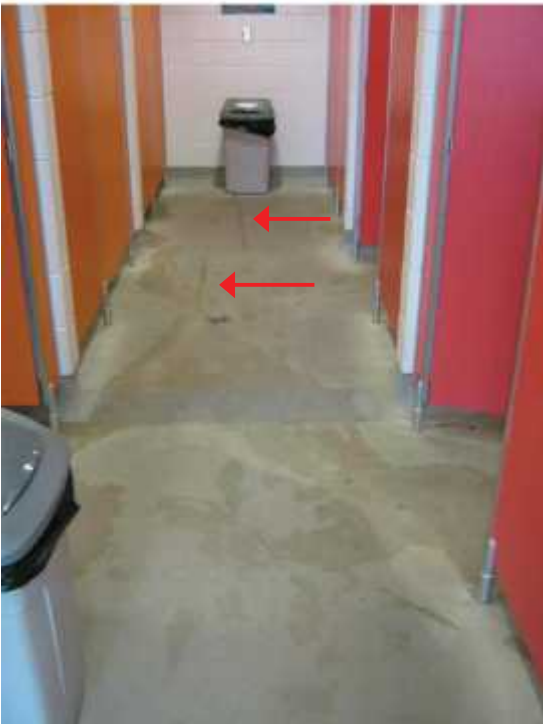
Photo 4: Cracks in floor slab in the Family Changing Rooms.
