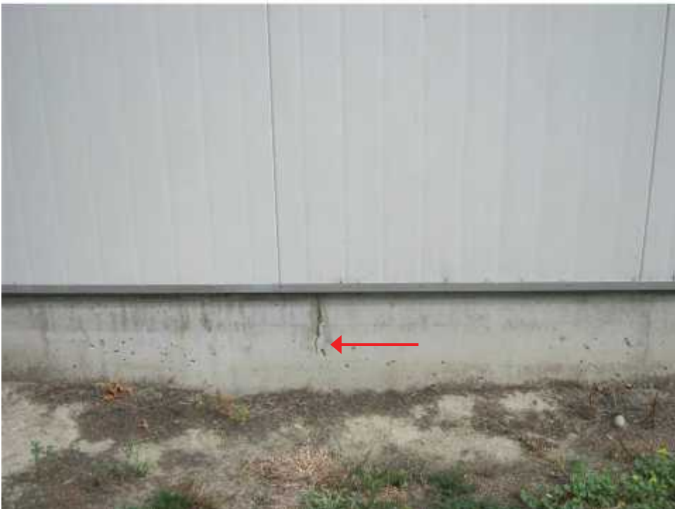
Photo 12: Crack in perimeter strip footing, northern side of Internal Plant Room 3.
