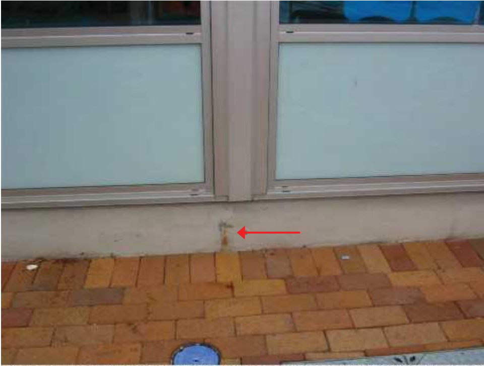
Photo 13: Crack in perimeter strip footing, north-west wall of the New Pool Hall.
