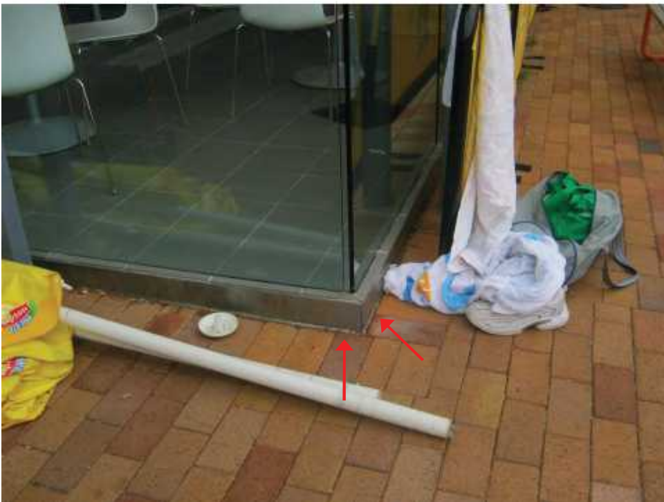
Photo 16: Minor settlement, approximately 10-15mm, between brick and tiled area outside of the cafe in the Foyer.
