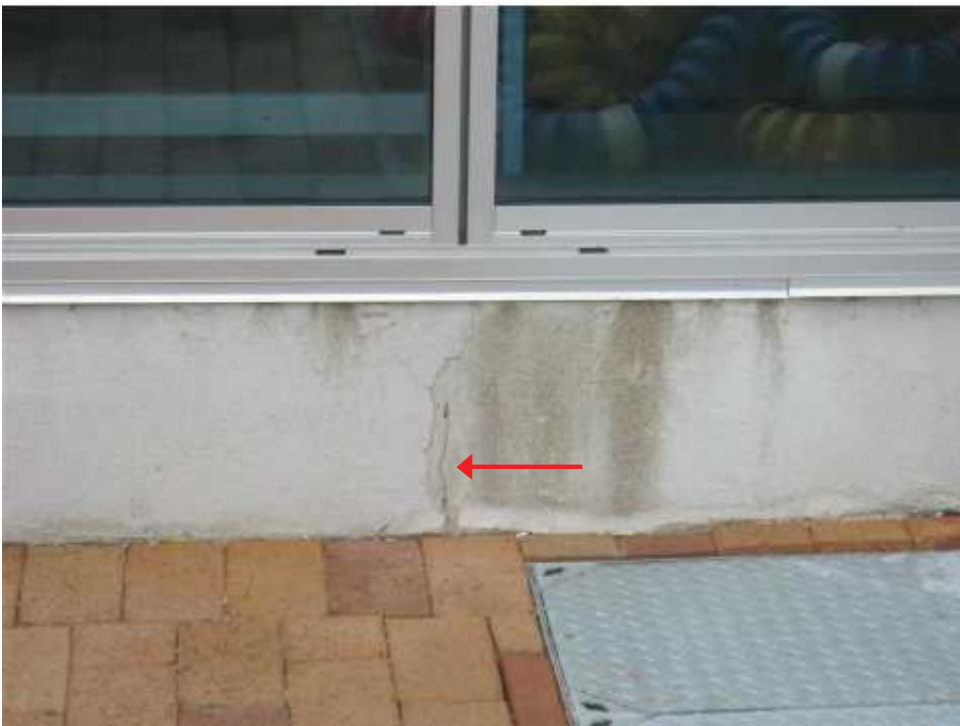
Photo 10: Cracking and spalling of concrete in the perimeter strip footing, north-west wall of the Spa Area.
