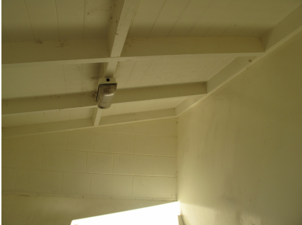
Photograph 7 Timber beams and purlins.
