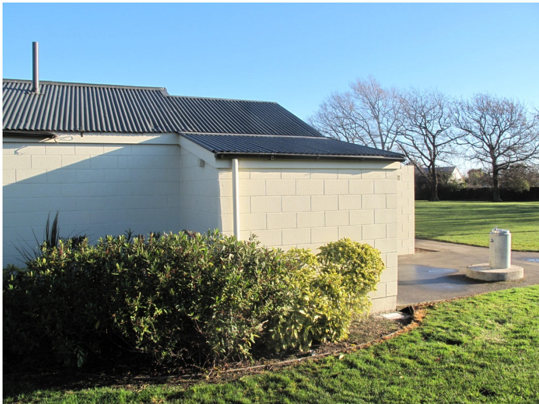
Photograph 2 View of the toilet block from the southeast
