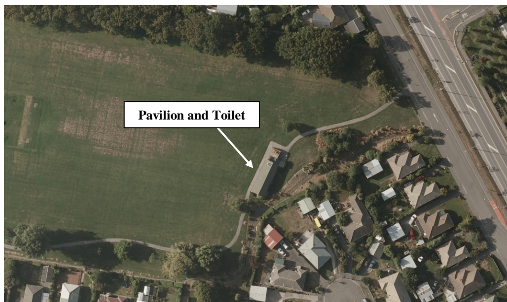
Figure 2 Post February 2011 Earthquake Aerial Photography 3
