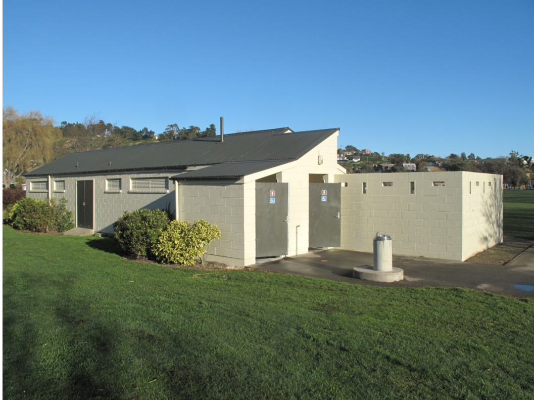
Photograph 3 View of the toilet block from the northeast.
