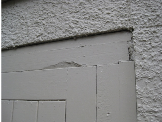
Photo 9: Existing impact damage to timber doorframe on the north side.
