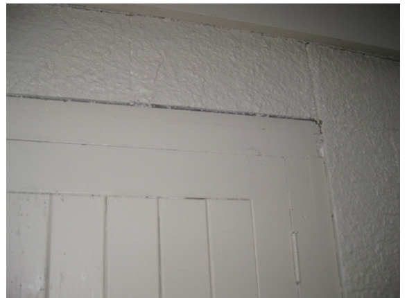
Photo 8: Gaps opening up between timber elements in the doorframe on the north side.
