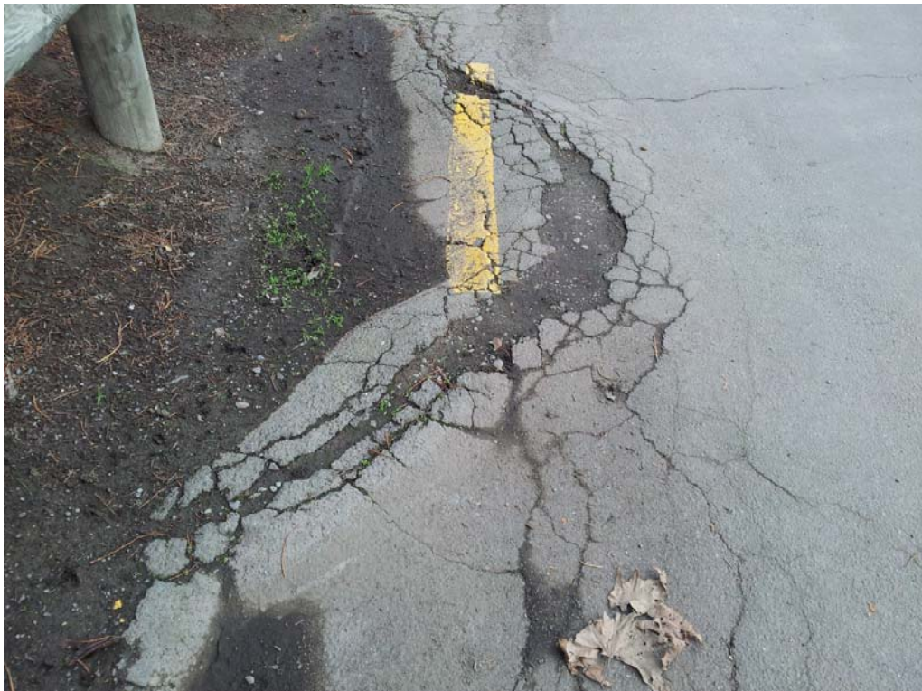
■ Figure 10– Observed ground bulges
