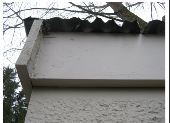
Photo 16: Gap opening up between masonry wall and timber roof edge beam on south side.
