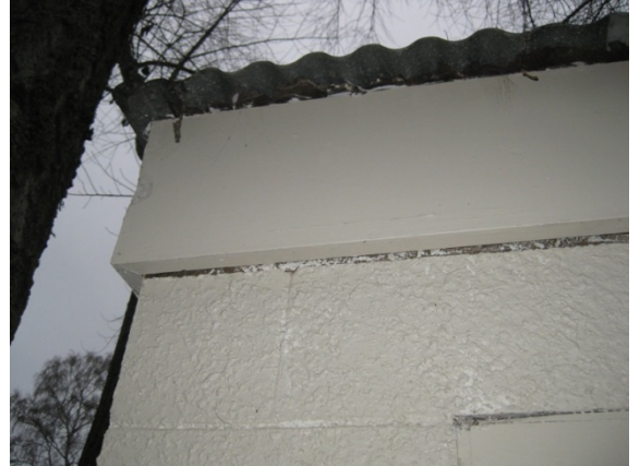
Photo 6: Gap opening up between masonry wall and timber roof edge beam on north side.
