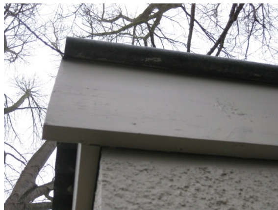
Photo 19: Gap opening up between masonry wall and timber roof edge beam on east side.
