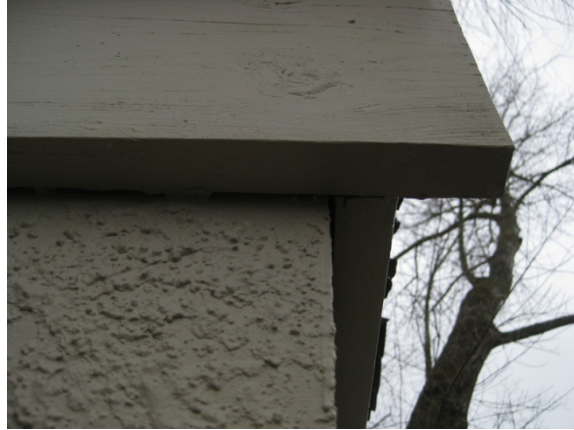
Photo 13: Gap opening up between masonry wall and timber roof edge beam on west side.
