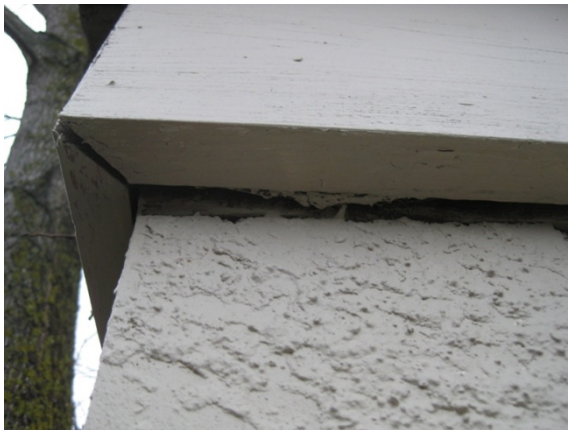
Photo 11: Gaps opening up between masonry wall and timber roof edge beam on northwest side.
