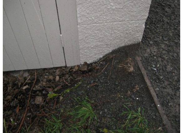
Photo 10: Level of the path is one block higher than the ground level at the entrance to the pumphouse on the north side.
