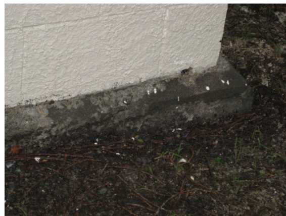
Photo 15: Concrete slab footing exposed on southwest corner.
