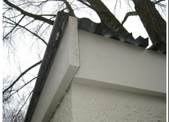
Photo 14: Overhang of 250 x 30 timber roof edge beam.
