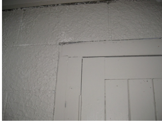
Photo 5: Gaps opening up between timber elements in the doorframe on the north side.
