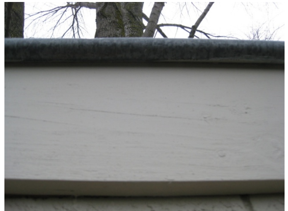
Photo 12: Longitudinal cracking on timber roof edge beam on west side.
