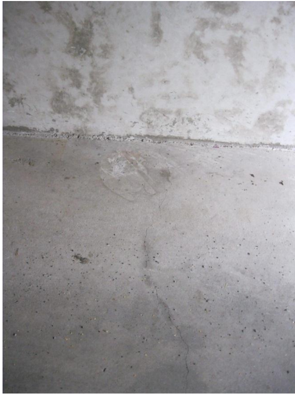
Photo 5. Minor cracking in reinforced concrete ground slab.
