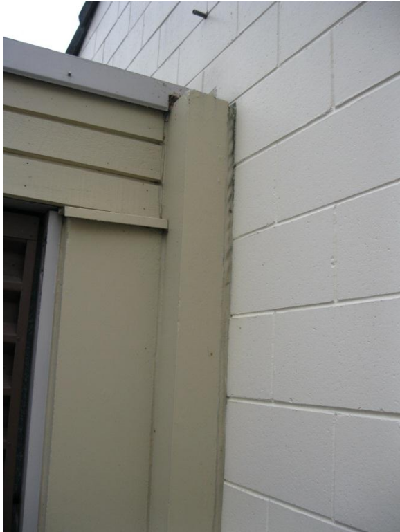
Photo 6. Flexible Filler between garage and gable wall of Block F.
