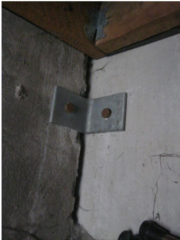
Photo 4. Cleat connection between rear and partition walls.
