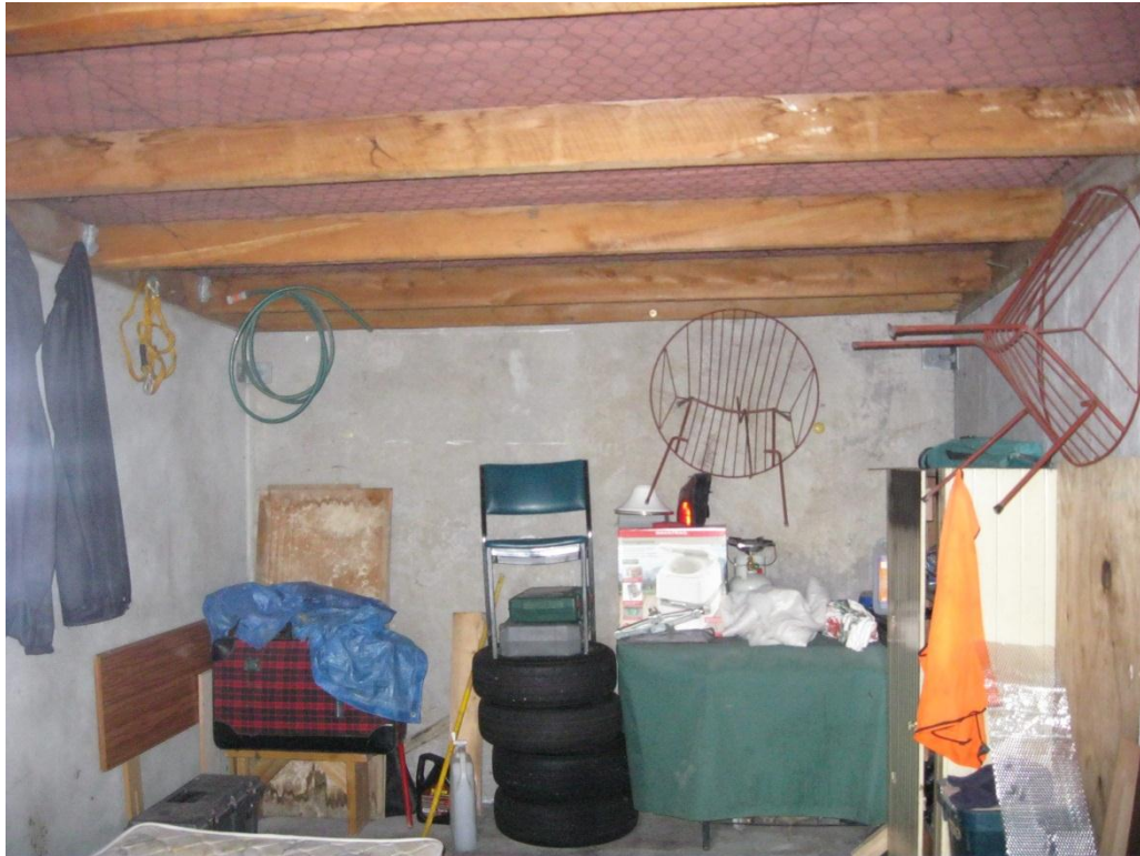
Photo 6. Roof joists spanning between partition walls.
