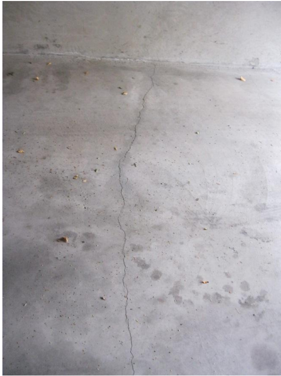
Photo 5. Minor cracking in reinforced concrete ground slab.
