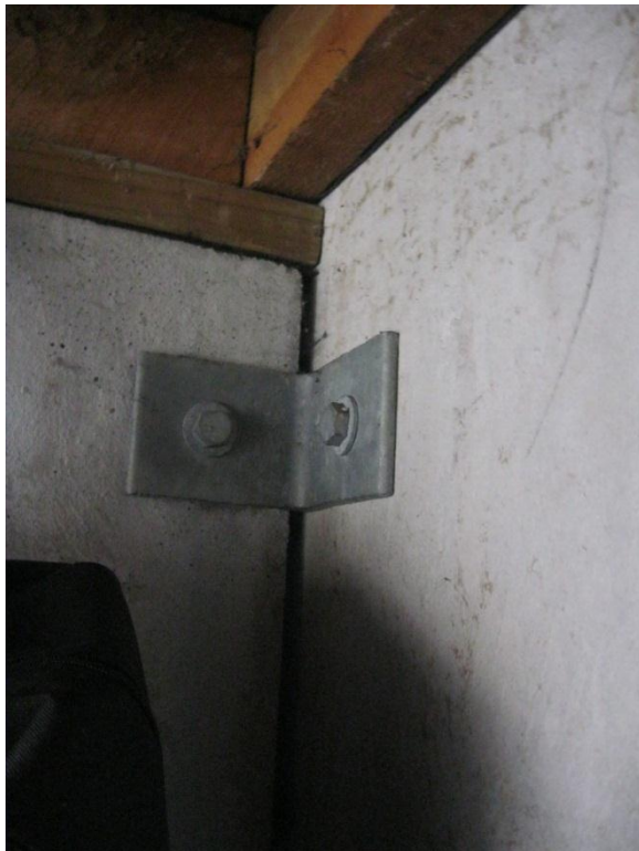
Photo 4. Cleat connection between rear and partition walls.
