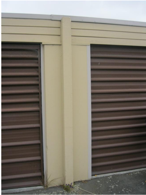
Photo 3. Minimal piers along garage door elevation.
