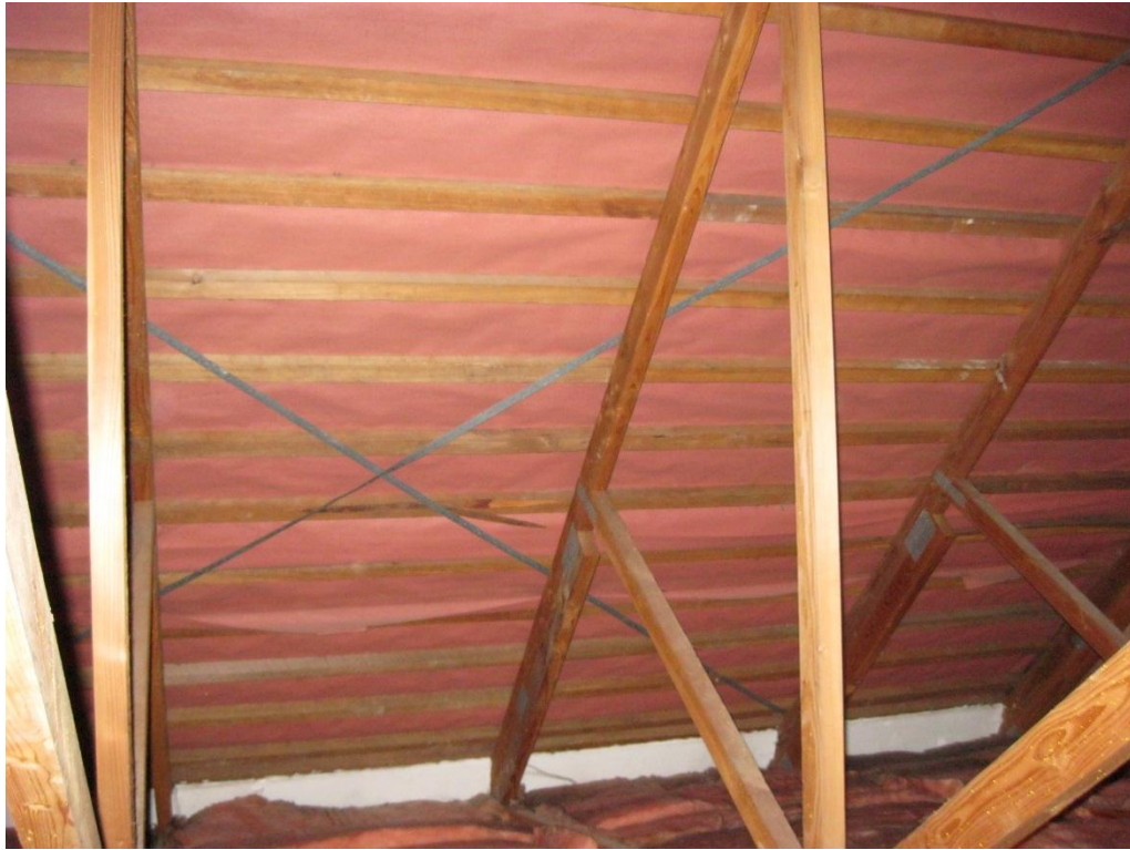
Photograph 11 Flat steel strap roof cross bracing.
