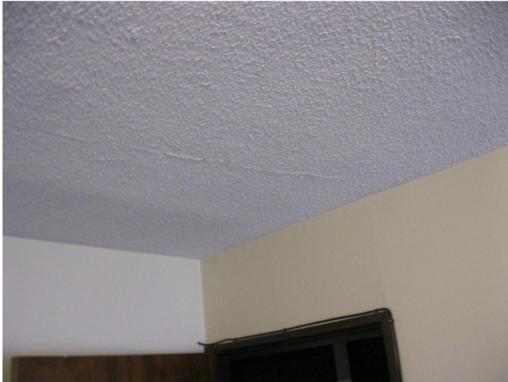
Photograph 3 Cracking to plaster finish on the underside of the suspended floor slab.
