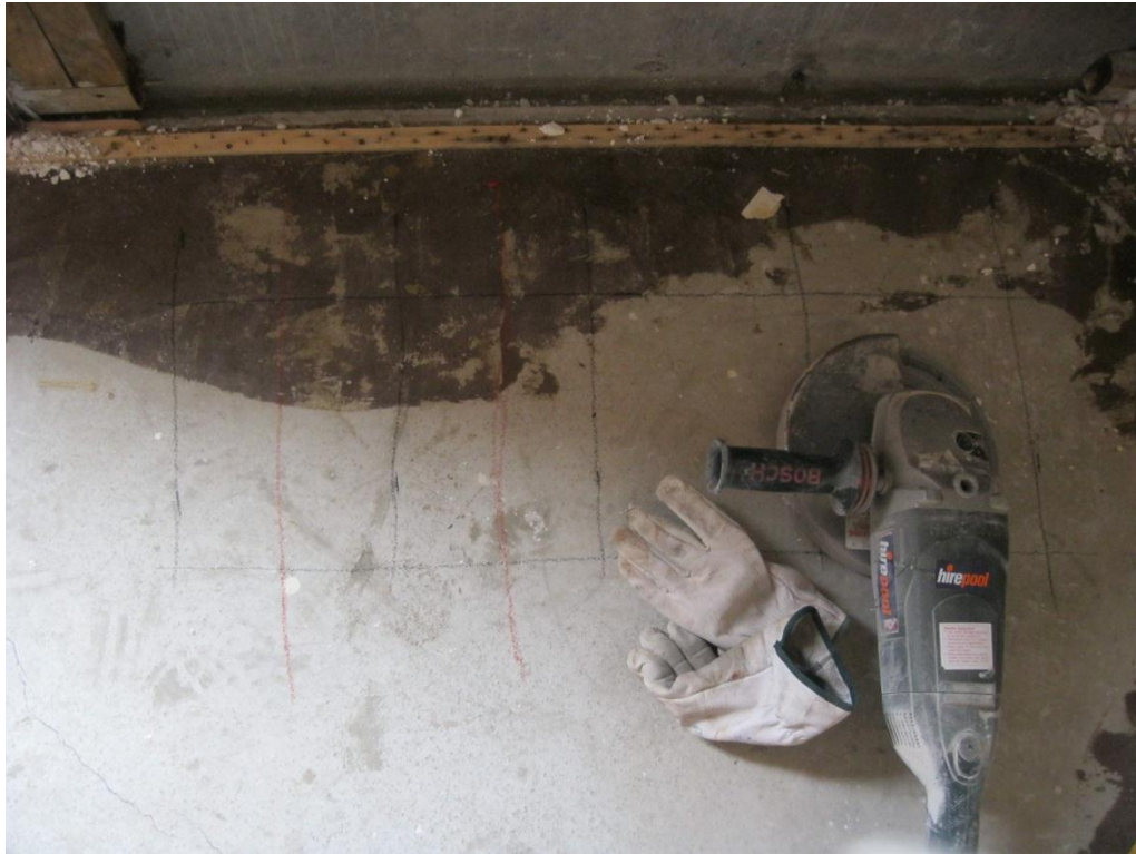
Photograph 19 Black lines indicating where reinforcement is expected to be found and red lines indicating area to be exposed.
