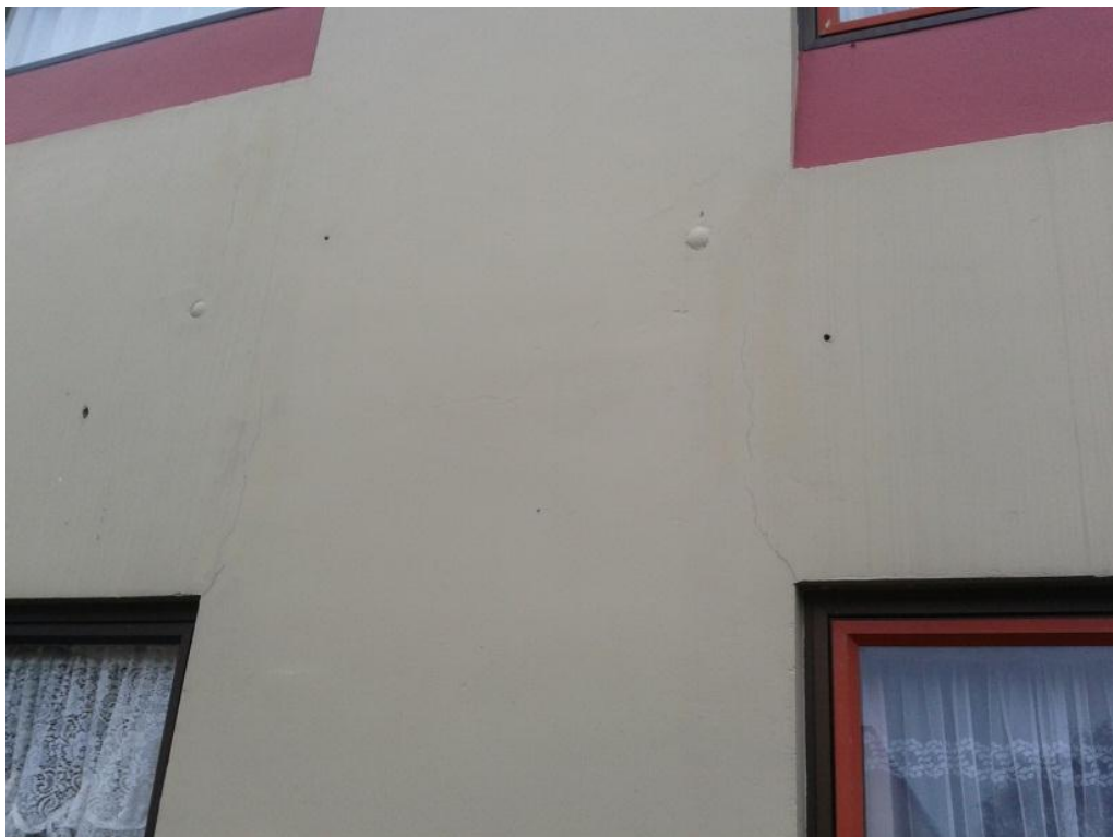
Photograph 2 Cracking to exterior walls at window corners.
