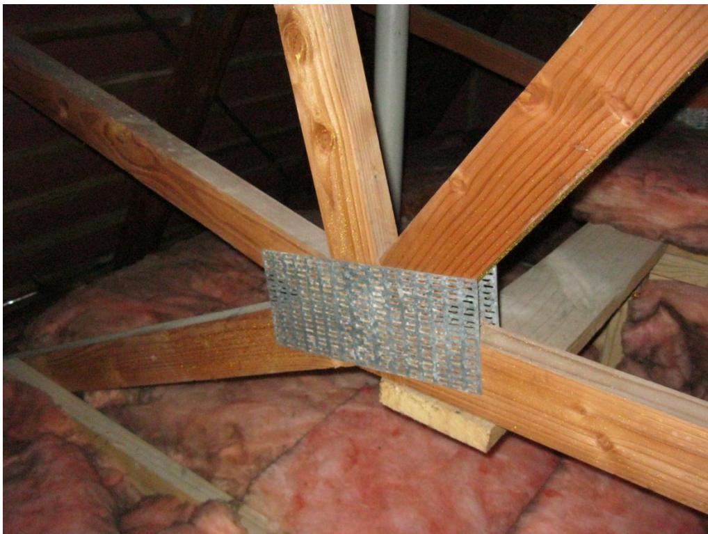
Photograph 10 Connection of timber roof truss members.
