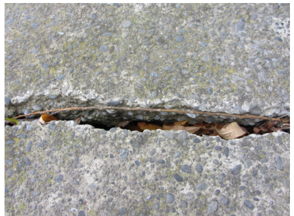
Photo 8: Close up view of cracking in pavement from photo 7
