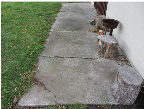
Photo 7: Cracking in pavement
