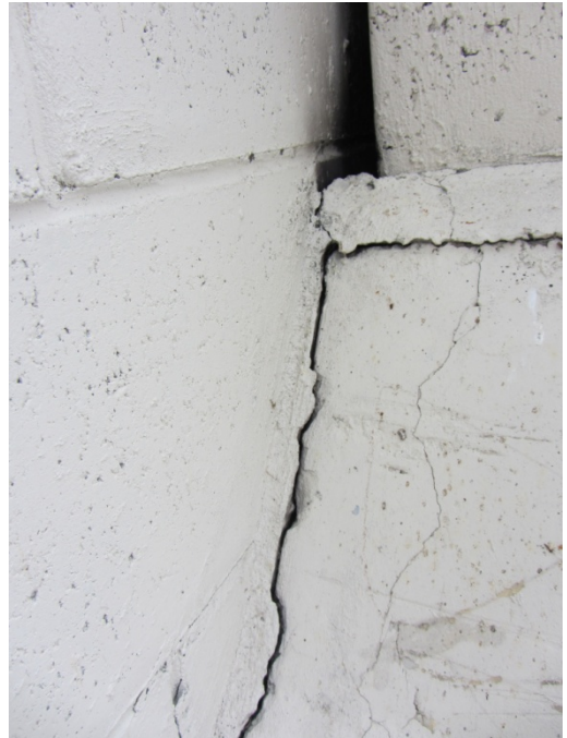
Photo 10: Close view of 1.5mm crack between chimney and main structure
