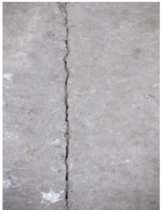
Photo 12: Close up view of 1.5mm interior floor slab crack
