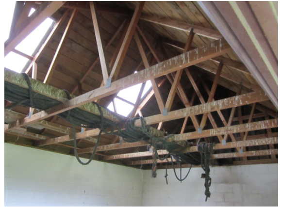
Photo 6: Interior view of the building showing the timber roof trusses
