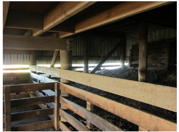
Photo 14: View of subfloor showing subfloor bracing in south east corner of building (1)
