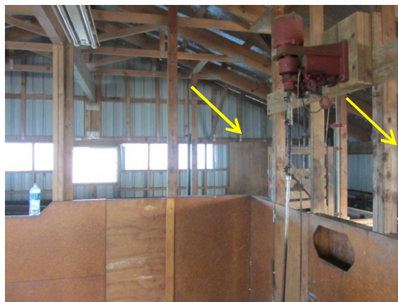
Photo 11: Interior view of Wool Shed showing plywood bracing in south west corner of building
