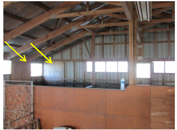
Photo 10: Interior view of Wool Shed showing plywood bracing in north west corner of building
