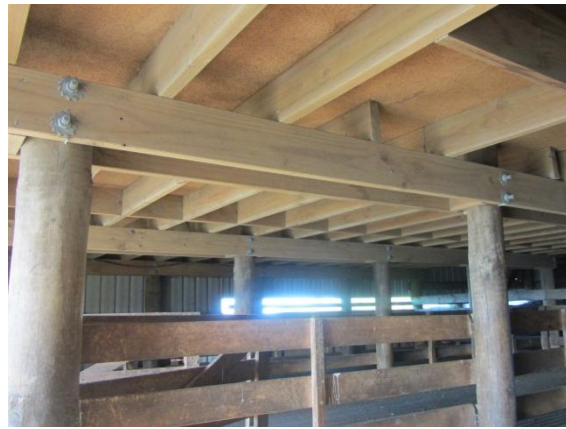
Photo 13: View of subfloor showing floor structure
