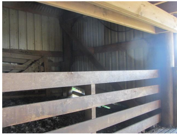
Photo 17: View of subfloor showing subfloor bracing in north west corner of building
