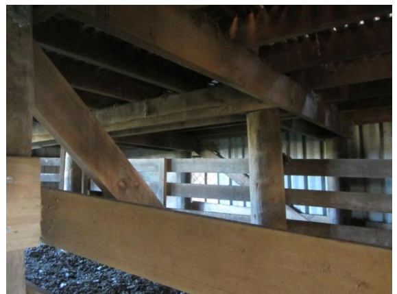
Photo 16: View of subfloor showing subfloor bracing in south west corner of building
