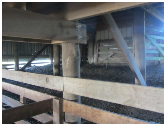
Photo 15: View of subfloor showing subfloor bracing in south east corner of building (2)
