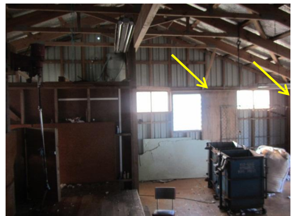
Photo 12: Interior view of Wool Shed showing plywood bracing in north east corner of building
