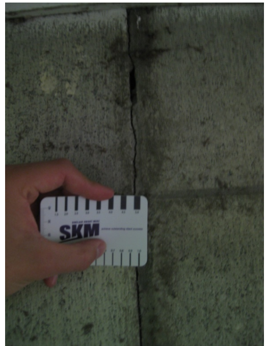
Photo 8: Close up from photo 7 showing 1mm crack between junction
