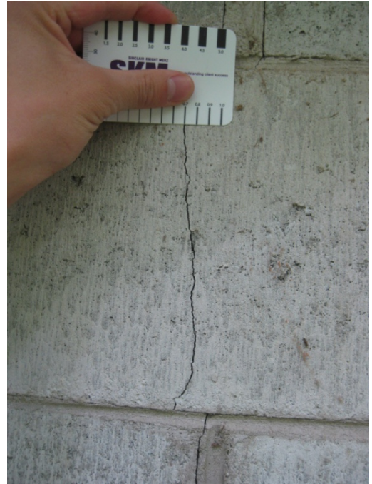
Photo 14: Close up of north wall showing 0.7mm vertical crack
