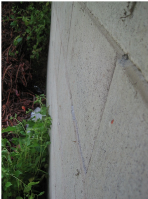
Photo 11: View of west wall showing displaced blocks
