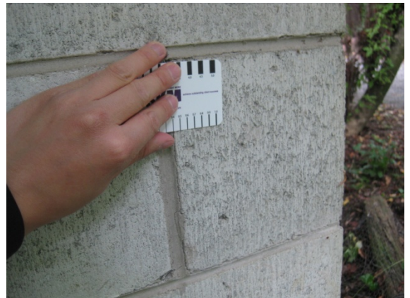
Photo 20: Close up view of photo 19 showing 0.4mm crack
