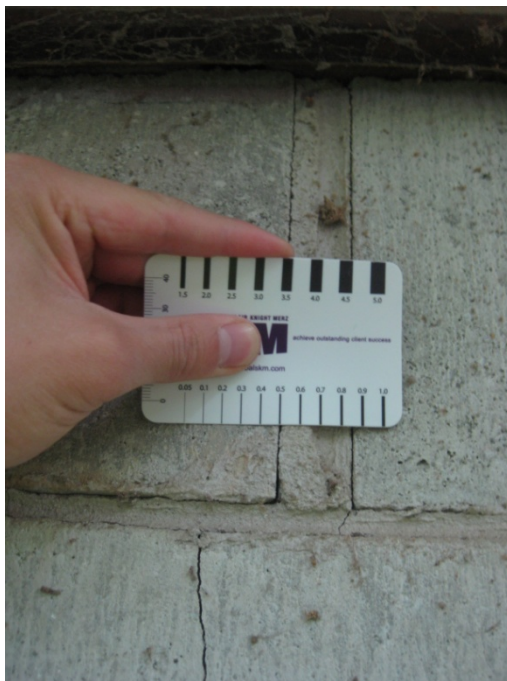
Photo 15: 0.5mm vertical crack at masonry block joint
