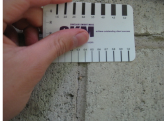
Photo 10: Close up view from photo 9 showing 0.3mm crack
