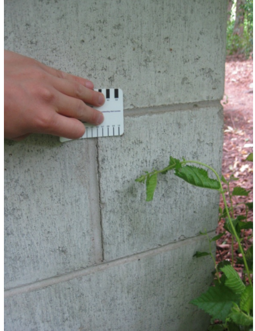
Photo 18: Close up view from photo 16 showing 0.6mm crack.
