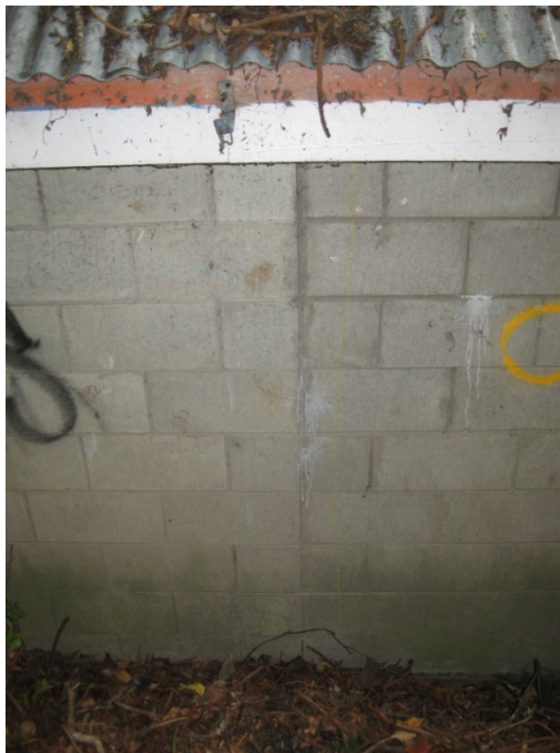
Photo 7: West wall, with junction between unreinforced wall and reinforced wall
