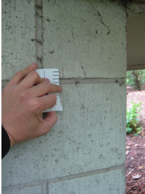
Photo 17: Close up view from photo 16 showing 0.8mm crack at top block course
