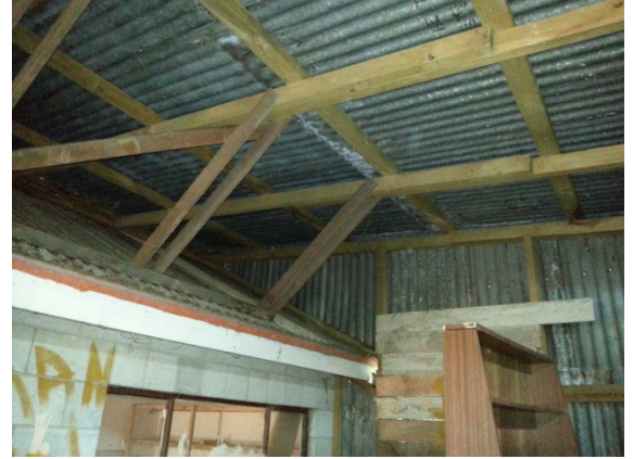
Photo 32: Roof frame of timber framed addition
