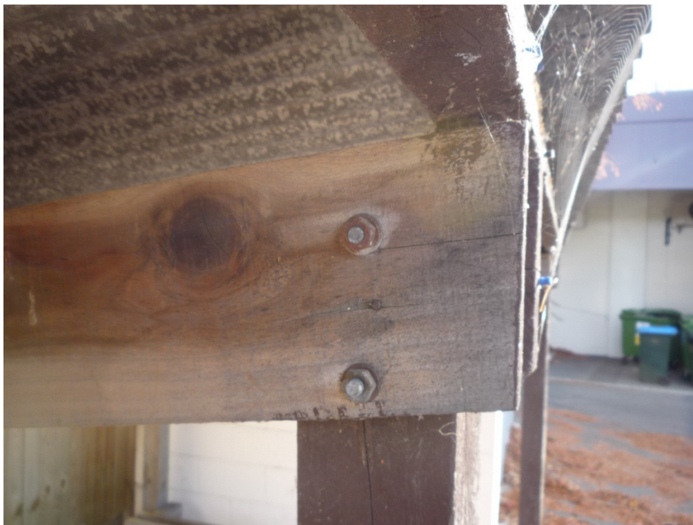
Photo 2: View of the beam column joint.
