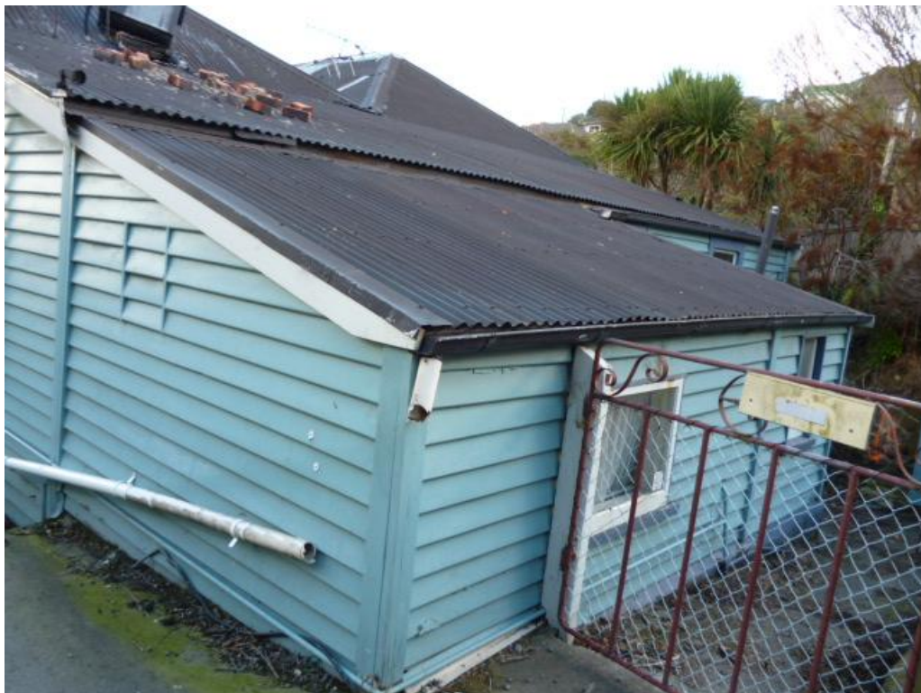
Photograph 4 Southern elevation and collapsed chimney.
