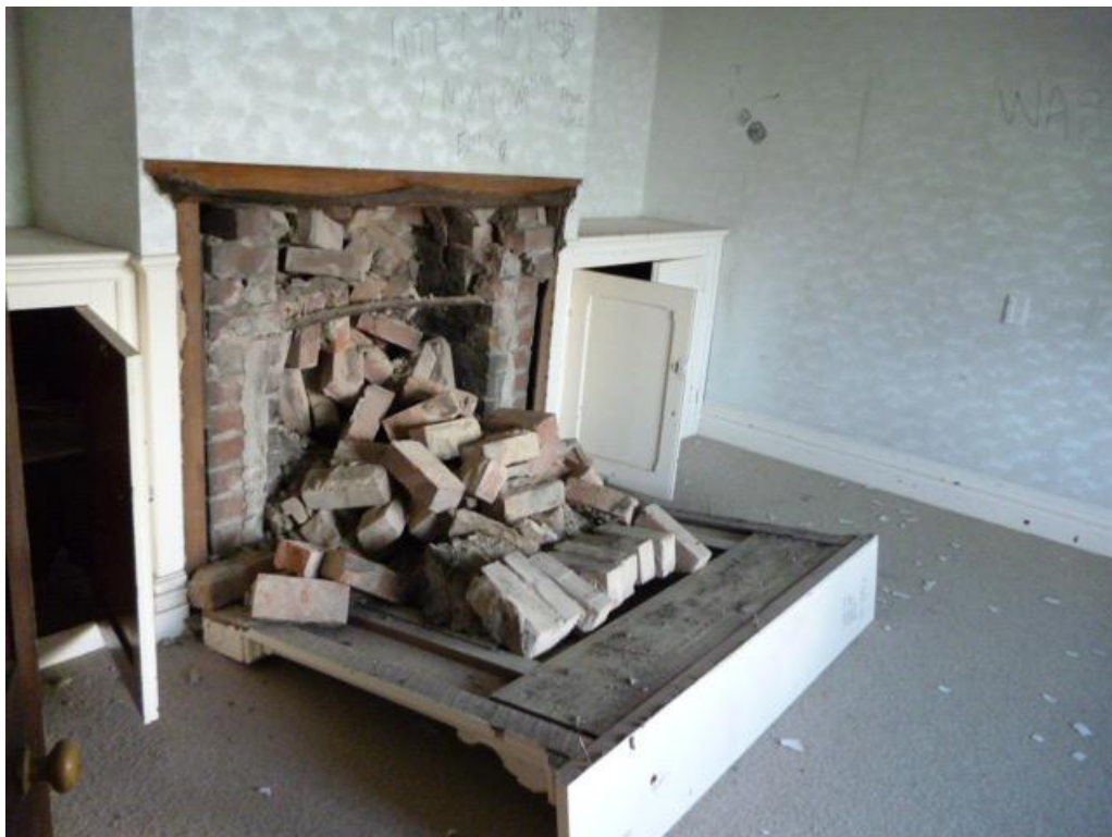
Photograph 6 Collapsed fireplace mantel.
