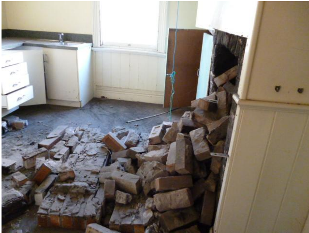
Photograph 9 Kitchen and collapsed chimney and fireplace
