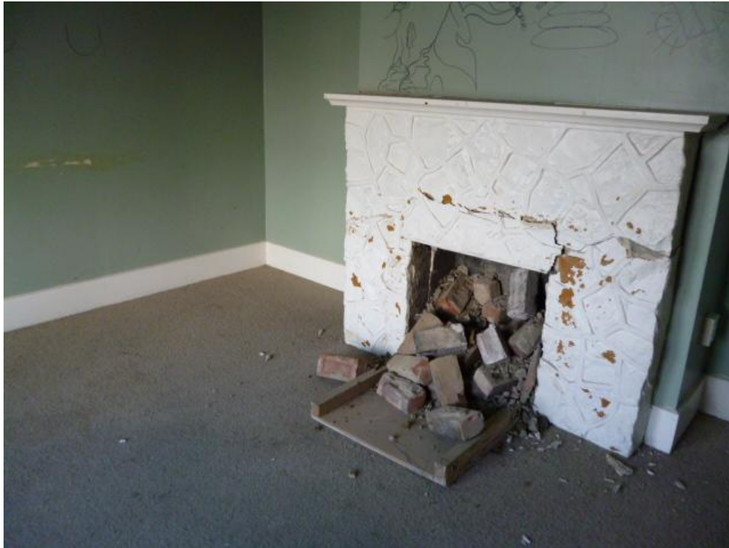
Photograph 7 Collapsed fireplace mantel.
