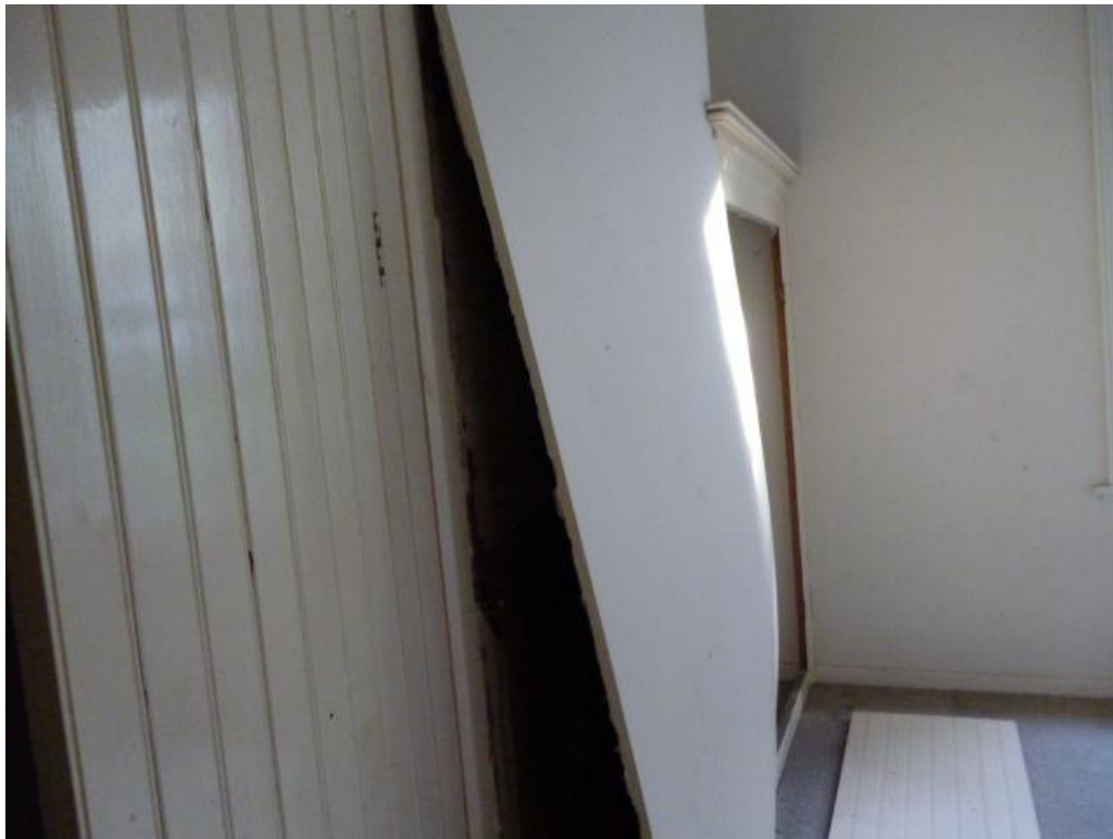
Photograph 11 Displaced plasterboard
