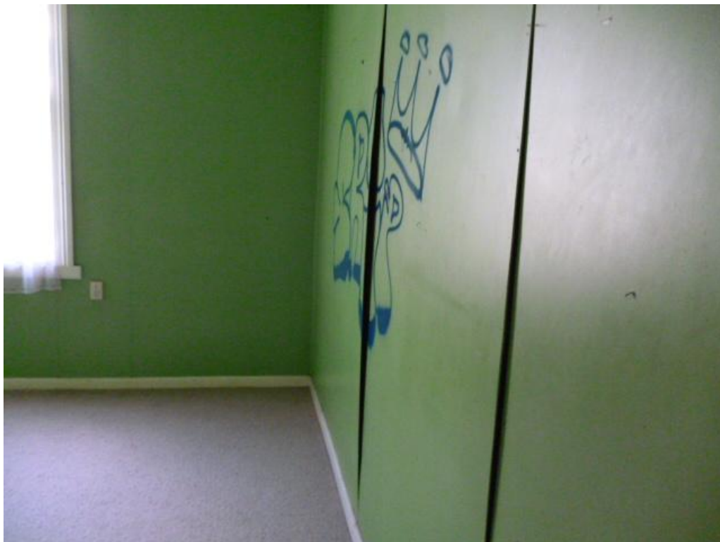
Photograph 8 Displaced plasterboard.
