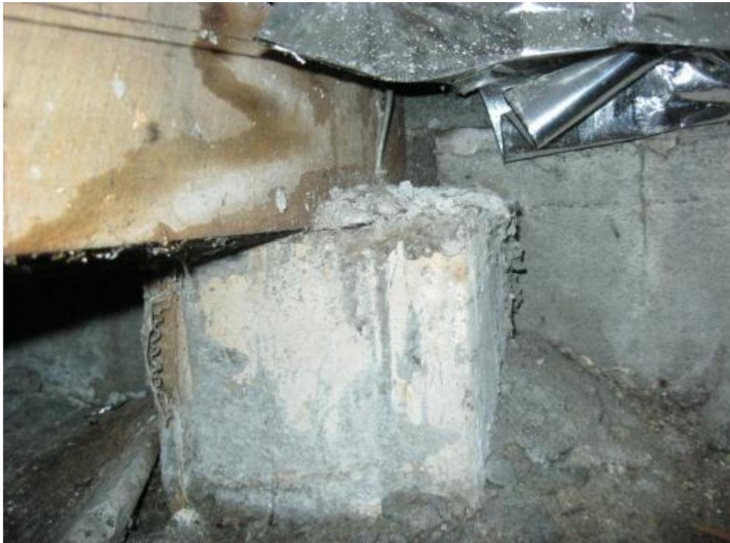
**Photograph 7 Timber bearer supported by concrete pile.**
