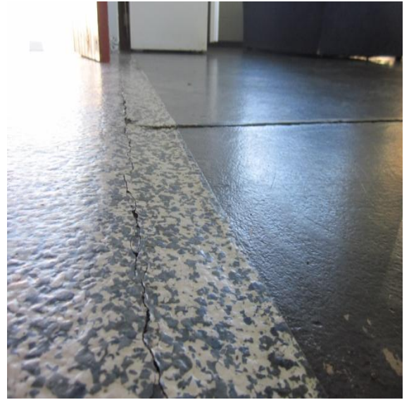
Photo 2: Separation and differential settlement between slab sections in the kitchen/living
