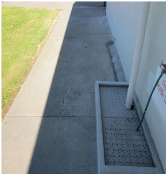
Photo 19: The external concrete path on the east side of the building showing typical differential settlement
