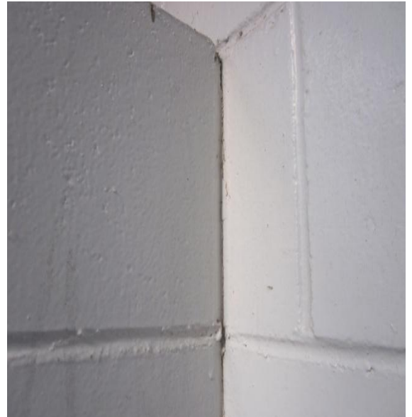
Photo 14: Typical hairline separation between the 2m high internal walls and the perpendicular walls
