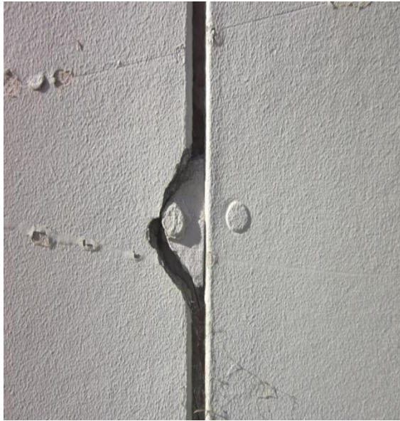
Photo 17: Typical damage to the external wall lining on the western wall of the building
