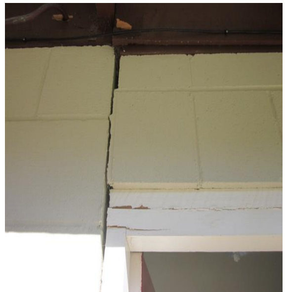
Photo 4: Detail of the separation and damage to the door framing at the northern junction
