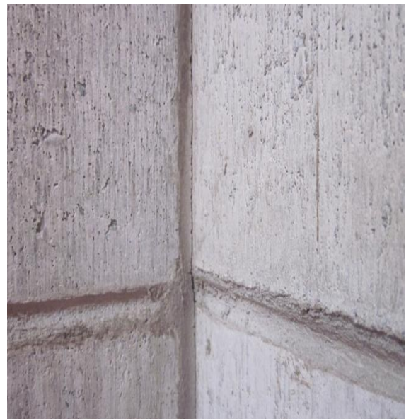
Photo 12: Separation at the west end of the dividing wall
