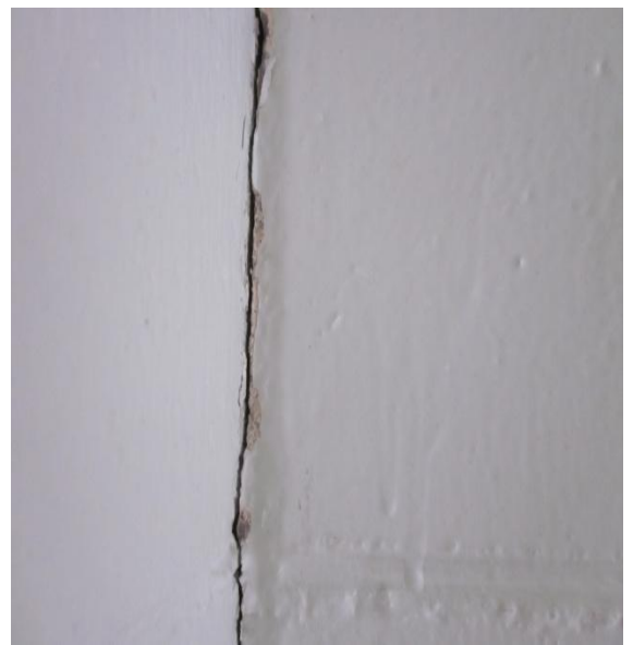
Photo 8: 1.5mm separation at the south end of the north-south wall
