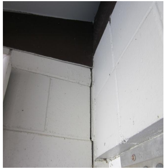
Photo 6: Detail of the separation at the southern junction
