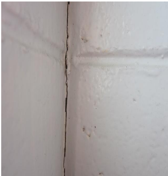
Photo 15: 1mm separation between the 2m high internal walls and the northern walls of the toilet block
