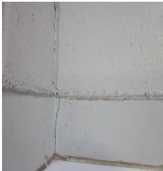
Photo 11: Separation at the east end of the dividing wall
