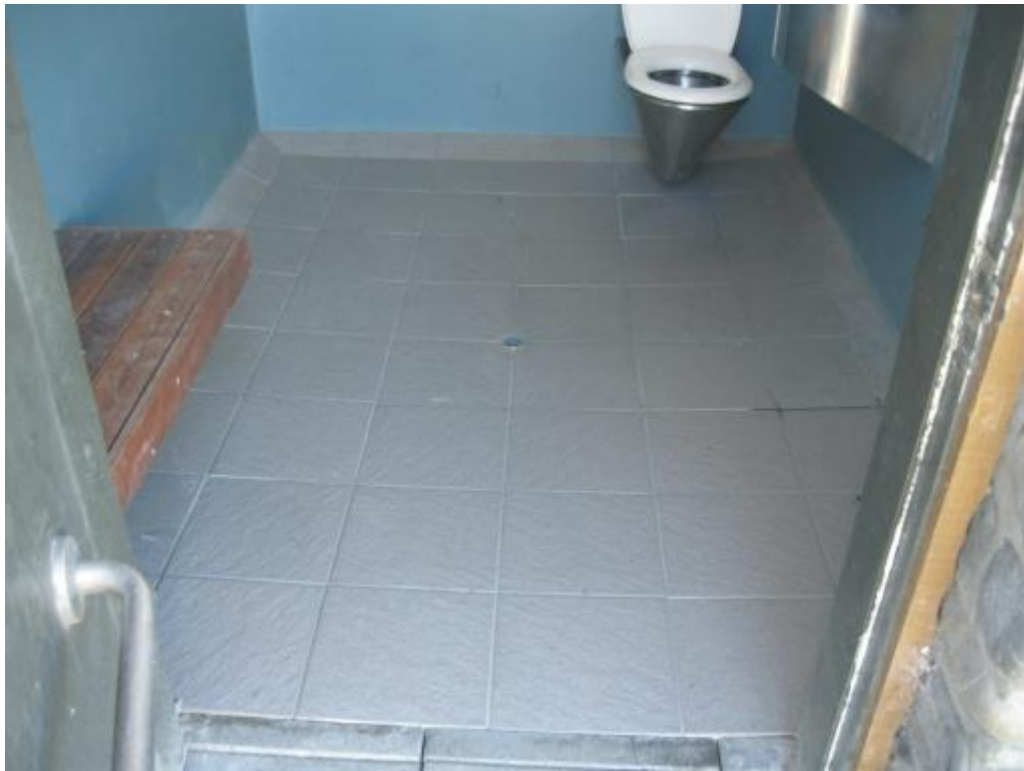
Photograph 5 Tiled concrete floor slab.
