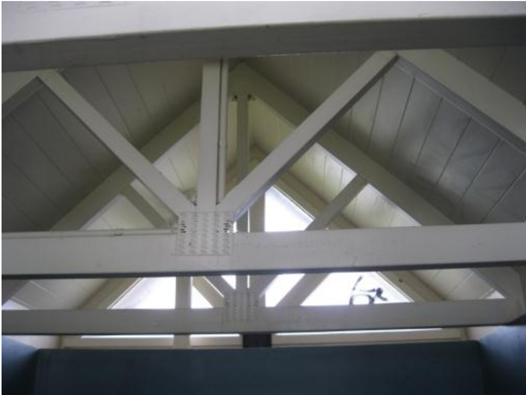
Photograph 3 Timber Truss roof structure
