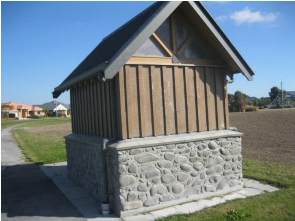
Photograph 2 View of building from the Northeast.
