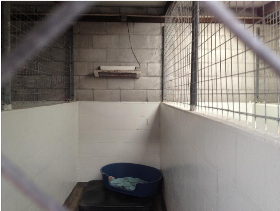
Photo 3: Interior view of typical dog shelter space with transverse half height concrete masonry partitions
