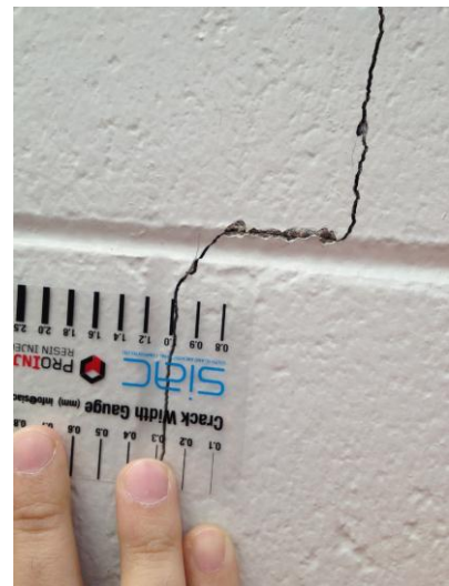
Photo 10A and 10B: Vertical cracking to concrete masonry in the order of 1.0mm at midspan of wall length.
