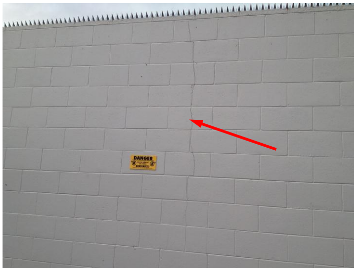
Photo 10A and 10B: Vertical cracking to concrete masonry in the order of 1.0mm at midspan of wall length.
