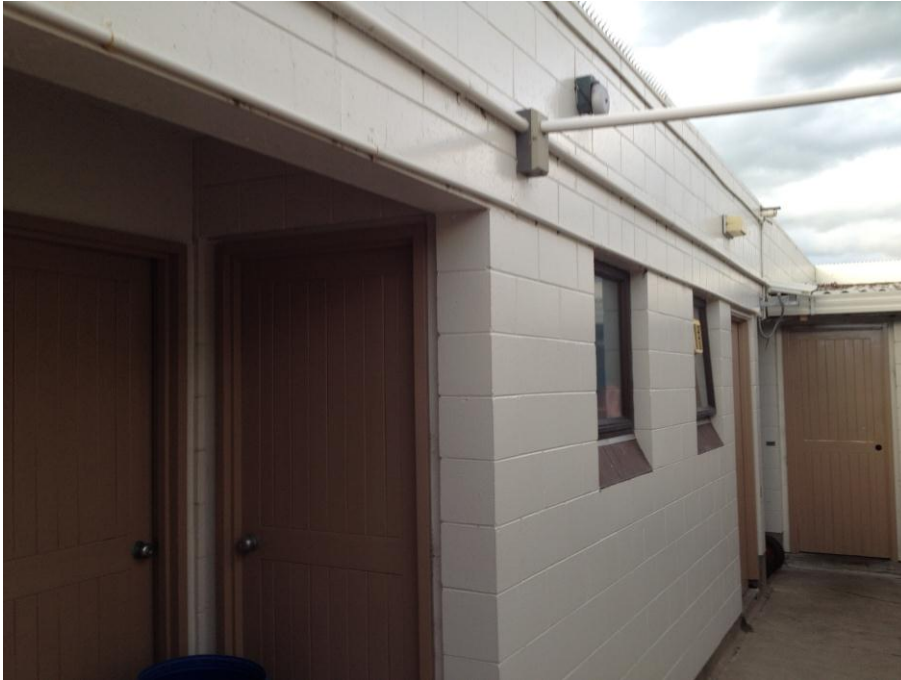
Photo 5: Interior view of headers and lintels in the main corridor.
