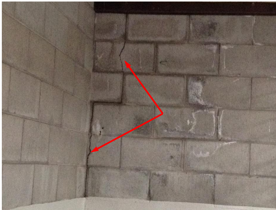
Photo 8: Vertical cracking to concrete masonry wall in the order of 3.5mm at corner where intersecting walls occur
