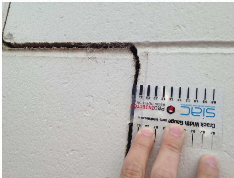
Photo 11A, 11B & 11C: Vertical cracking to concrete masonry wall on the order of 4.0mm at midspan of wall length
