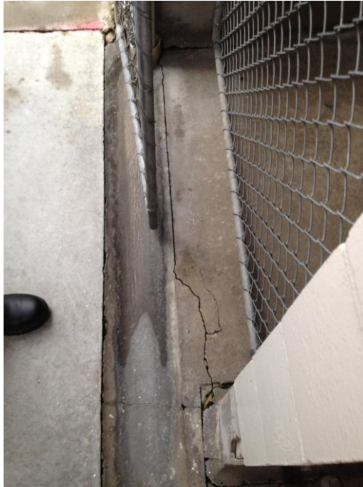
Photo 12: Cracks and separation of floor slab on the order of 1.0mm – 4.0mm at construction joints and at walls.
