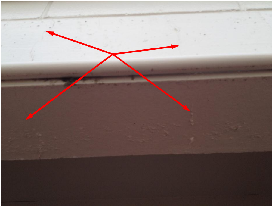
Photo 9: Hairline cracking at concrete masonry lintel.
